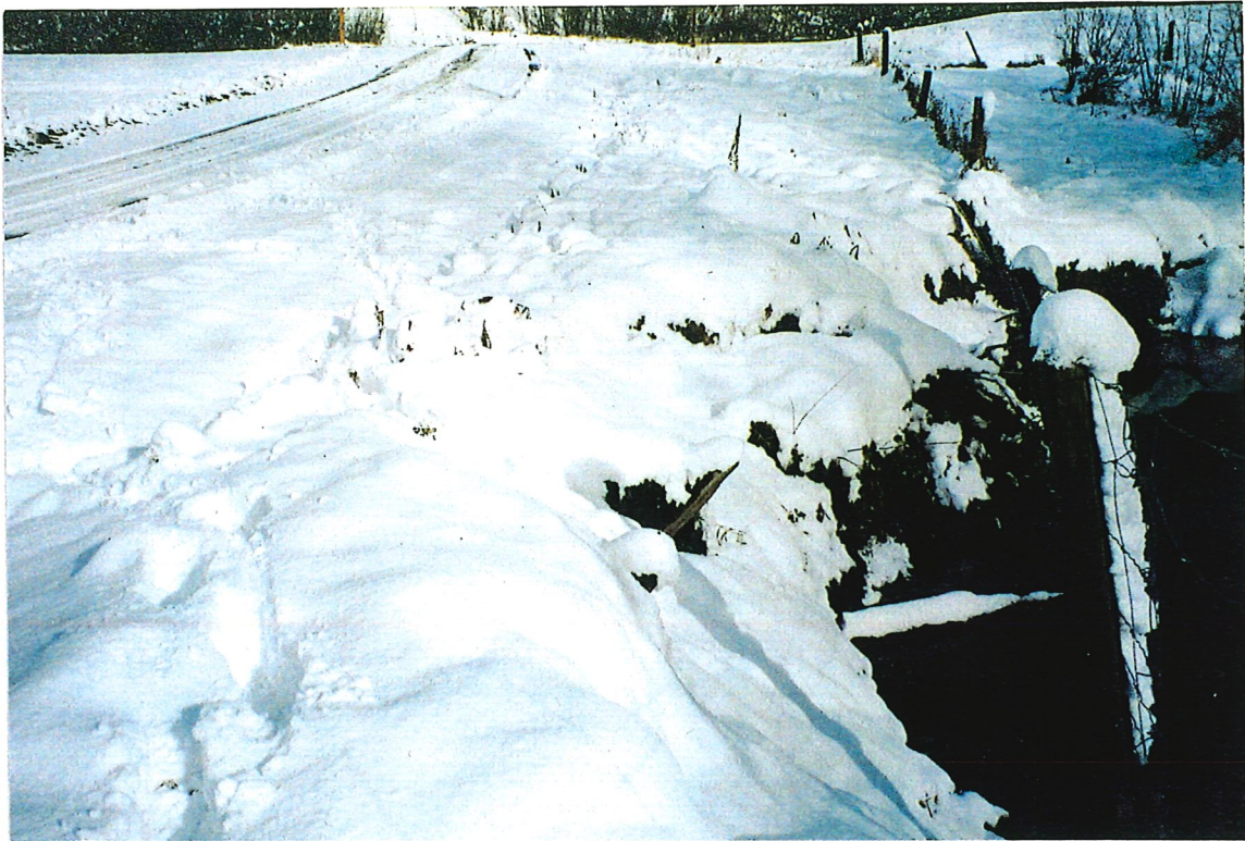
Photo 27 Bank Erosion is Gradually Undermining the Rose Lake Cutoff Roadbank at BR-S10
