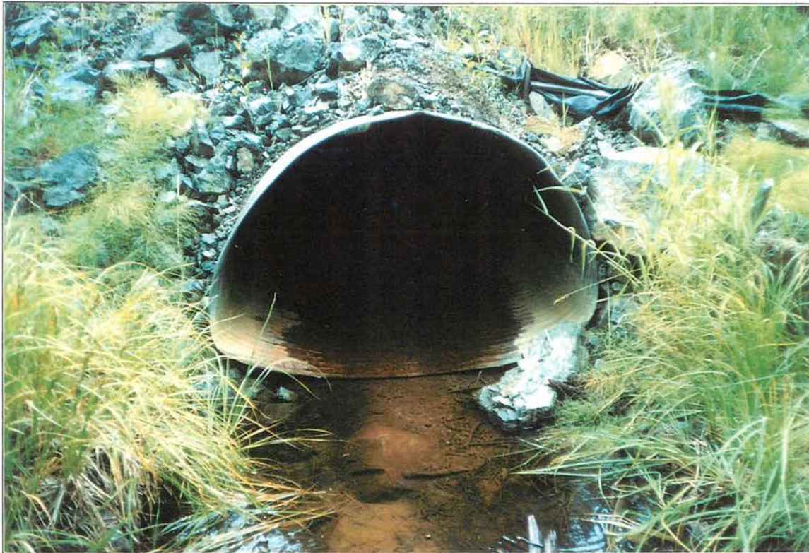
Site #580, Culvert outlet. Roll #58, Frame #20, Date: 2002/09/13
