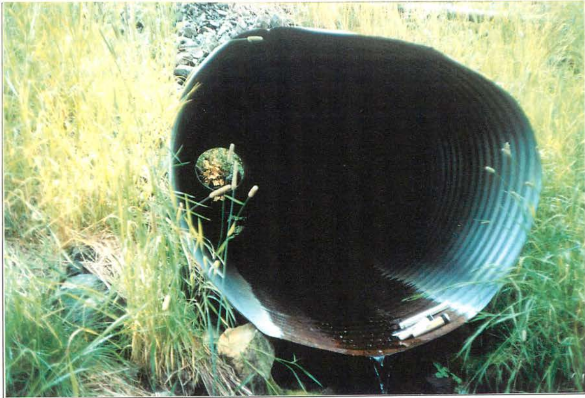
Site #578, Culvert outlet (note meters, tape and thermometer). Roll #58, Frame #16, Date: 2002/09/13
