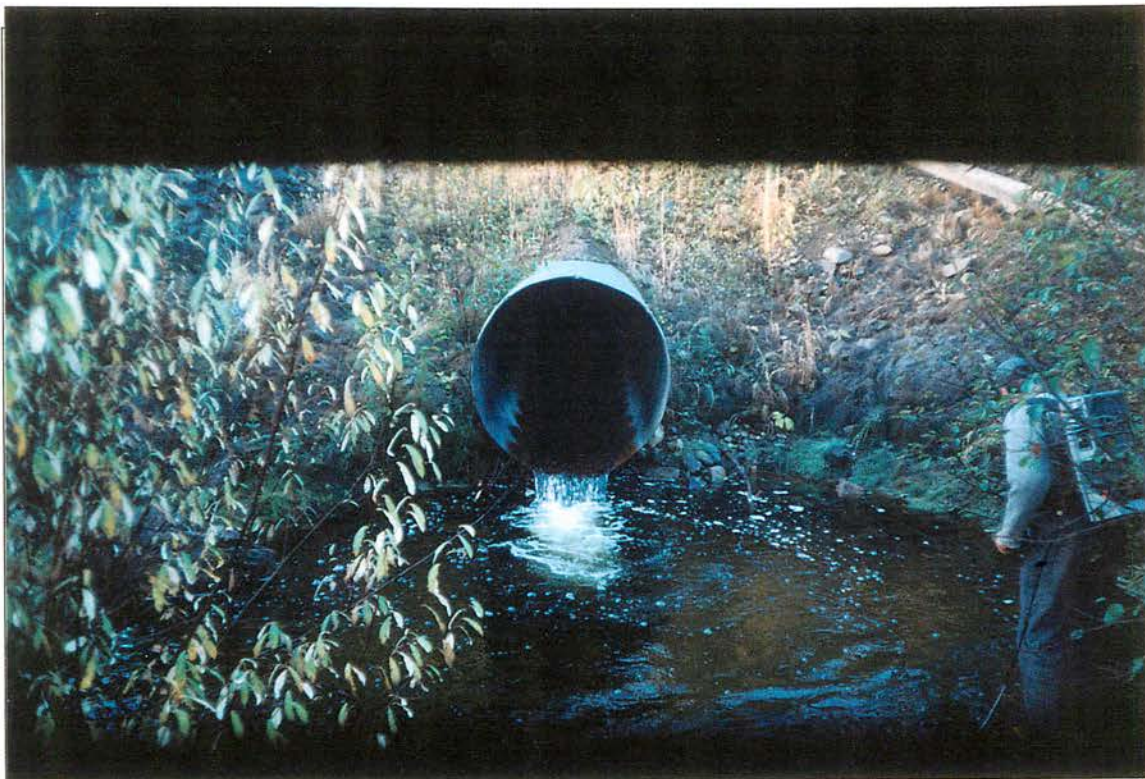
Site #363, Upstream photo of 1.6 m cv, perched 25 cm. Roll #80, Frame #03, Date: 2002/10/07
