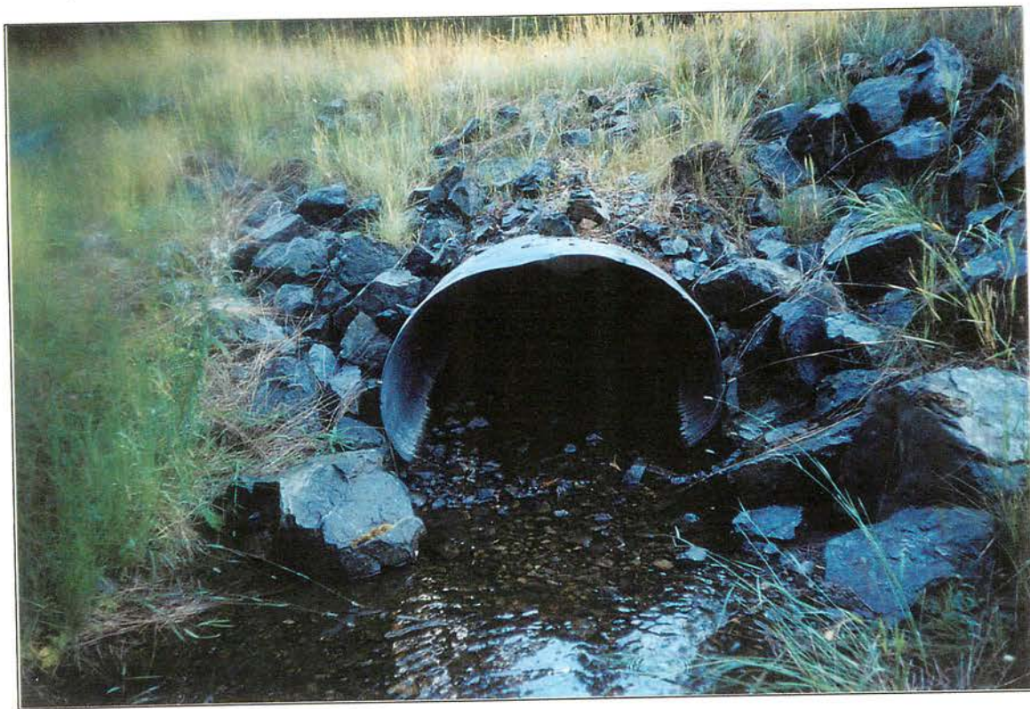
Site #74, Upstream photo of culvert. Roll #9, Frame #13A, Date: 2002/09/29
