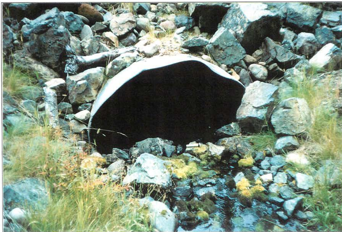
Site #578, Downstream culvert on lower road, good crossing structure downstream of road crossing. Roll #58, Frame #19, Date: 2002/09/13
