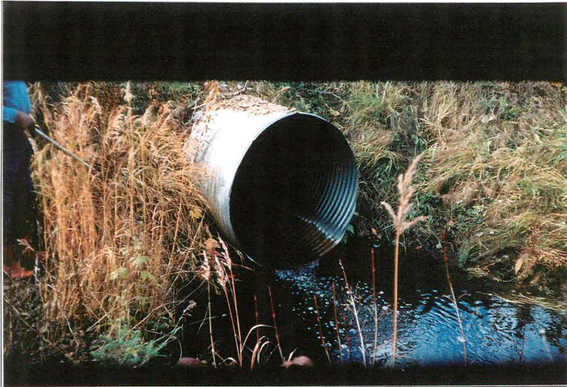
Site #373, Upstream photo of culvert, partial barrier at low flows. Roll #80, Frame #18, Date: 2002/10/08
