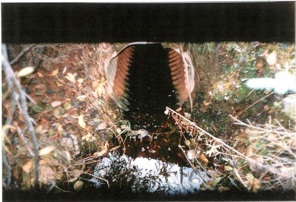
Site #374, Upstream photo of 0.6 m culvert, passable under all flows. Roll #80, Frame #23, Date: 2002/10/08
