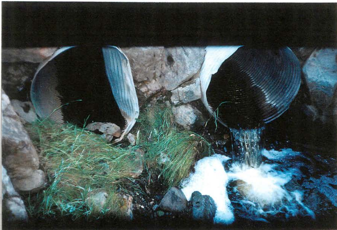
Site #372, Upstream view of 1.4 m twim cv's, perched 0.5 m. Roll #80, Frame #14, Date: 2002/10/08
