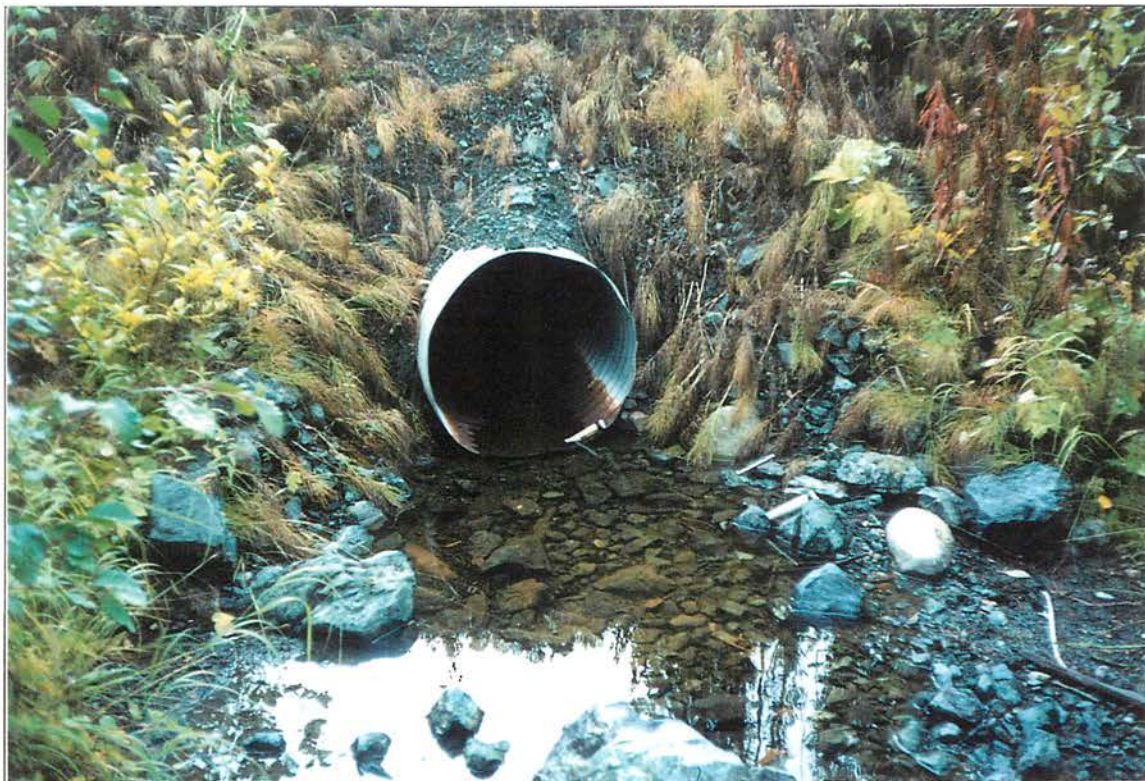
Site #576, Culvert outlet (not pH and conductivity meters with thermometer). Roll #58, Frame #11, Date: 2002/09/13
