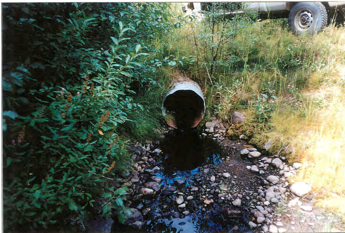
Site #38, Photo of culvert partial barrier. Roll #4, Frame #22A, Date: 2002/08/30
