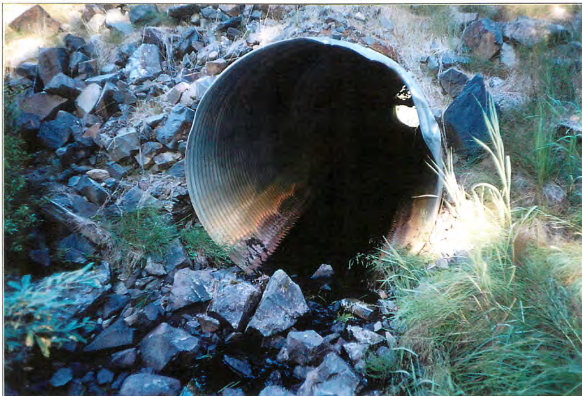
Site #35, Photo of well placed culvert. Roll #4, Frame #13A, Date: 2002/08/30
