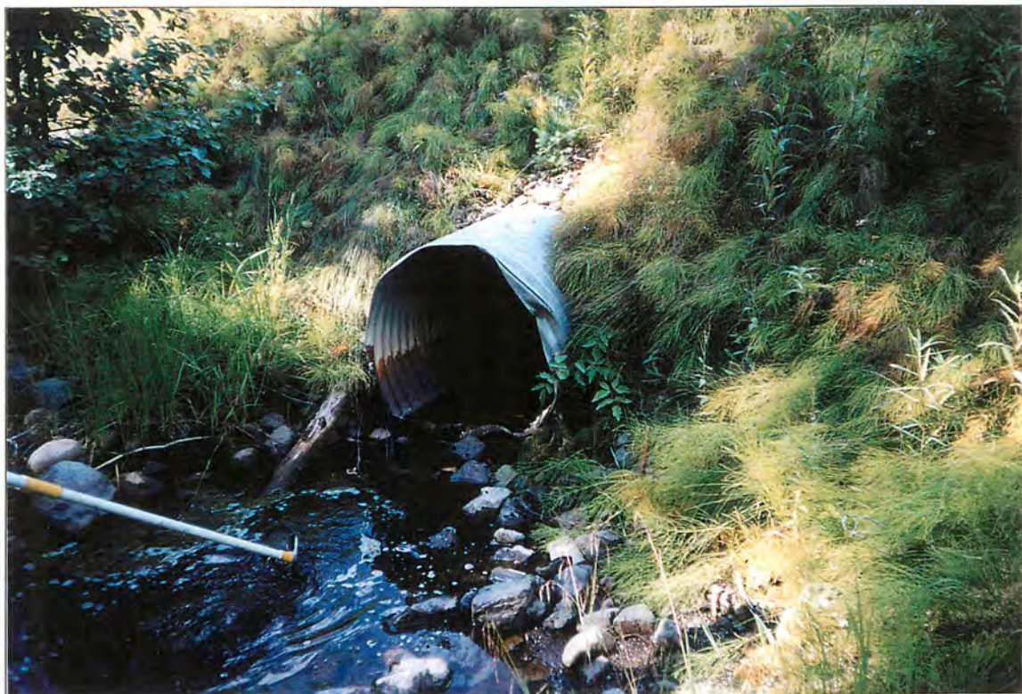
Site #31, Photo of culvert - partial barrier. Roll #4, Frame #1A, Date: 2002/08/29
