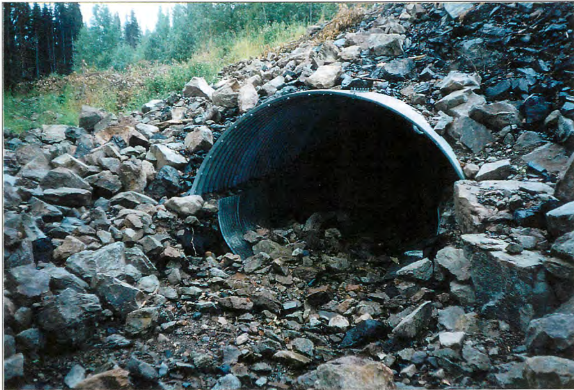
Site #11, Upstream photo of arch culvert. Roll #1, Frame #20A, Date: 2002/08/28
