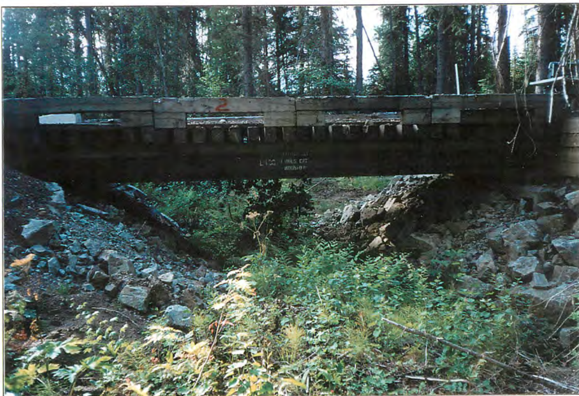
Site #2, Upstream photo of bridge crossing. Roll #1, Frame #3A, Date: 2002/08/27
