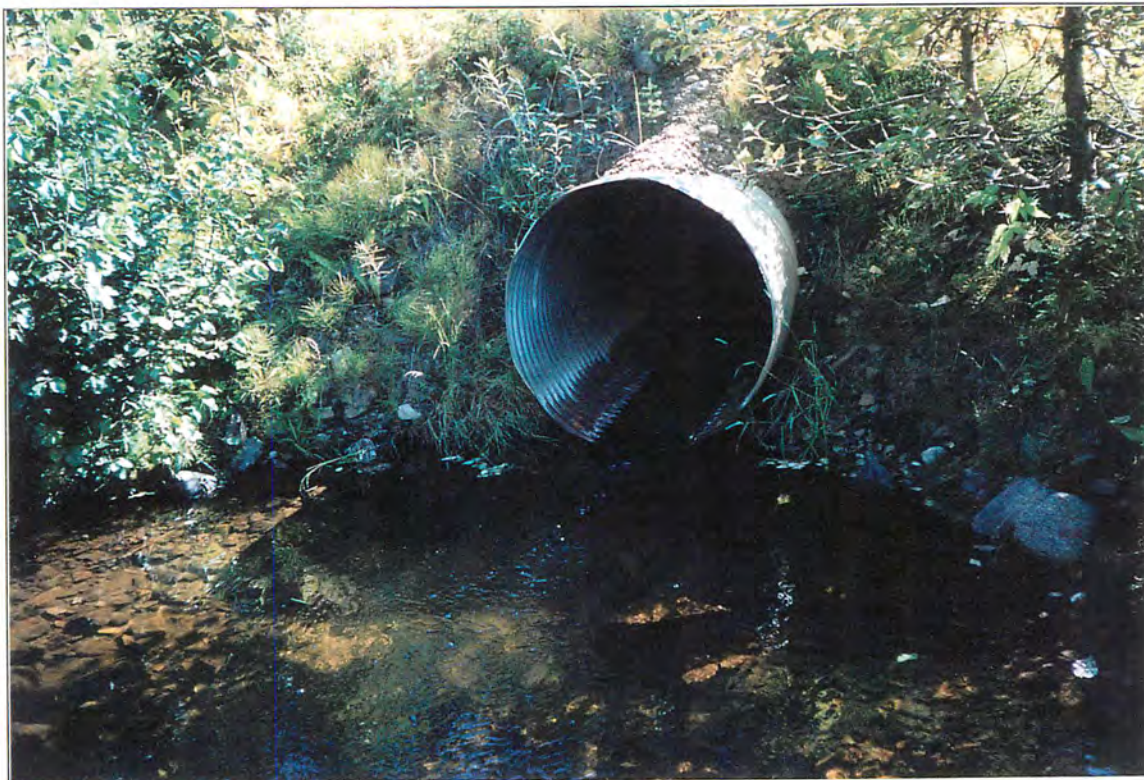
Site #36, Photo of culvert - possible velocity barrier. Roll #4, Frame #16A, Date: 2002/08/30
