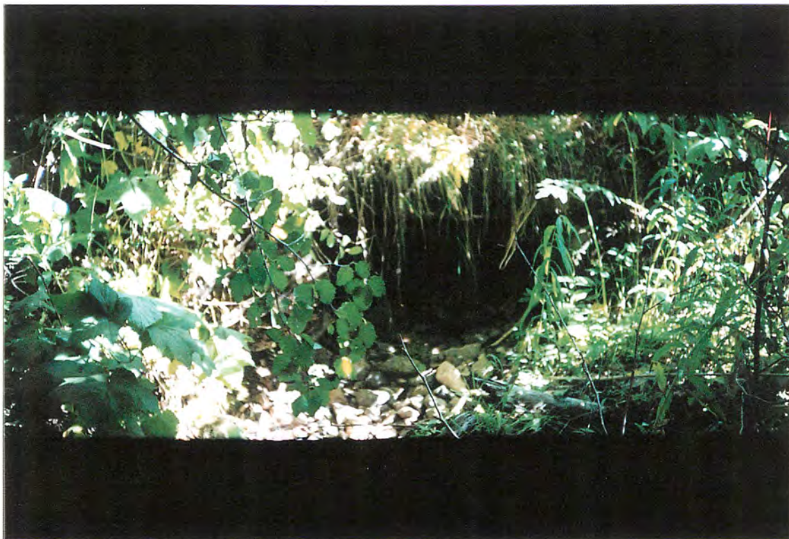
Site #26, Wooden box culvert. Roll #3, Frame #08, Date: 2002/08/29
