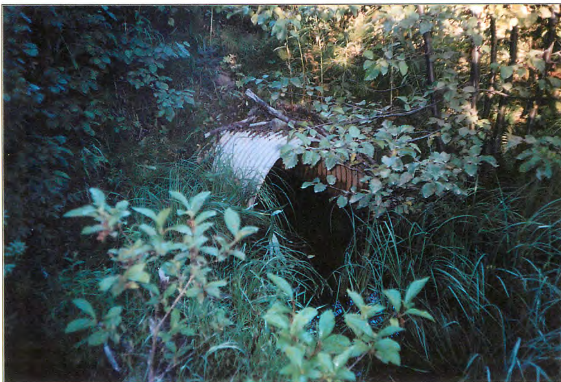
Site #32, Photo of well placed culvert. Roll #4, Frame #5A, Date: 2002/08/30
