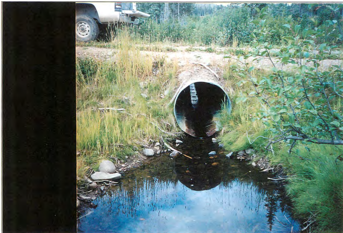
Site #39, Photo of culvert. Roll #4, Frame #25A, Date: 2002/08/30
