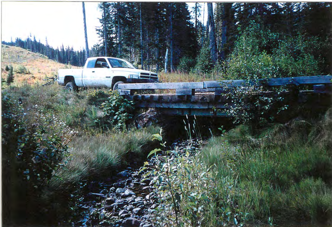
Site #37, Bridge crossing. Roll #4, Frame #19A, Date: 2002/08/30
