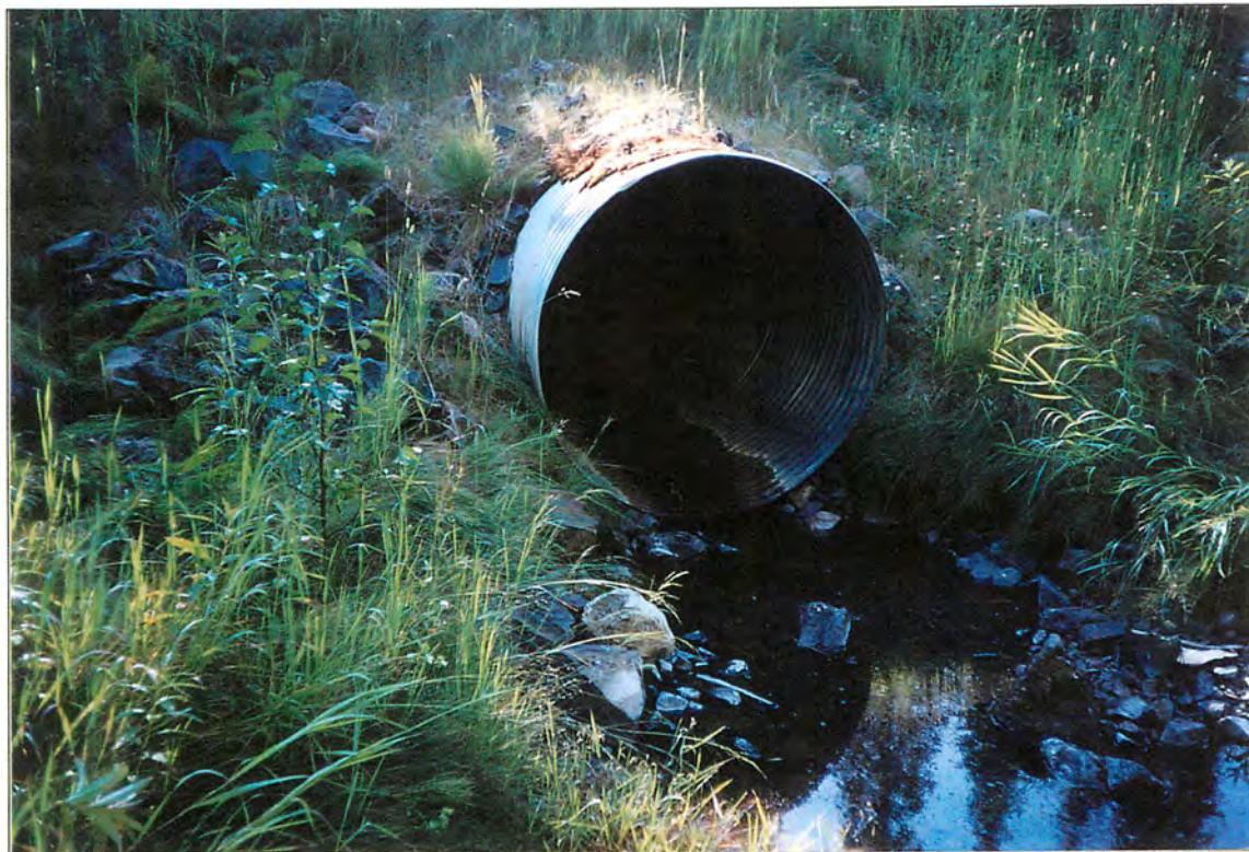
Site #34, Photo of culvert - partial barrier. Roll #4, Frame #10A, Date: 2002/08/30
