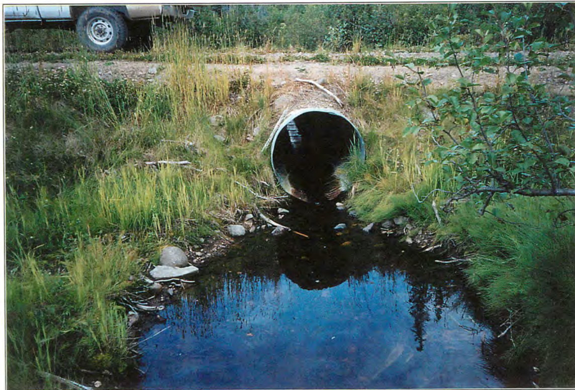
Site #39, Photo of culvert. Roll #5, Frame #01, Date: 2002/08/30
