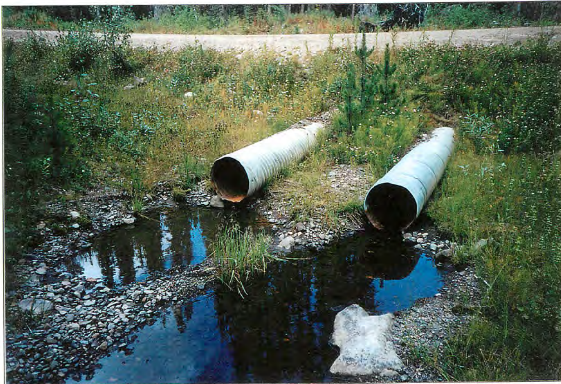
Site #30, Upstream photo of twin culverts. Roll #3, Frame #20, Date: 2002/08/29
