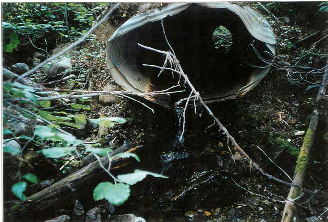
Site #20, Upstream photo of culvert crossing. Roll #2, Frame #17A, Date: 2002/08/28
