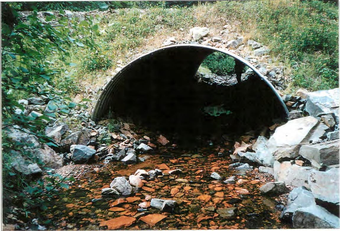
Site #19, Arch culver in Reach 1. Roll #2, Frame #13A, Date: 2002/08/28
