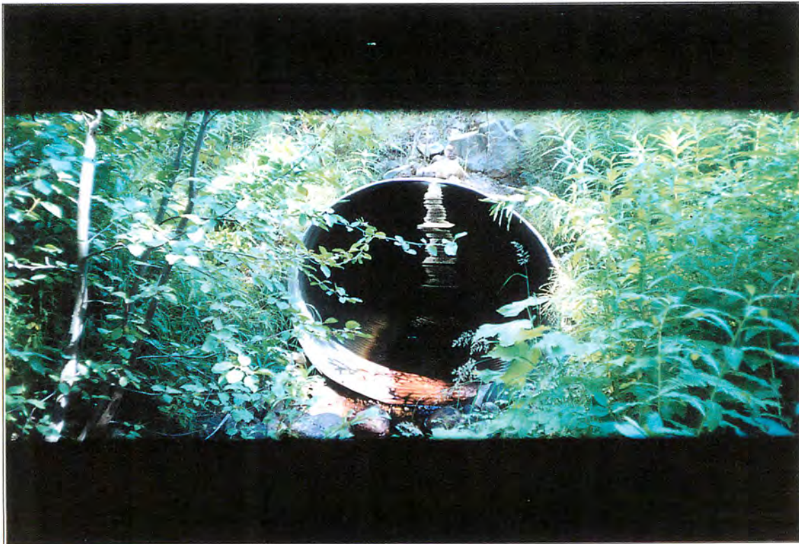
Site #29, Photo of well placed culvert. Roll #3, Frame #17, Date: 2002/08/29
