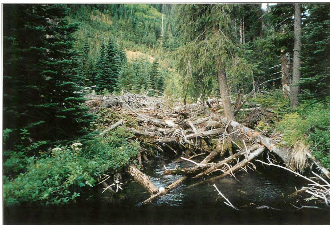
Site #986, Upstream photo of log jam from multiple slides. Roll #95, Frame #14, Date: 2002/09/07
