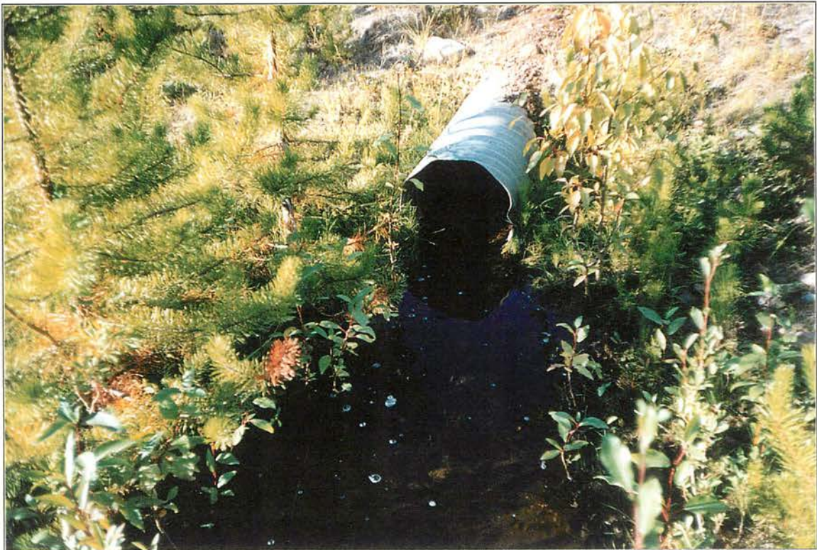
Site #527, 0.5 m culvert outlet. Roll #53, Frame #19, Date: 2002/09/05
