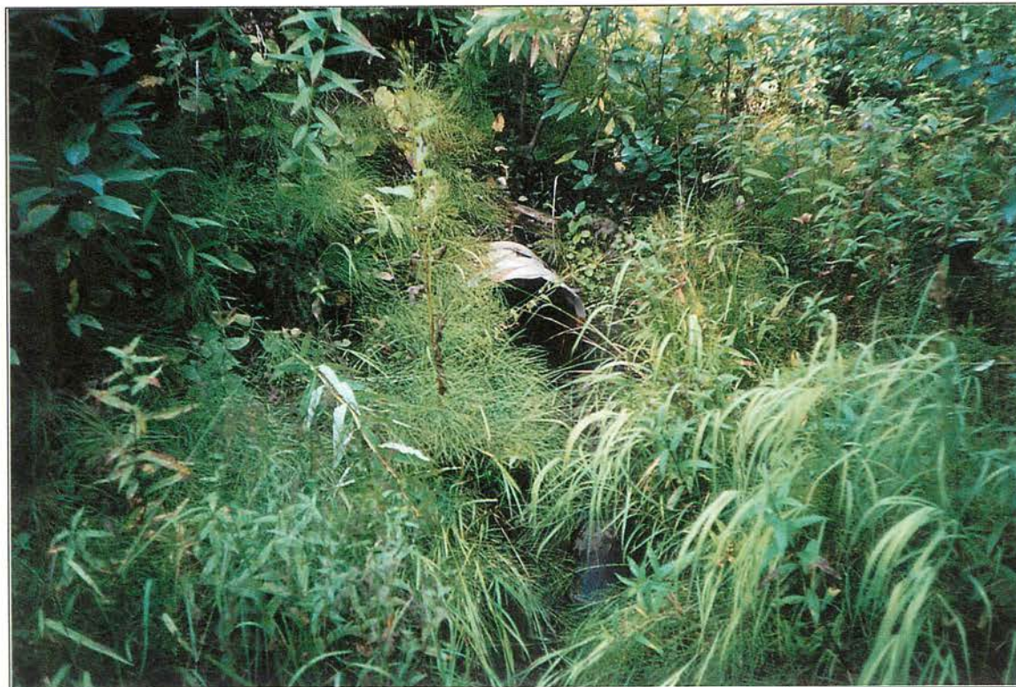
Site #522, Culvert providing adequate drainage. Roll #52, Frame #16, Date: 2002/09/05
