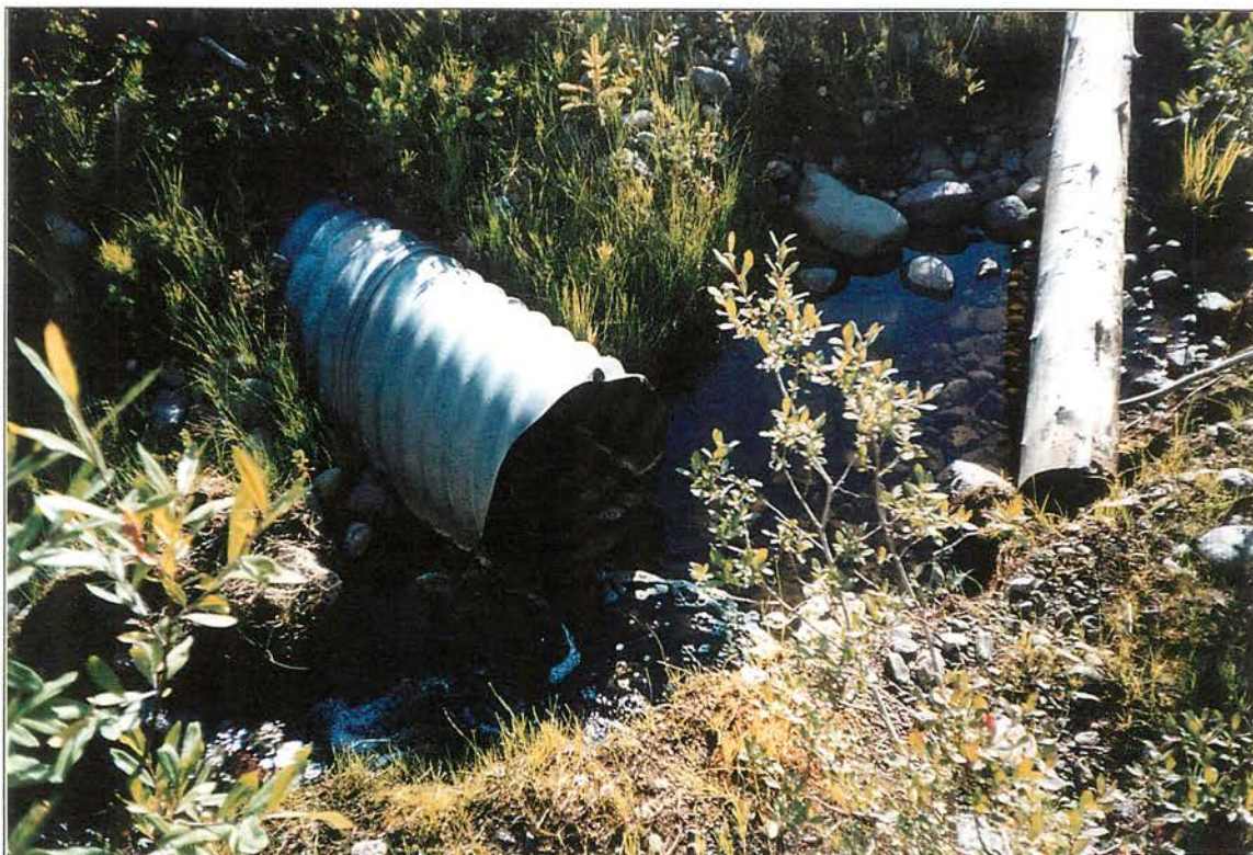
Site #527, Diversion through .5 m culvert (inlet). Roll #53, Frame #16, Date: 2002/09/05
