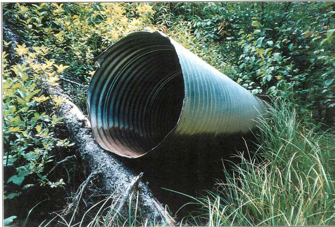
Site #521, Extension at upstream end of culvert slightly perched. Roll #52, Frame #14, Date: 2002/09/05
