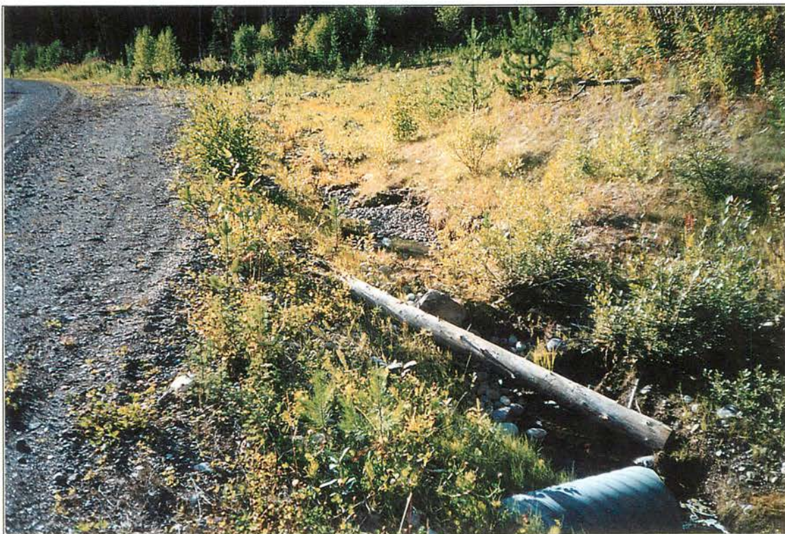
Site #527, 0.5 m culvert in foreground and overflow down ditchline in background. Roll #53, Frame #17, Date: 2002/09/05
