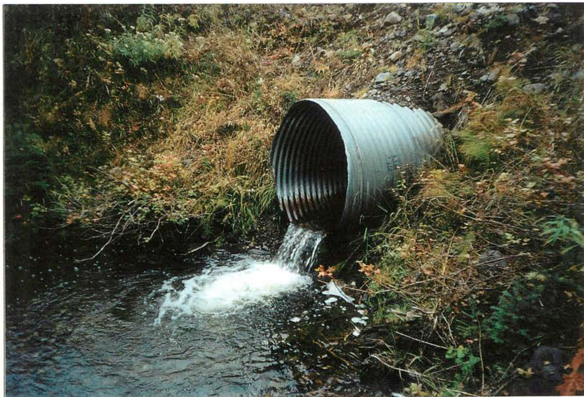
Site #456, Culvert outlet. Roll #66, Frame #06, Date: 2002/10/01
