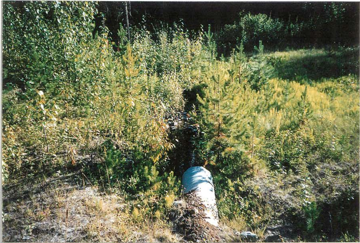
Site #527, 0.5 m culvert outlet and stream flowing into forested area. Roll #53, Frame #18, Date: 2002/09/05
