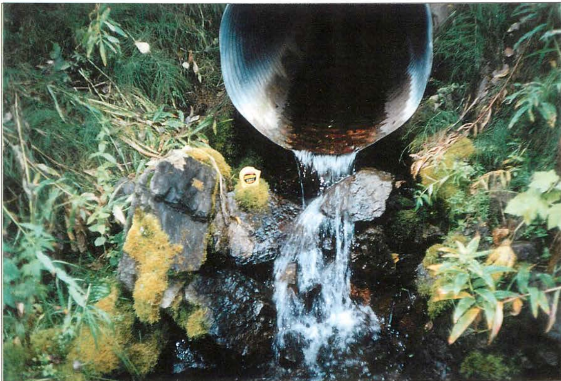
Site #505, Culvert outlet. Roll #50, Frame #15, Date: 2002/09/03
