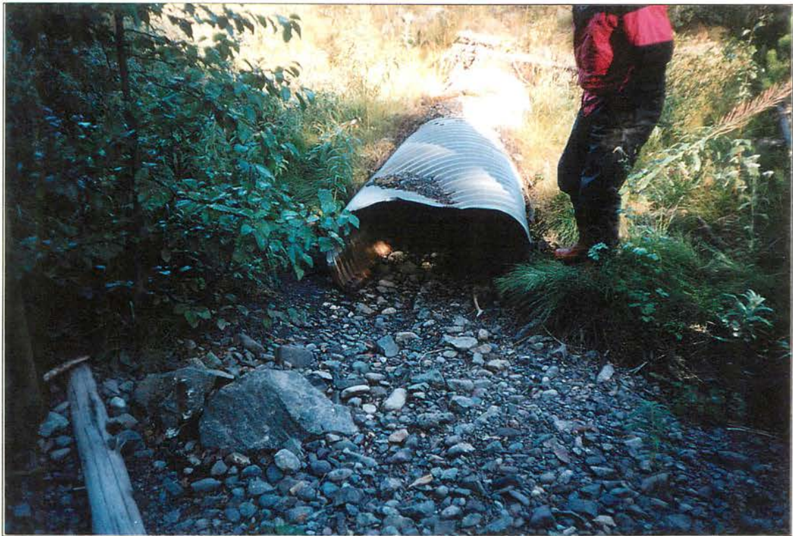
Site #529, Culvert outlet. Roll #54, Frame #01, Date: 2002/09/06
