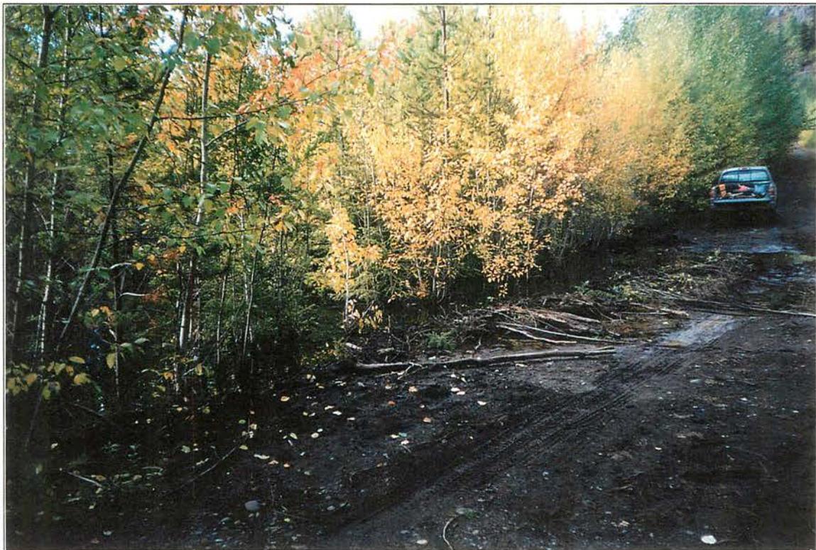
Site #558, Beaver dam at road - flooded. Roll #57, Frame #13, Date: 2002/09/10
