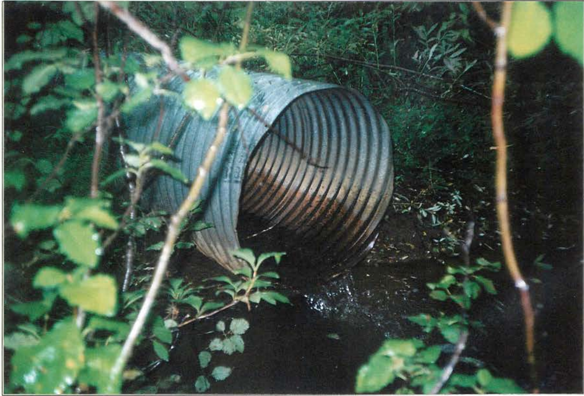
Site #509, Culvert outlet / extension. Roll #51, Frame #03, Date: 2002/09/04
