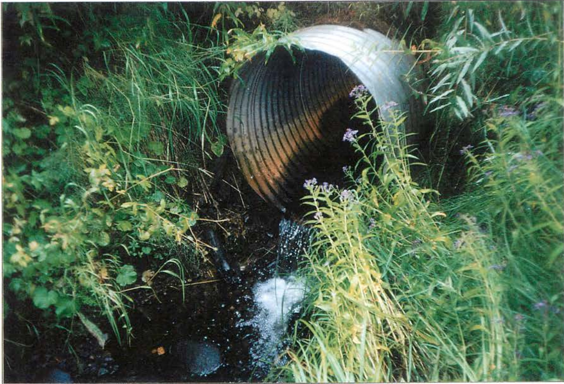
Site #511, Culvert outlet. Roll #51, Frame #04, Date: 2002/09/04
