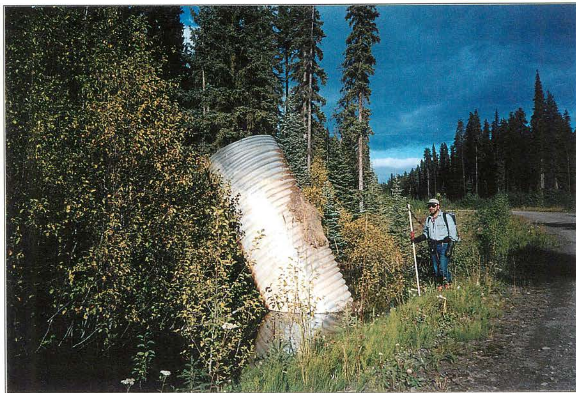
Site #527, Culvert inlet and ponded section. Roll #53, Frame #07, Date: 2002/09/05
