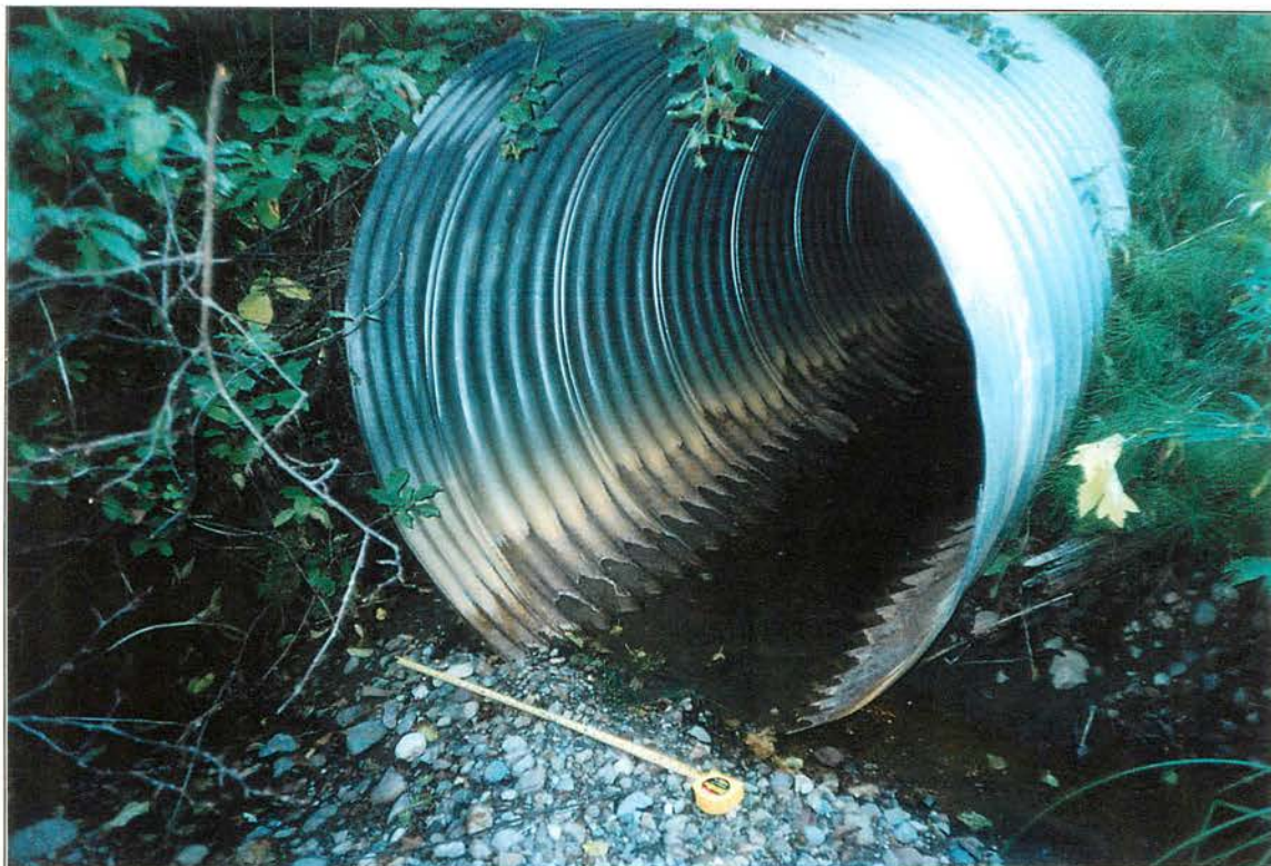
Site #527, Dewatered culvert due to upstream disturbance. Roll #53, Frame #04, Date: 2002/09/05
