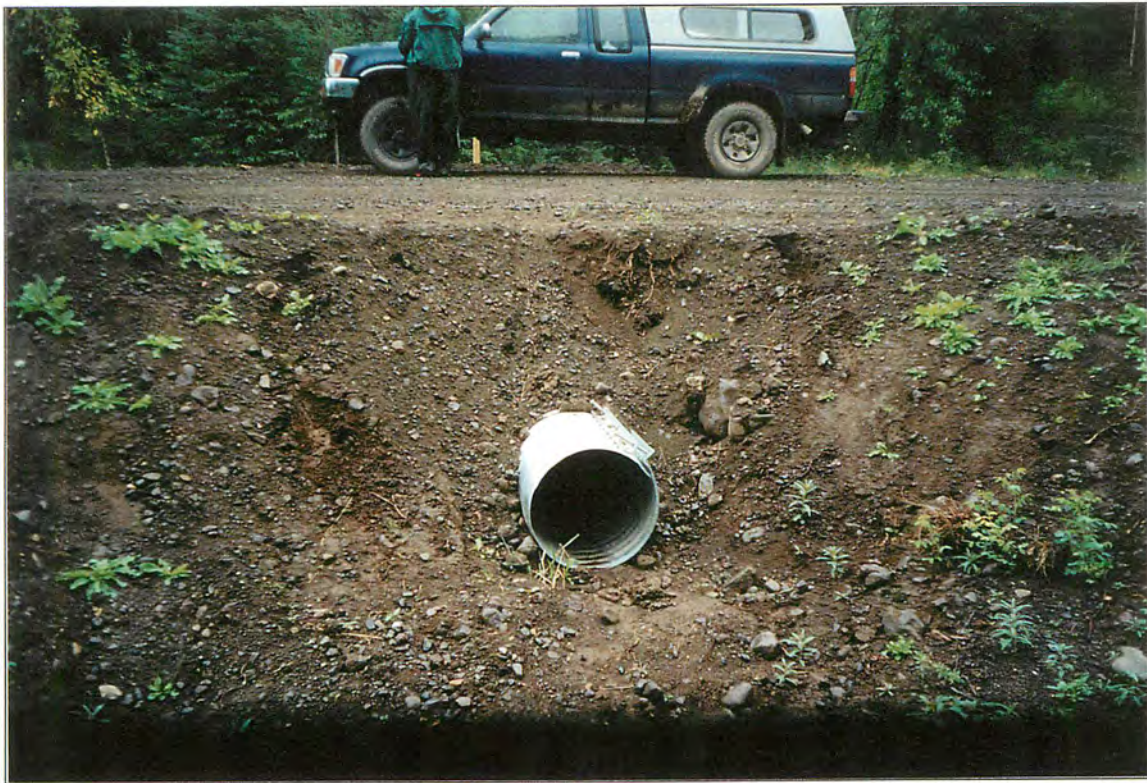
Site #254, Upstream photo of newly installed culvert. Roll #99, Frame #12, Date: 2002/09/03
