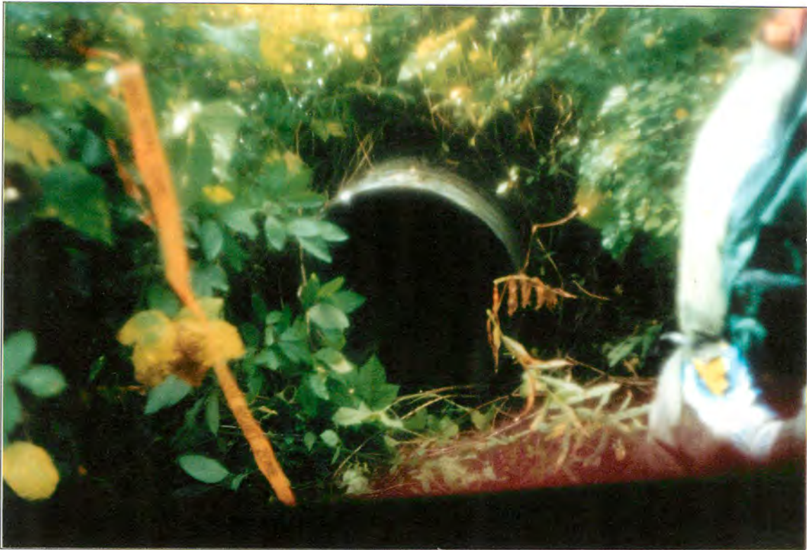
Site #261, Upstream photo of passable 0.8 x 10 m culvert. Roll #98, Frame #07, Date: 2002/09/03
