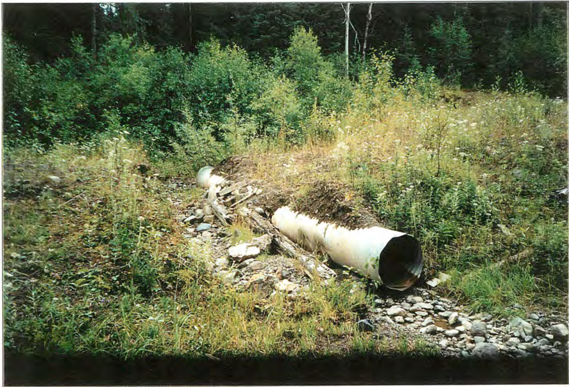
Site #283, Upstream photo of culvert (50 cm by 8 m) Roll #95, Frame #03, Date: 2002/09/06
