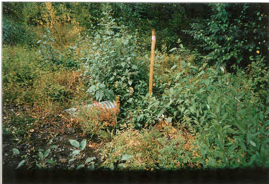
Site #258, Photo of culvert. Roll #99, Frame #24, Date: 2002/09/03
