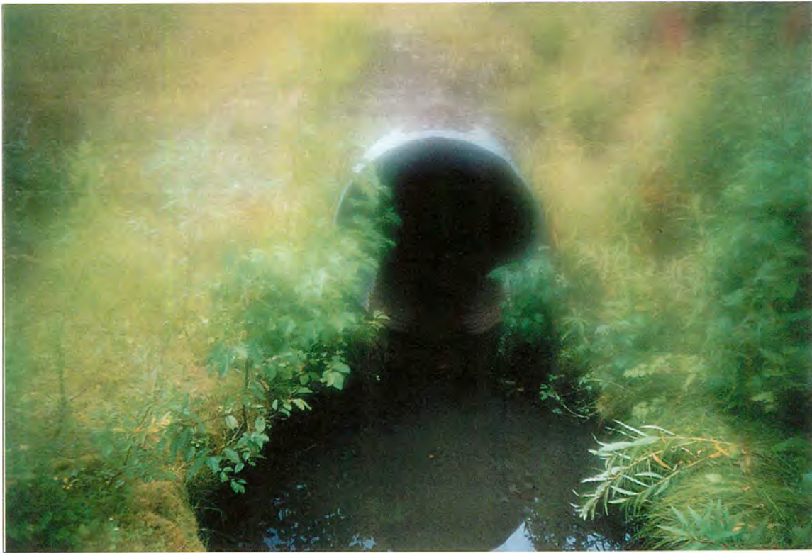
Site #50, Photo of culvert. Roll #6, Frame #07A, Date: 2002/09/03
