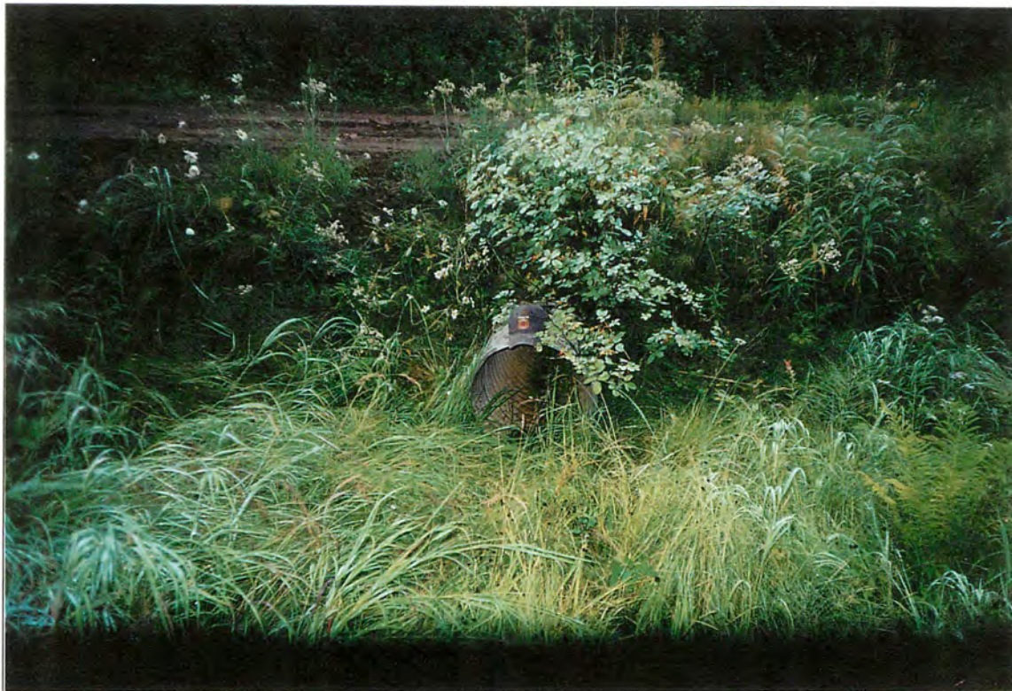
Site #262, Upstream photo of dry culvert outlet. Roll #98, Frame #12, Date: 2002/09/04
