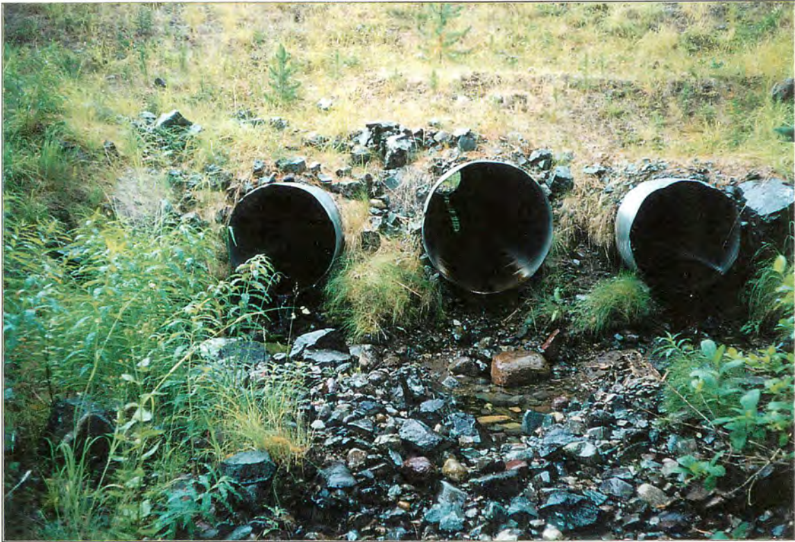
Site #49, Photo of 3 culverts at crossing. Roll #6, Frame #04A, Date: 2002/09/03
