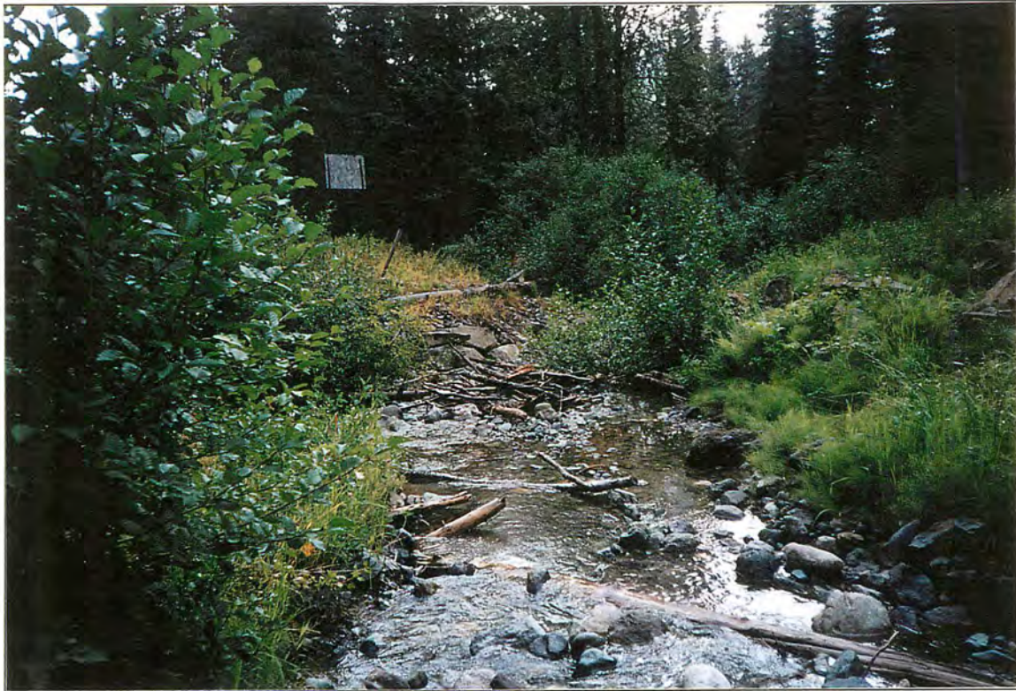
Site #44, Downstream photo of de-activated road crossing. Roll #5, Frame #13, Date: 2002/09/03
