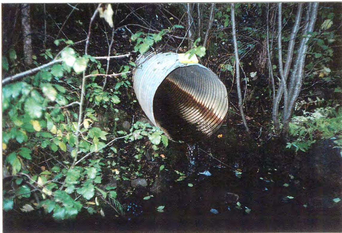
Site #273, Upstream photo of 0.25 m perched CV (partial barrier). Roll #97, Frame #15, Date: 2002/09/05
