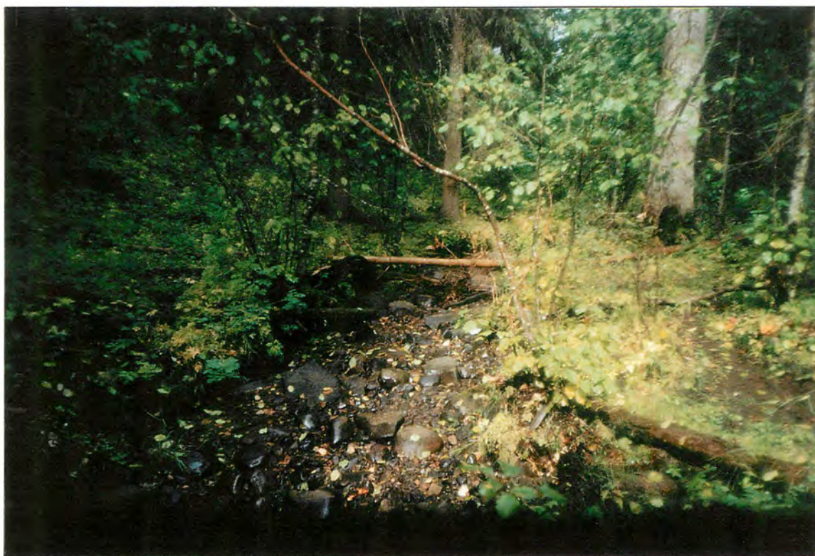
Site #259, Downstream photo of dry channel. Roll #98, Frame #03, Date: 2002/09/03
