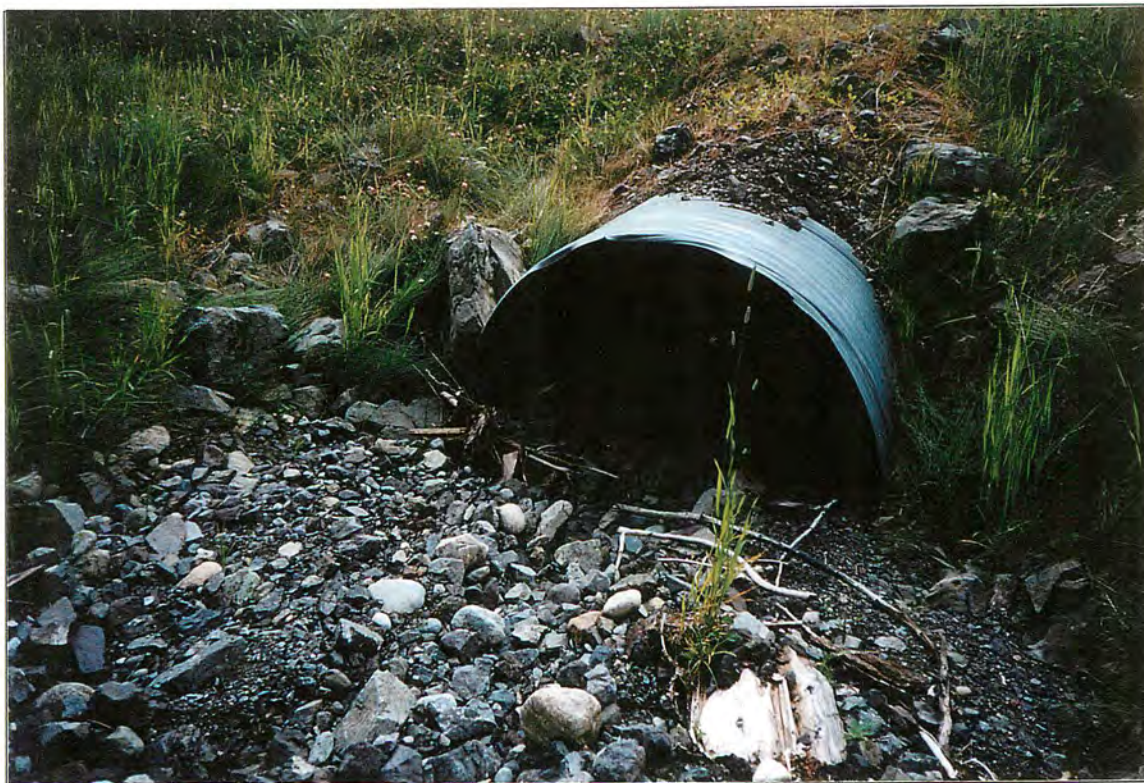
Site #45, Naturally embedded culvert (1700 mm). Roll #5, Frame #17, Date: 2002/09/03
