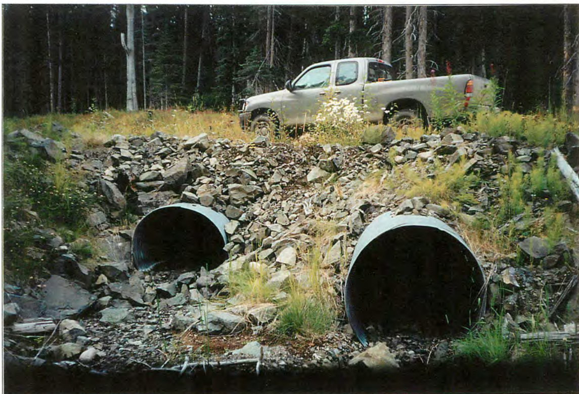
Site #309, Upstream photo of good passable culverts. Roll #92, Frame #13, Date: 2002/09/11
