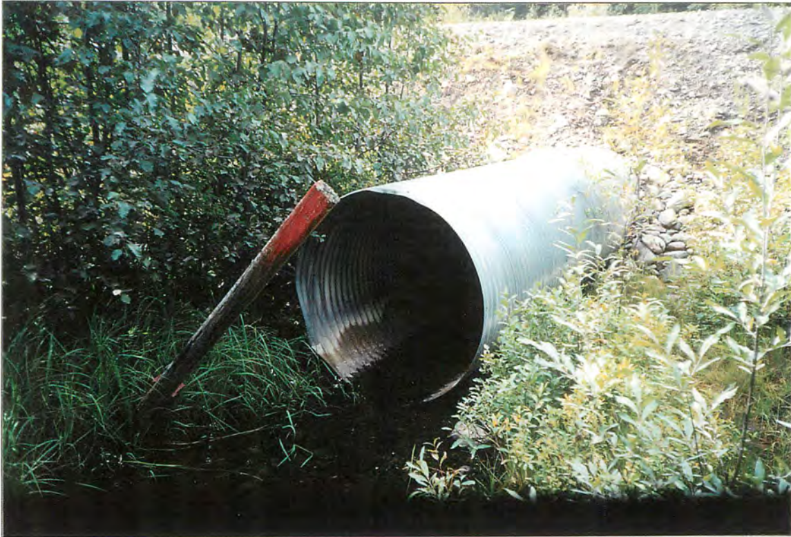
Site #301, Upstream view of culvert. Roll #93, Frame #19, Date: 2002/09/11
