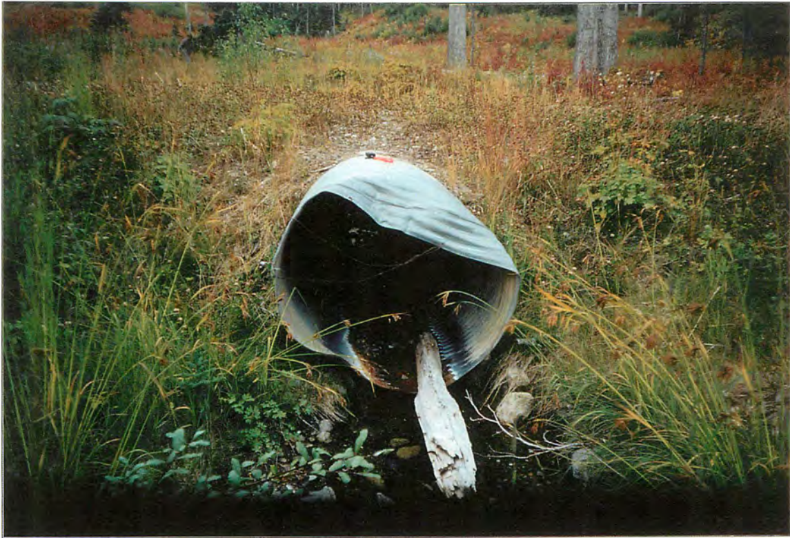
Site #310, Upstream photo of 1.2 x 10 m culvert. Roll #92, Frame #16, Date: 2002/09/11
