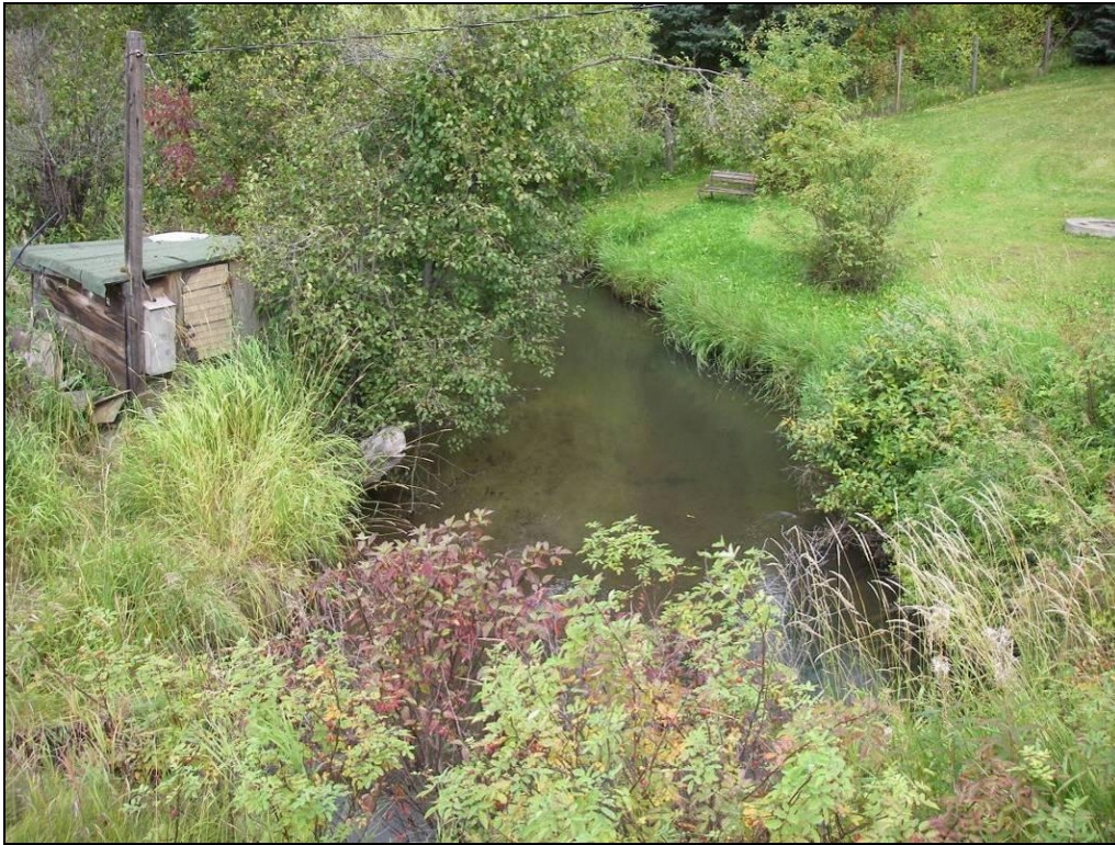
Figure 8. View upstream from the Highway 16 culvert (September 24, 2011).
