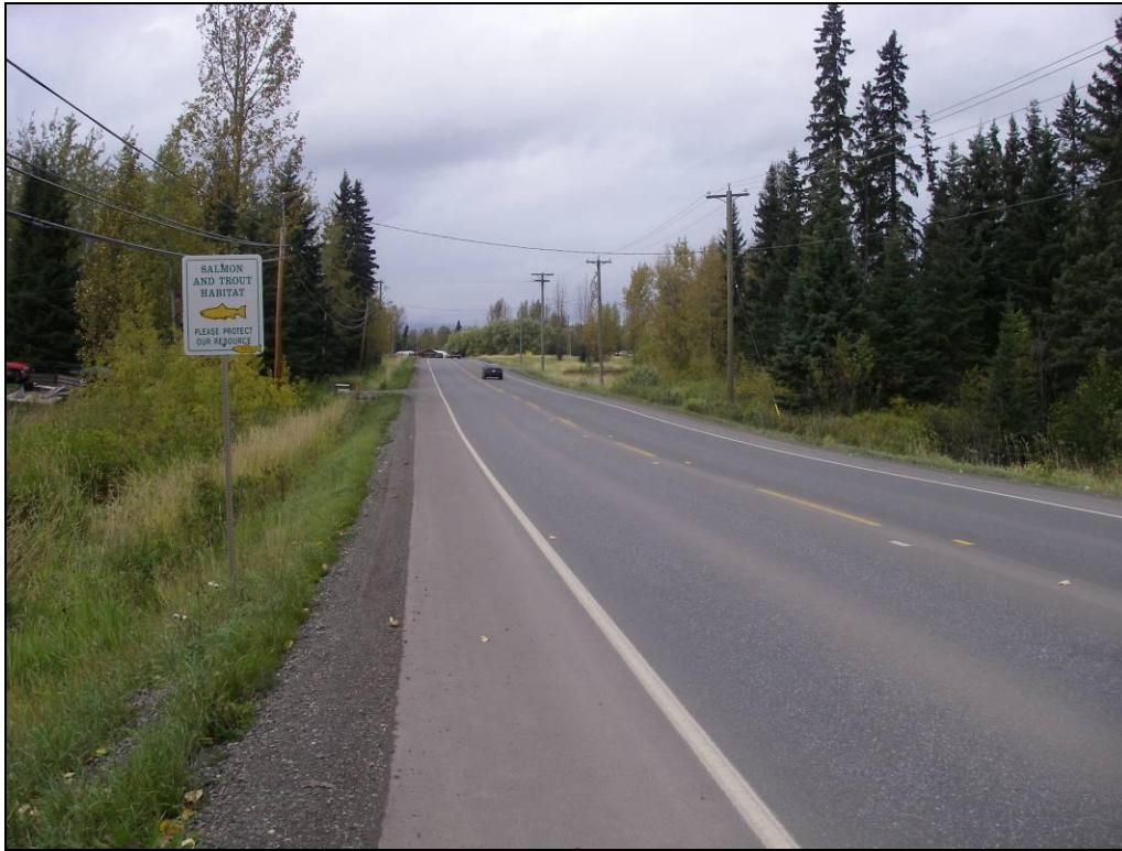
Figure 14. Westbound view, crossing near sign September 24, 2011.
