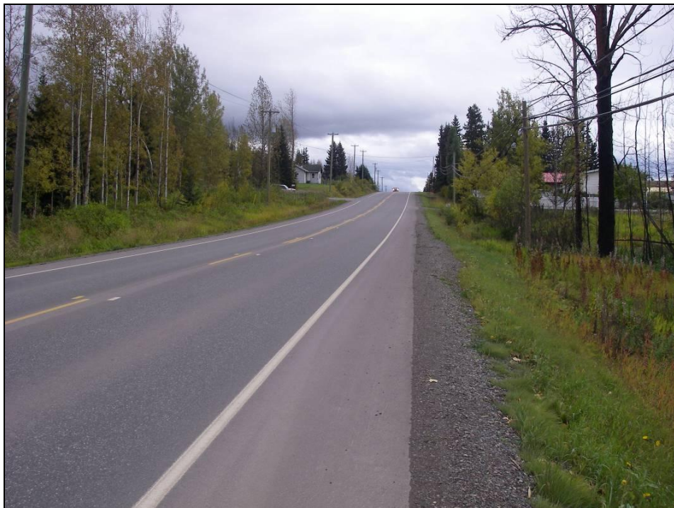
Figure 16. Eastbound view September 24, 2011.
