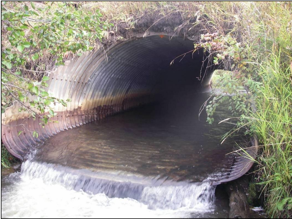
Figure 3. View upstream to outlet, 3500 mm wide by 2200 mm high elliptical culvert, 20 cm outlet drop (September 24, 2011).
