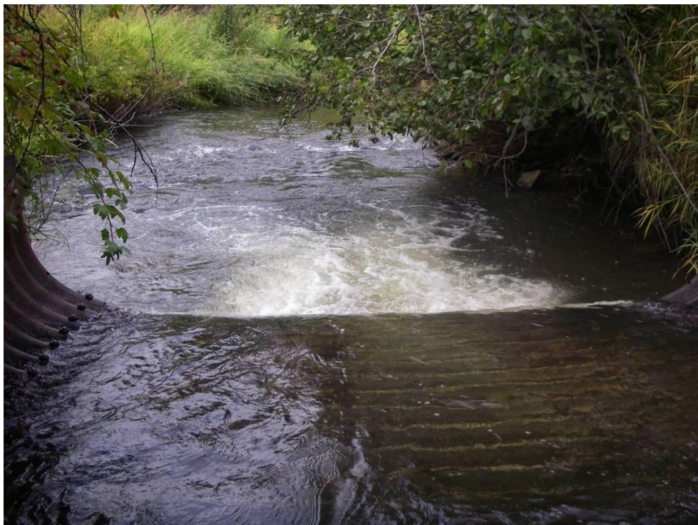
Figure 4. View downstream showing outlet pool and short riffle section (September 24, 2011).
