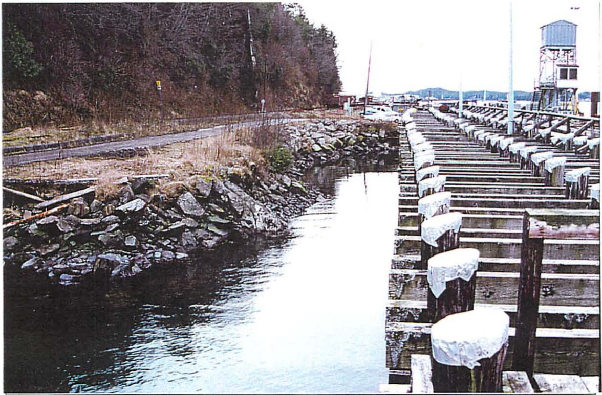
Photo #8: Looking south at the back of the mooring wall.
