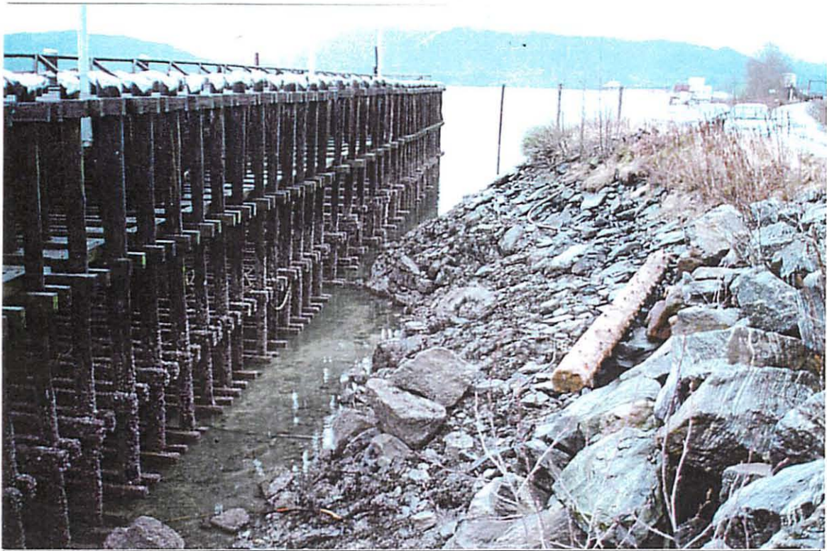
Photo #5: Looking north along the back of the mooring wall.
