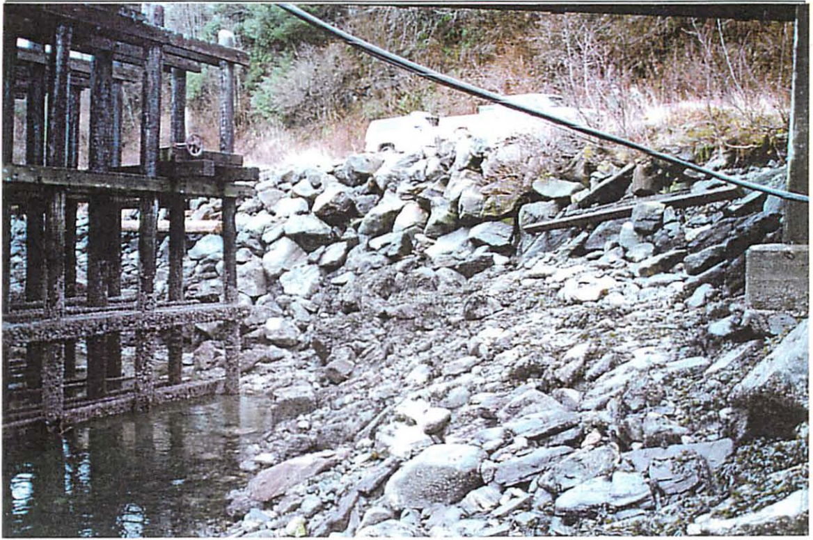
Photo #3: Looking at the south end of the mooring wall.
