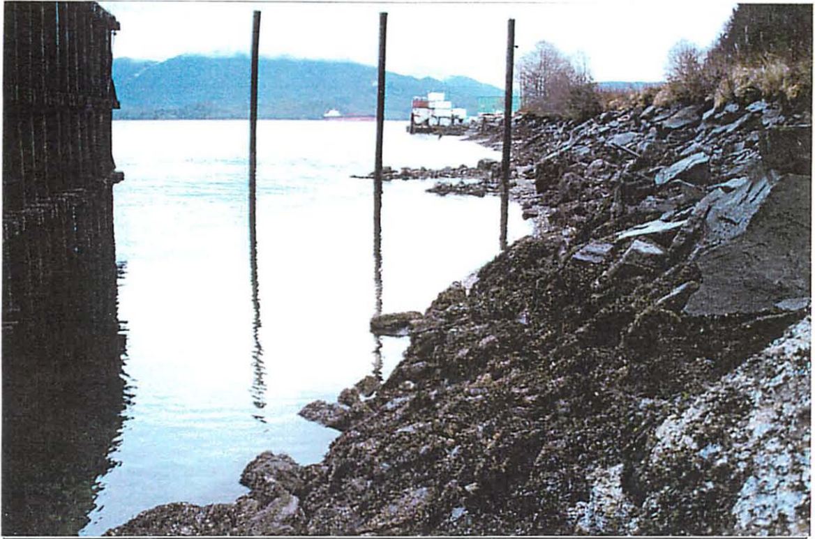
Photo #7: Looking north near the north end of the mooring wall.
