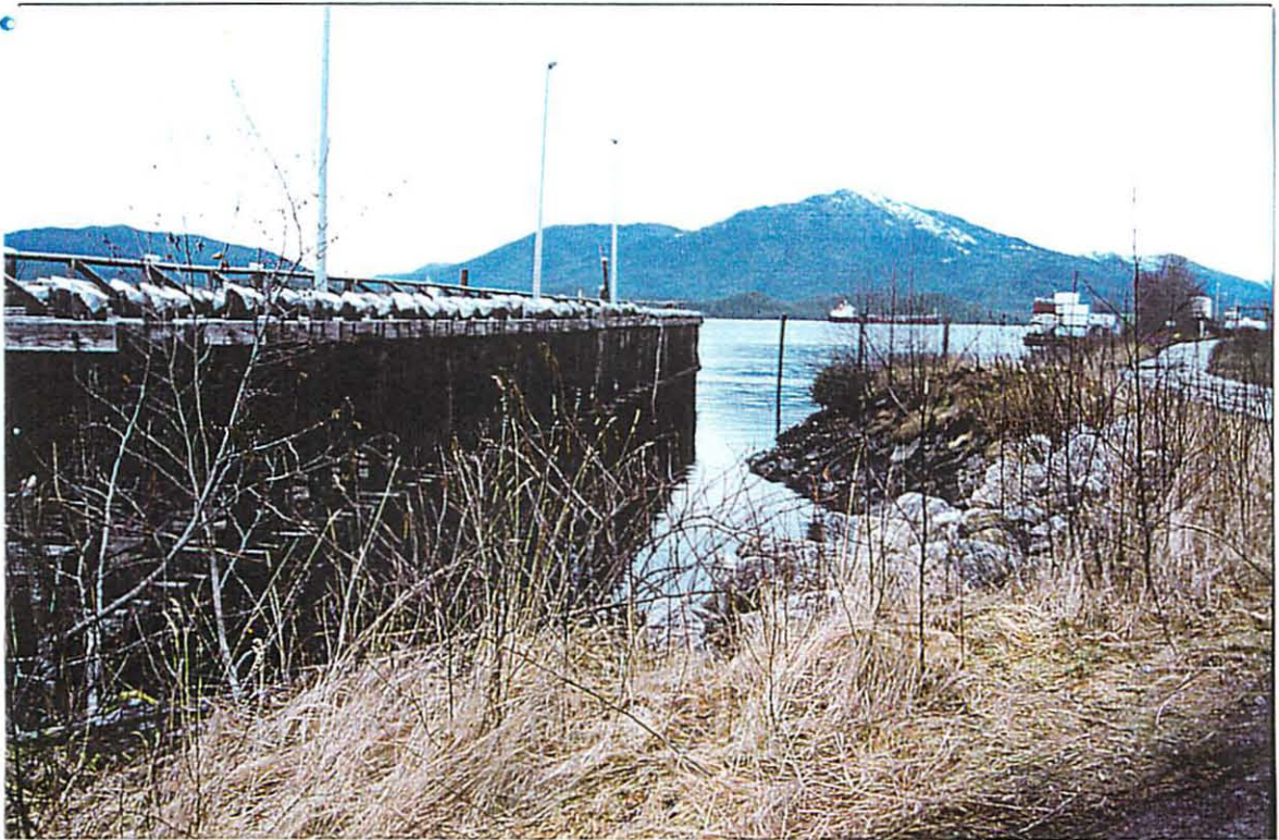
Photo #2: Viewing the back of the mooring wall. Looking North.
