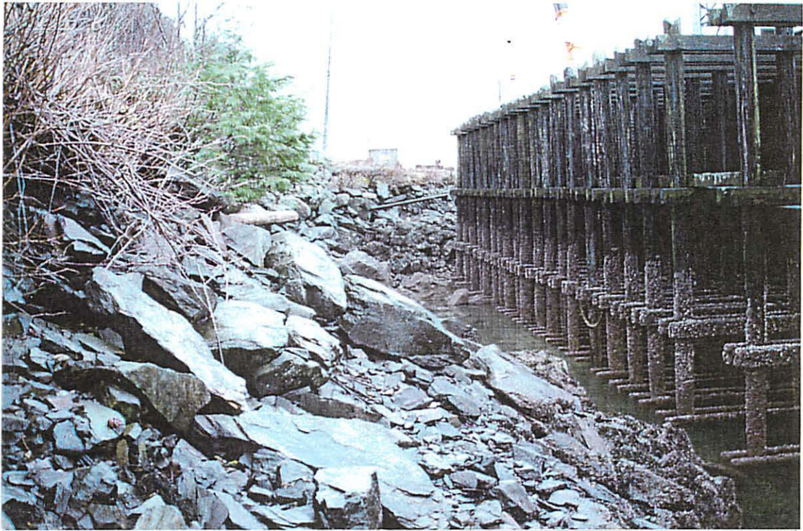
Photo #9: Looking south at the back of the mooring wall.
