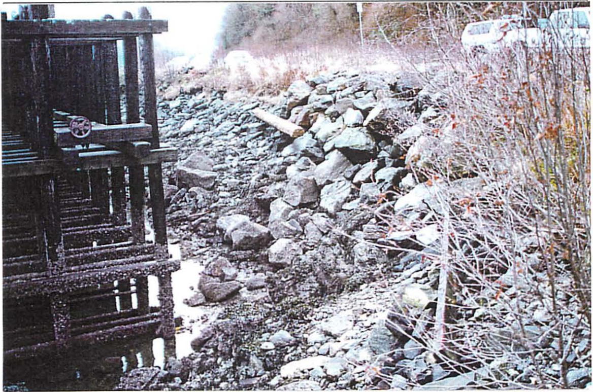
Photo #4: Looking at the south end of the mooring wall.
