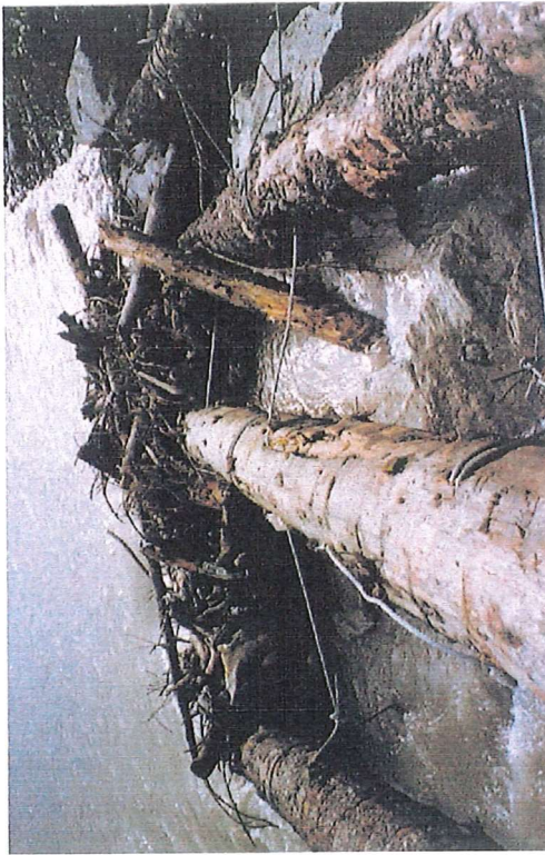
Photo 20: Copper River Debris Catcher 1. Rock ballast being anchored to trash logs to support the upstream end of the structure.
