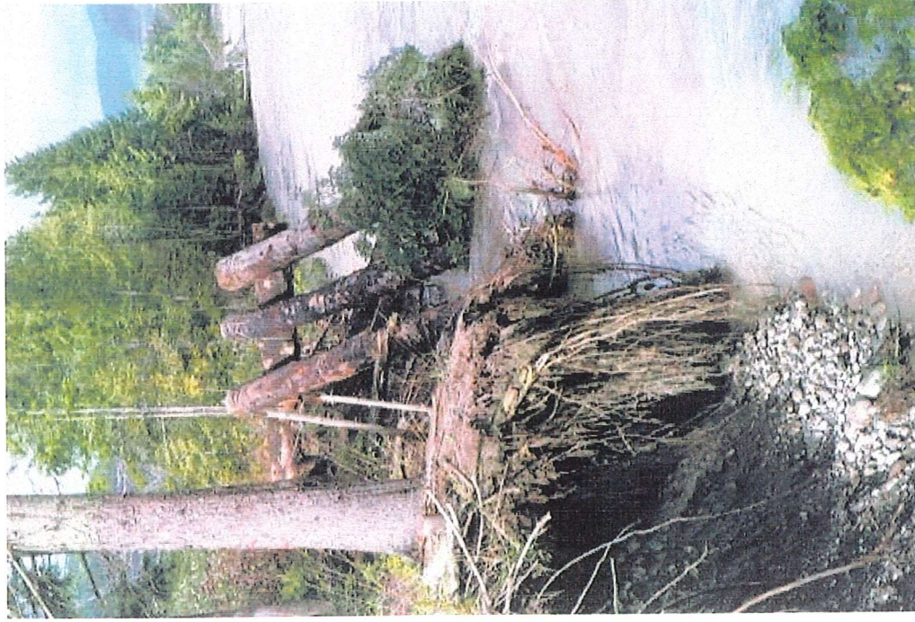
Photo 32: Copper River Debris Catcher 2. Downstream view during fall runoff (1m higher than summer). Floodwaters inundated the lower portion of the catcher. Fallen trees from eroding bank were loaded onto debris catcher in October.
