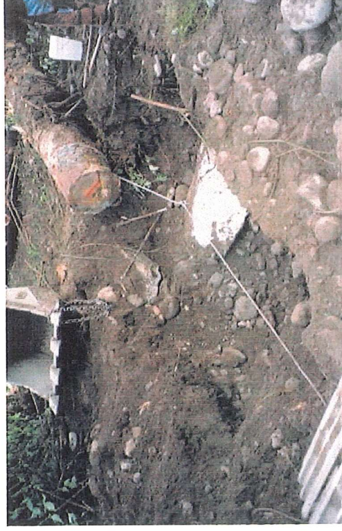
Photo 27: Copper River Debris Catcher 2. Three rocks buried adjacent to cross log. The main cable to the buried deadman (bottom left) is joined to rock as well.
