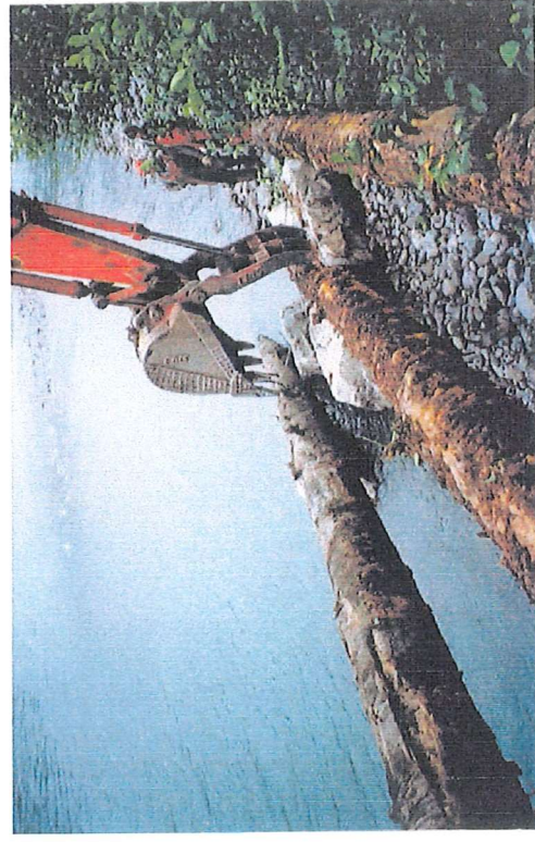
Photo 18: Copper River Debris Catcher 1. Upstream end of structure anchored to rock ballast.
