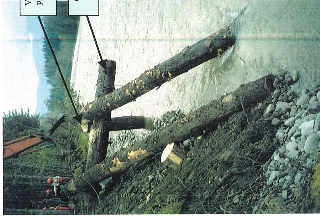
Photo 33: Copper River Debris Catcher 3. Downstream view of construction. Post is being placed under cross log.
