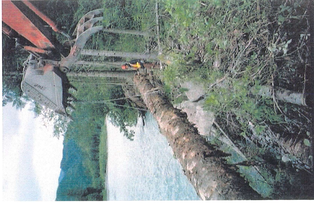
Photo 29: Copper River Debris Catcher 2. Rock ballast (approx. 3000 lbs pre rock) is hung on the second log then placed into stream channel.
