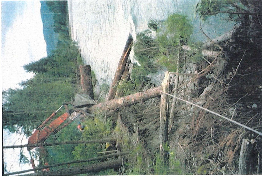
Photo 28: Copper River Debris Catcher 2. First trash log is placed on X-frame logs.
