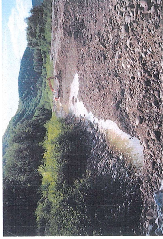
Photo 3: Copper River Site 9 Channel. Excavator backfilling the upper section of the channel.
