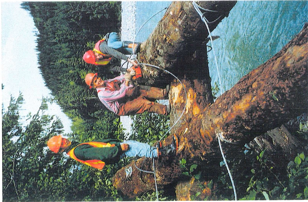
Photo 19: Copper River Debris Catcher 1. Cabling trash logs to support log. From left to right, Steve Bolton, Jack Mussel and Brian Schafhauser.
