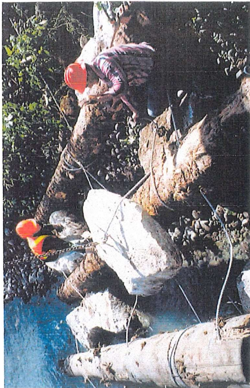
Photo 20: Copper River Debris Catcher 1. Rock ballast being anchored to trash logs to support the upstream end of the structure.
