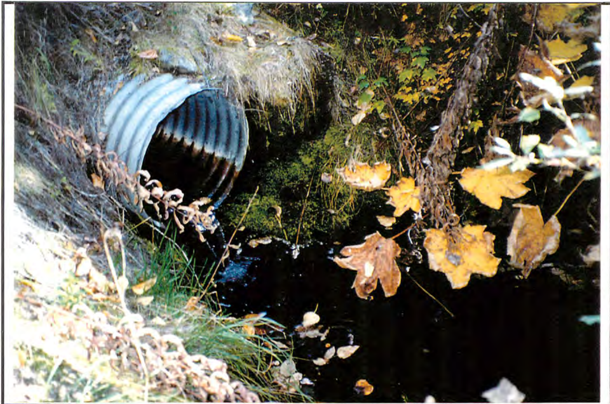
Photo 15 - A view of the downstream end of the culvert on stream 11010. This stream was classified as S4.
