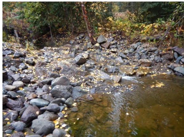
Photo 10. Moan Creek at Lawson Road – Upstream view of riffle 1 (6 m d/s culvert outlet) after construction (29 September 2017).
