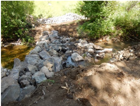
Photo 3. Johnny David Creek at Highway 16 – View from the right bank of riffle 1 (12 m d/s culvert outlet) during construction (17 July 2017).
