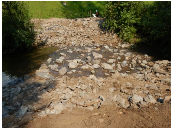
Photo 4. Johnny David Creek at Highway 16 – View from the right bank of riffle 1 (0+012 m) after construction (20 July 2017).
