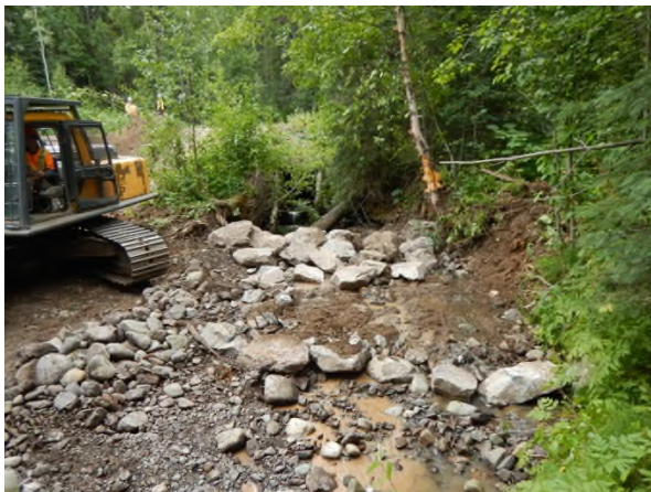
Photo 9. Moan Creek at Lawson Road – Upstream view of riffle 1 (6 m d/s culvert outlet) during construction (24 July 2017).
