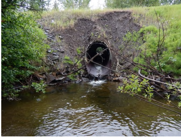
Photo 1. Johnny David Creek at Highway 16 – Upstream view of the culvert outlet prior to construction (15 July 2017).
