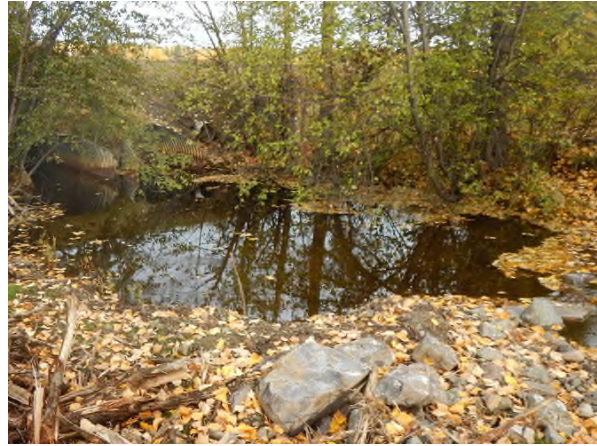
Photo 14. Tchesinkut Creek at Highway 35 – Upstream view of the culvert outlets and outlet pool after construction (30 September 2017).
