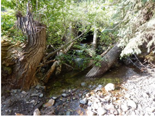
Photo 7. Moan Creek at Lawson Road – Upstream view of the culvert outlet prior to construction (21 July 2017).
