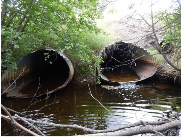
Photo 13. Tchesinkut Creek at Highway 35 – Upstream view of the culvert outlets and outlet pool prior to construction (23 July 2017).
