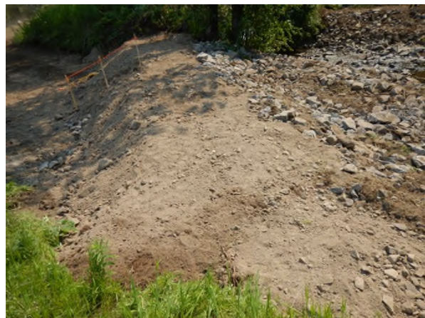
Photo 6. Johnny David Creek at Highway 16 – Downstream view of the left-bank berm after construction (20 July 2017).
