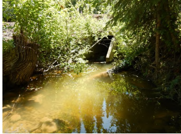
Photo 8. Moan Creek at Lawson Road – Upstream view of the culvert outlet after construction (24 July 2017).
