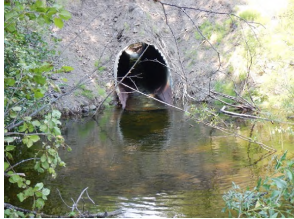
Photo 2. Johnny David Creek at Highway 16 – Upstream view of the culvert outlet after construction (20 July 2017).
