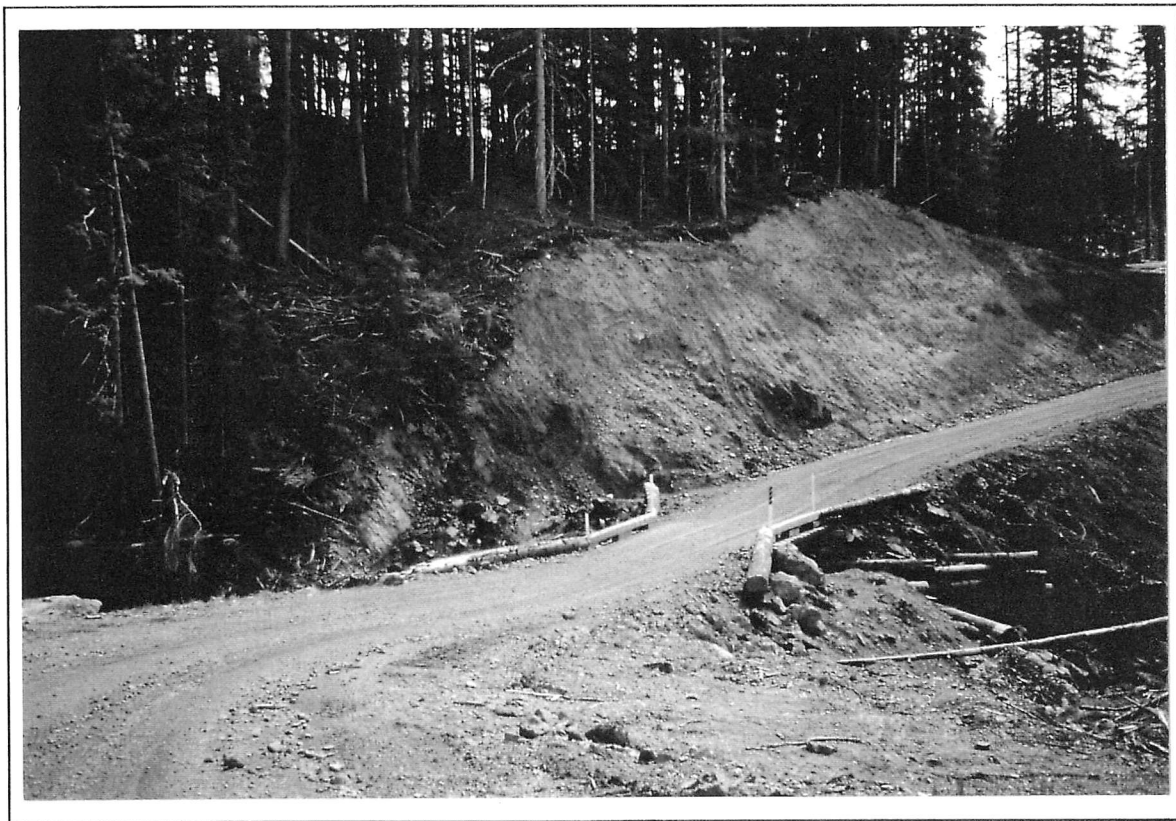
Figure 3.6) The photo above was taken at the Irvine Creek crossing on the McDonell Main Road. The bridge was built over a narrow red zoned corridor of the creek after approval by a Professional Engineer. According to map 93L.081 (Maynard 1994), the bridge crosses class V terrain with a H surface erosion potential and active gully erosion and/or landsliding. Care must be taken to ensure that erosion does not occur on the exposed cutbank and flow into the creek along the ditch. Grass seeding of the slope should be carried out for this purpose. Continued inspection and maintenance will be required for as long as the bridge exists.
