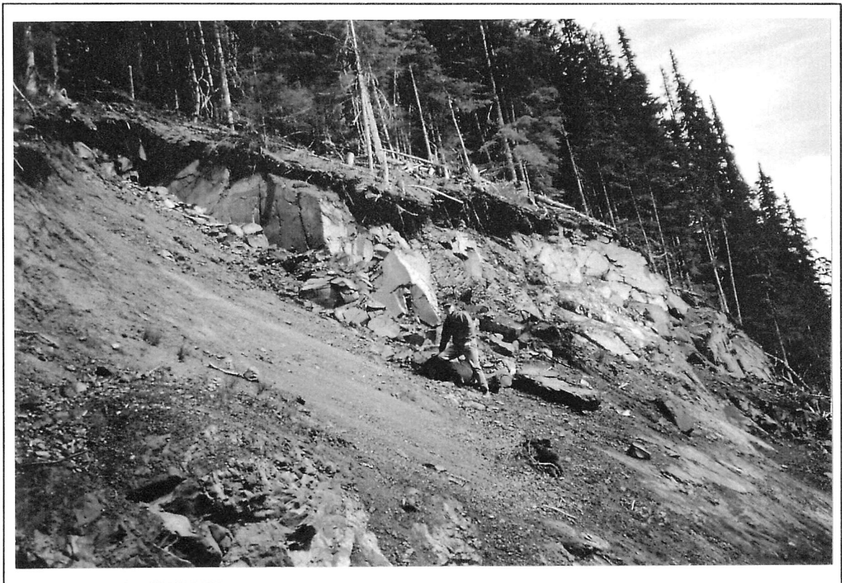
Figure 3.3) This recent, road initiated, small scale rockfall event was found on the McDonell Main Road approximately 150 metres west of the Irvine Creek crossing. As an orange 2 zone (of moderate concern), problems of instability can be expected following road building or clearcutting. This terrain is of stability class IV with a moderate (M) surface erosion potential (Maynard 1994, map 93L.081).
