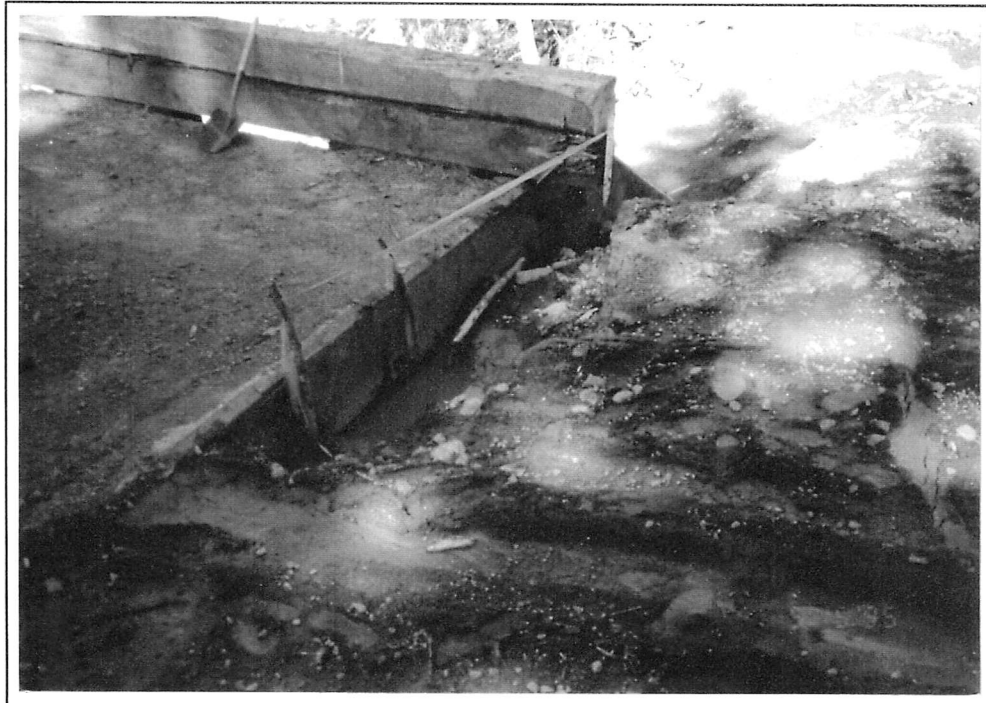
Figure 3.7a above & 3.7 b below) Red zoned terrain at this unnamed creek crossing at kilometre 3.7 on the South Copper Mainline was interpreted to be of stability class V with a very high (VH) surface erosion potential. Active rockfall and gully erosion by water and/or landsliding is also present (Maynard 1994, map 93L.072). At the time of this photograph, proper water management and erosion control precautions had not been taken at this location. As a result, runoff was eroding the soil foundation of the bridge and other disturbed areas, transporting it into the creek. (L. Vanderstar, personal communication, May 1995)
