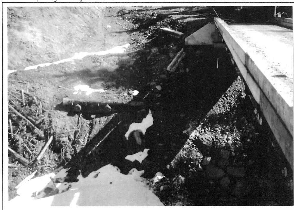
Figure 3.7a above & 3.7 b below) Red zoned terrain at this unnamed creek crossing at kilometre 3.7 on the South Copper Mainline was interpreted to be of stability class V with a very high (VH) surface erosion potential. Active rockfall and gully erosion by water and/or landsliding is also present (Maynard 1994, map 93L.072). At the time of this photograph, proper water management and erosion control precautions had not been taken at this location. As a result, runoff was eroding the soil foundation of the bridge and other disturbed areas, transporting it into the creek. (L. Vanderstar, personal communication, May 1995)
