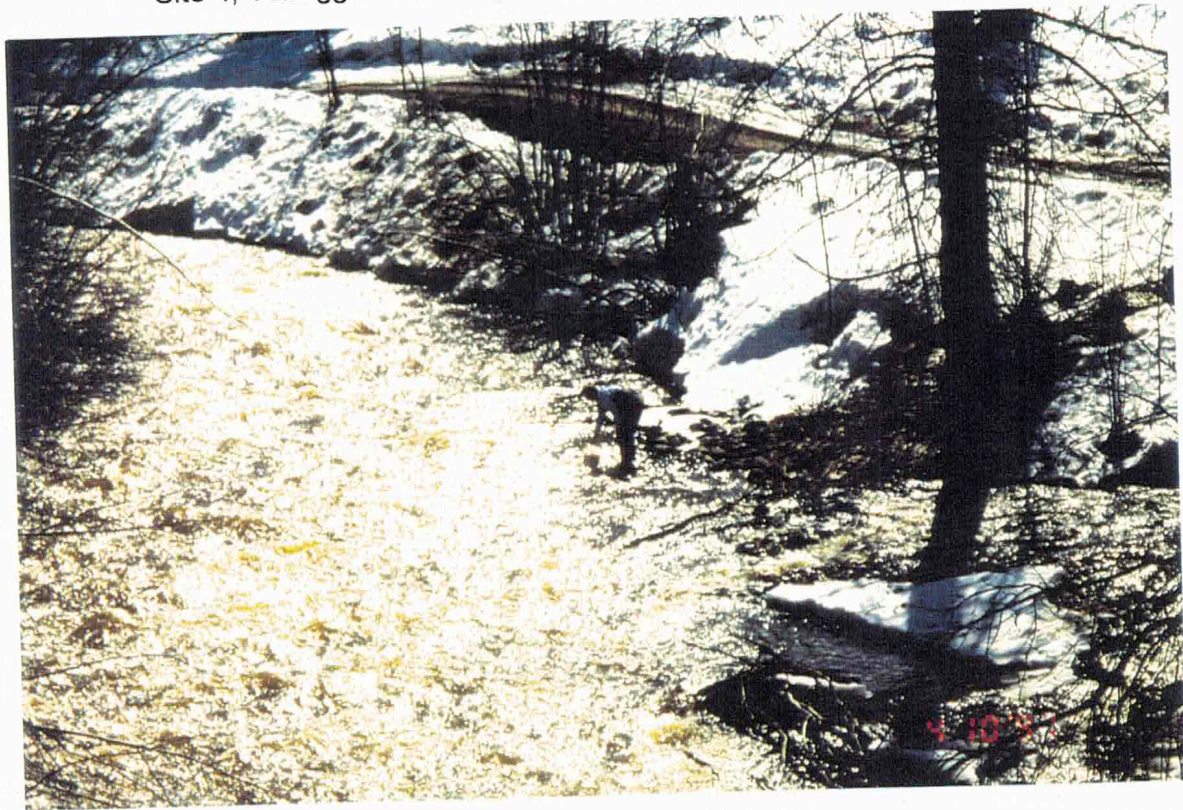
Site 5, Toboggan Creek upstream Highway 16 culvert
