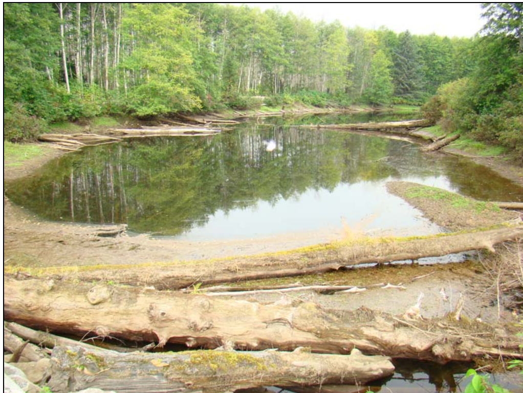
Figure 8 – The backchannel at Site 2 on September 18 th , before the lower water connection to the outlet culverts at Site 3 was opened up.
