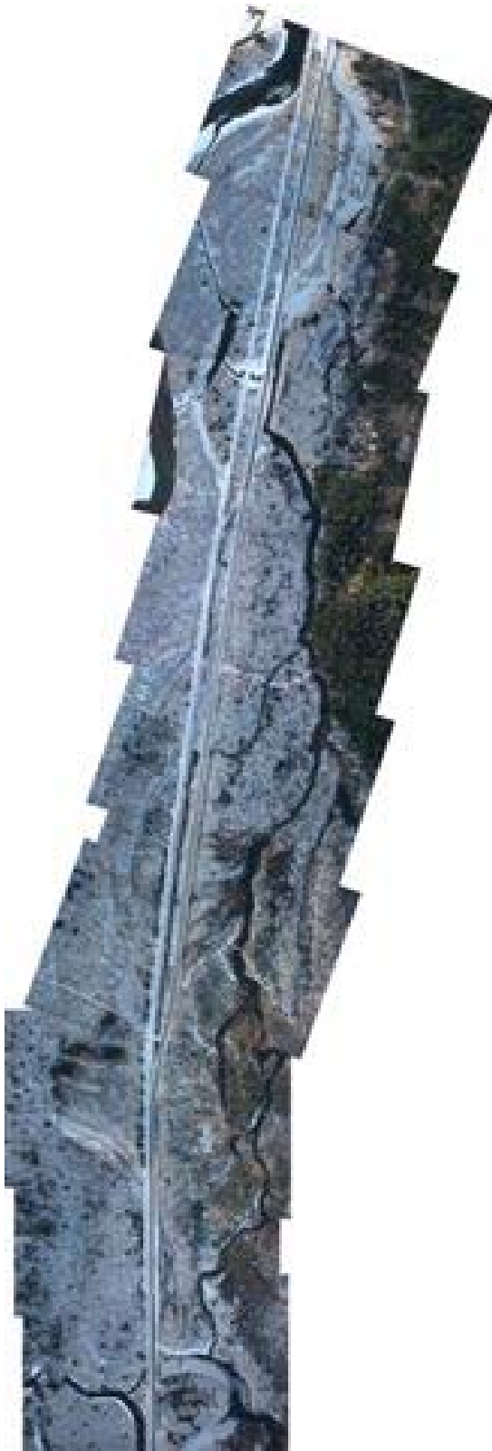
The west half of the project. North is on the right of the page.
