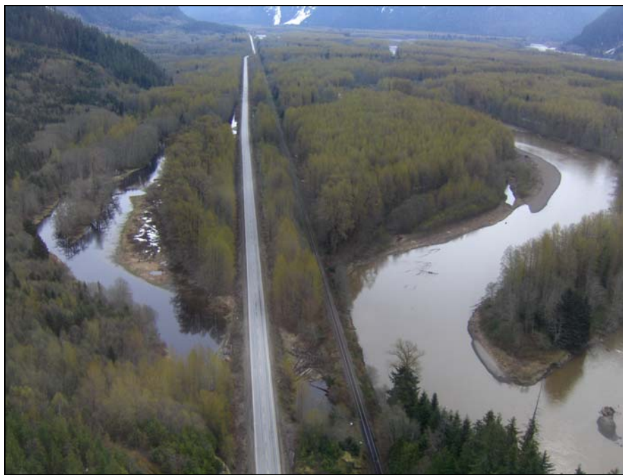
Figure 3: An aerial view of the Site 3 and Site 4, looking east, May 2007.
