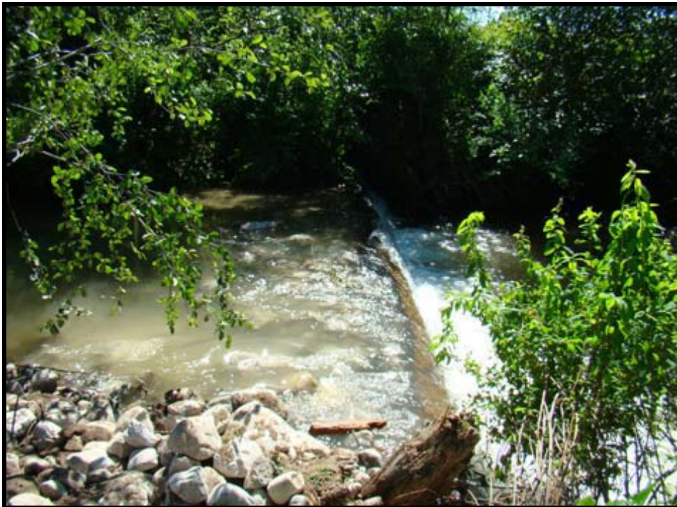
Photo 10 - Scully Creek - reinforced log weir at downstream end of one of the spawning platforms.
