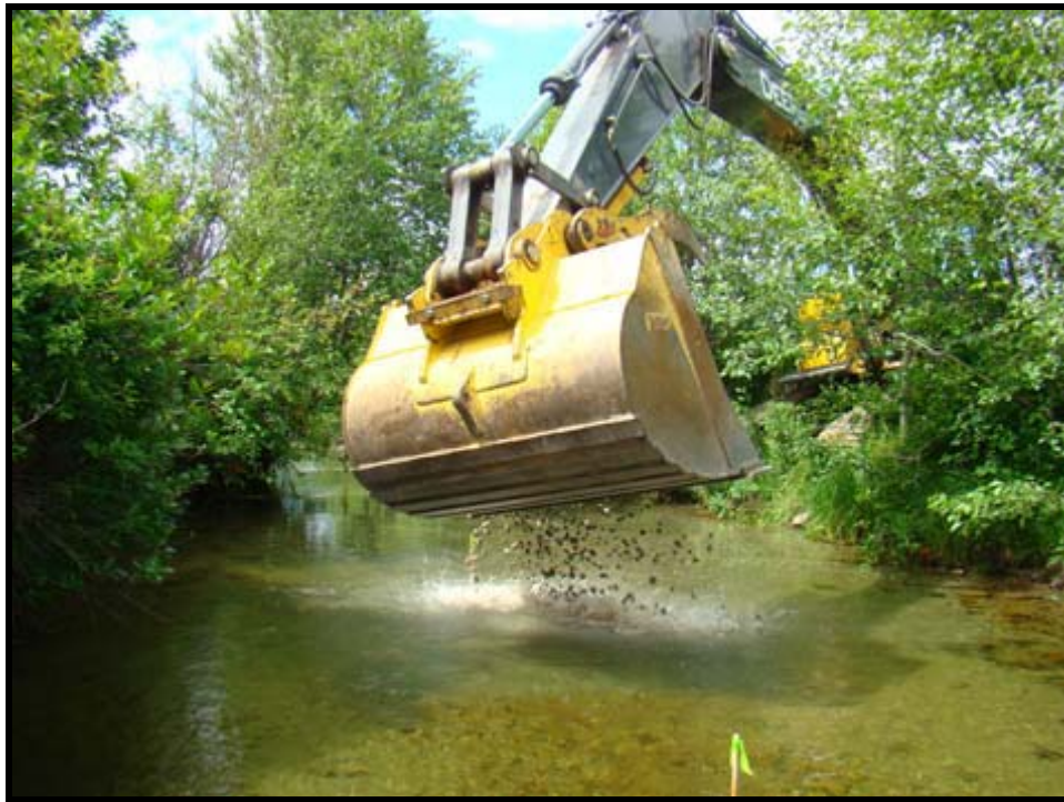
Photo 3 - Gravel being placed in Scully Mid-Channel by excavator.
