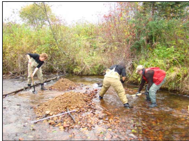
Photo 20 – Digging to install incubation boxes
