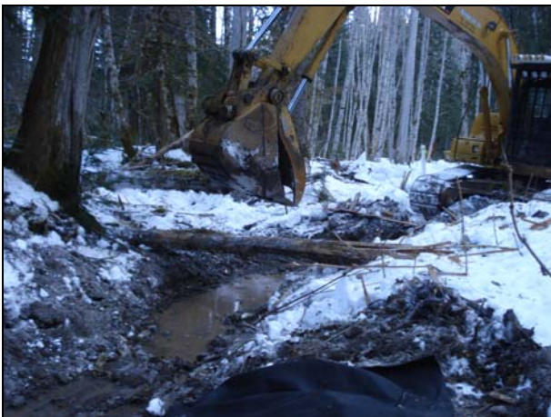
Photo 53 – Excavation worked from downstream to Upstream.
