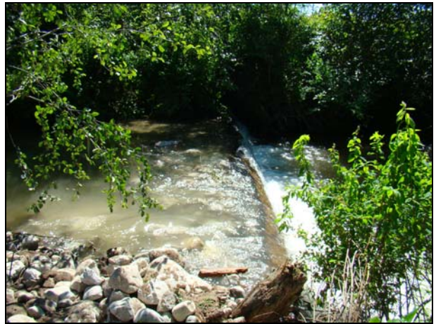
Photo 8 – Rock added behind the log to strengthen the weir.
