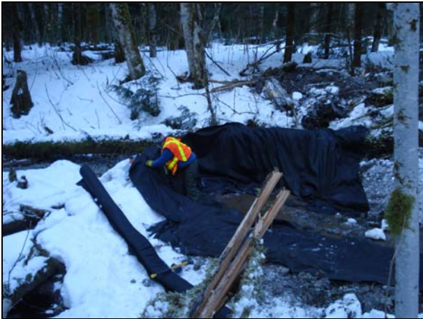
Photo 51 – Installing sediment control
