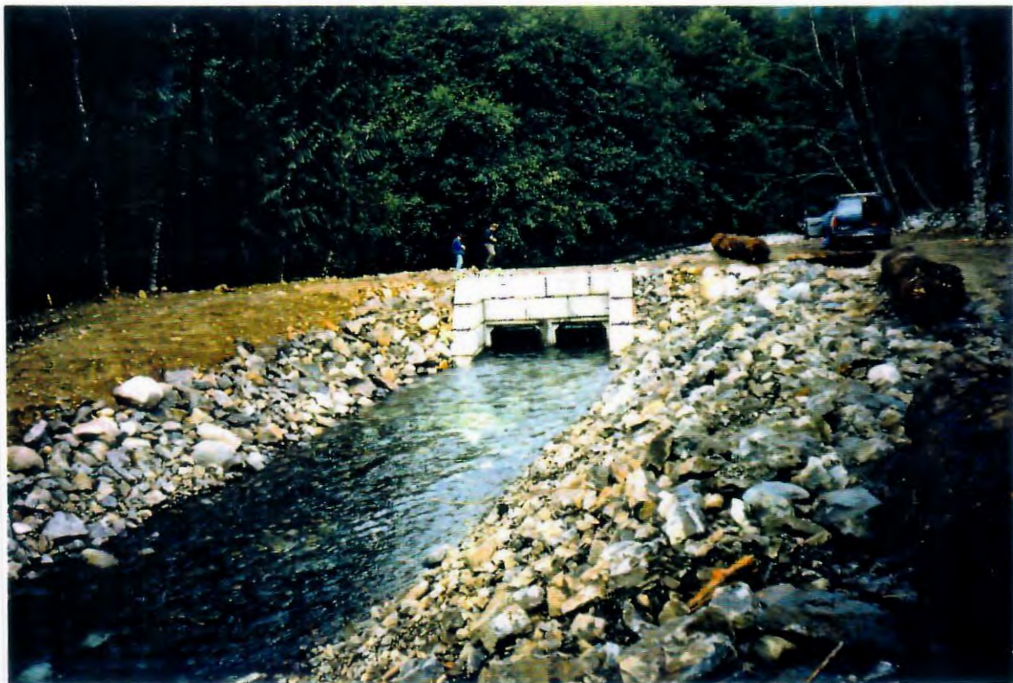
Photo 10. Water intake structure at Chilliwack River.
