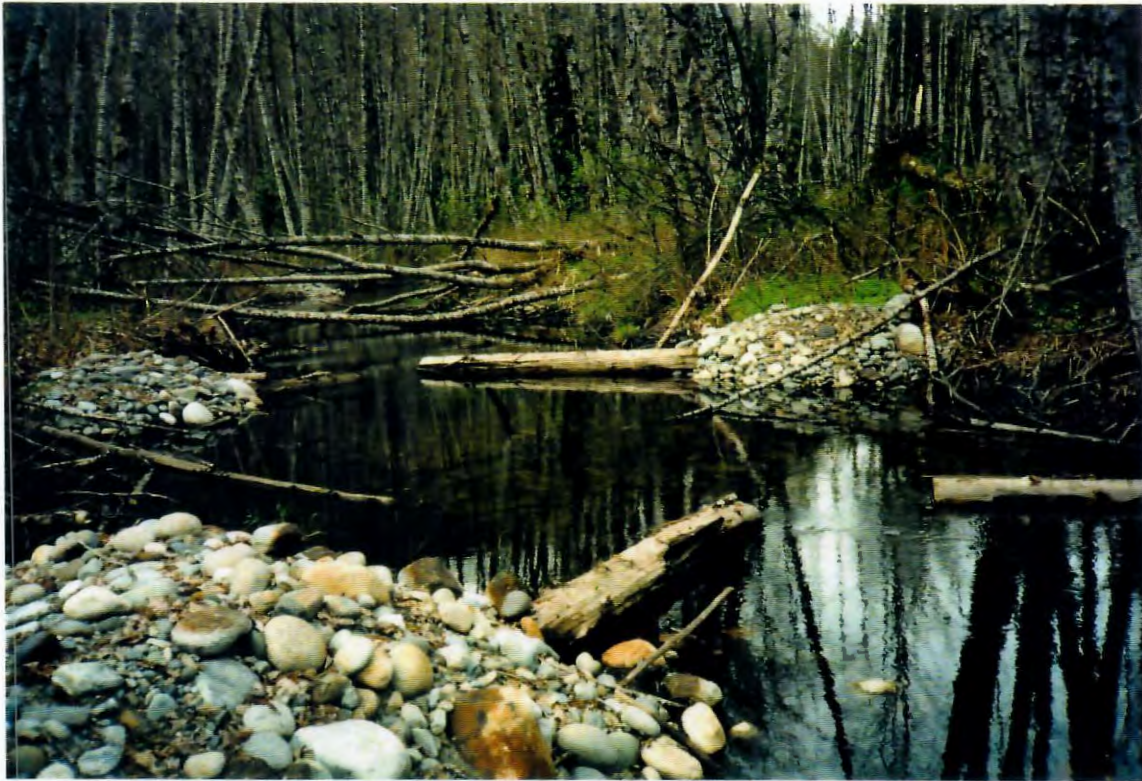
Photo 10. V-log weirs were installed by loading excavated bed materials on logs keyed into banks, and a log cover was attached to increase habitat complexity.
