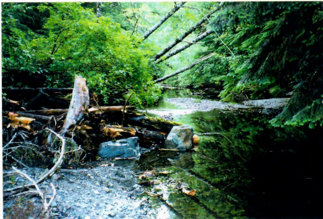
Photos 1 & 2. Streambank log jams were created at W80 sites which also capture large woody debris along the stream margin during high flows: key logs were secured by attaching large boulders. Prime juvenile salmonid rearing and overwintering habitat is provided, as well as cover for spawners.
