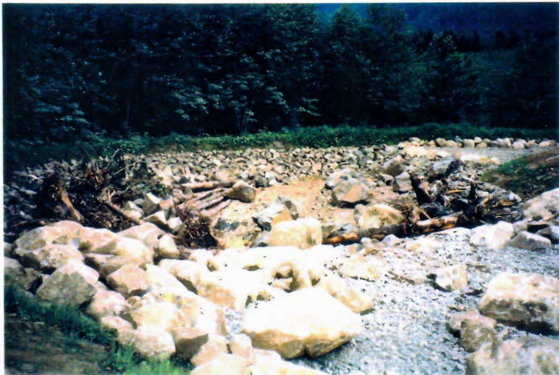
Photo 7. Gravel placement and channel complexing.
