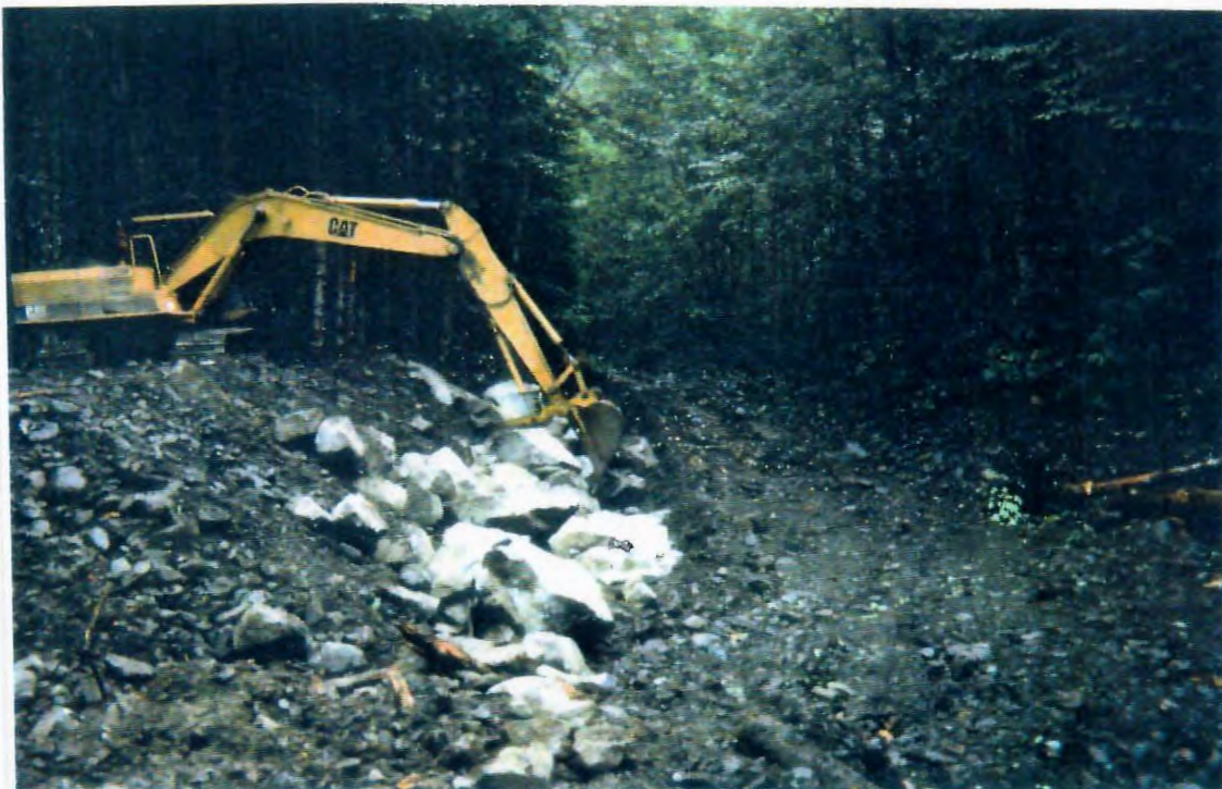
Photo 8. Construction of berm to protect avulsion channel which enters an old road creating a new channel impacting fish habitat.
