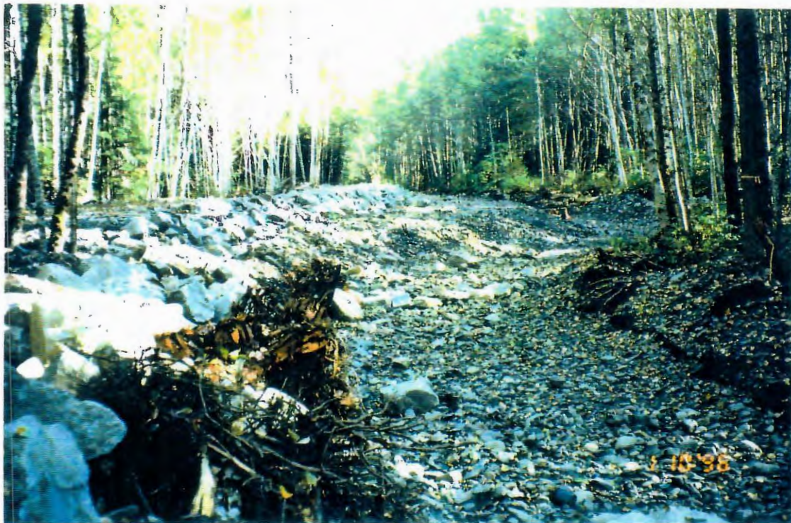
Photo 10. Completed berm - more large woody debris and boulder complexing to be installed.
