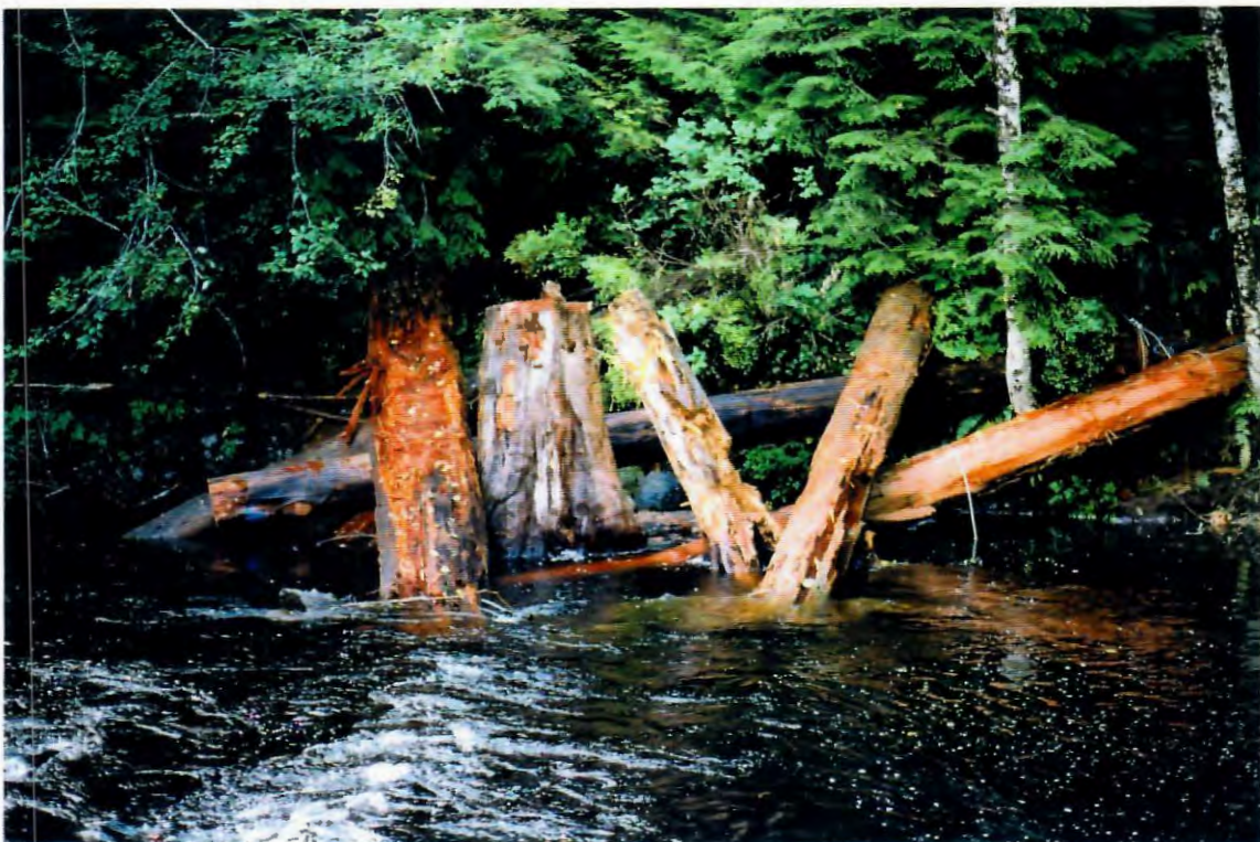
Photo 6. '80 bridge, site 18 after fish habitat rehabilitation.
