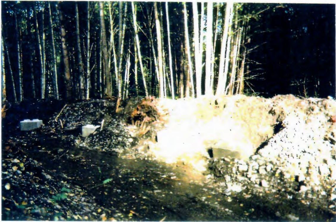
Photo 3. Anchor blocks placed in pits.
