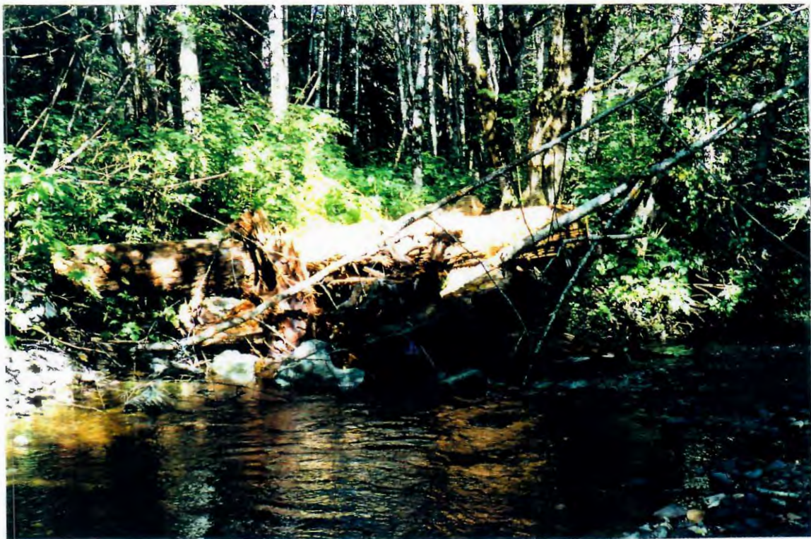
Photo 10. Streambank stabilization and provision of overhead cover with large woody debris secured to boulders at West Main site.
