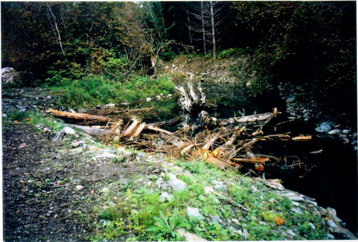
Photo 5. Constructed pond with large woody debris and rootwad placements for a juvenile overwintering refuge for coho.
