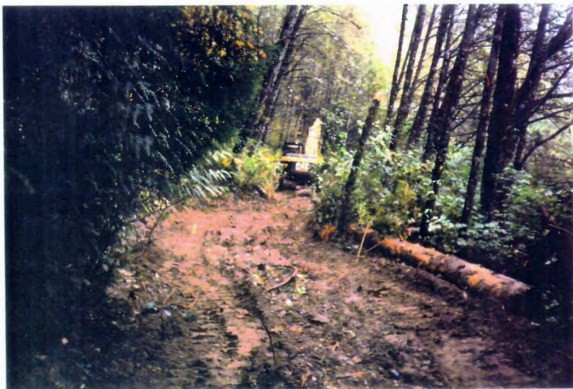
Photo 11 Excavator digging channel at lowermost end of habitat complex.
