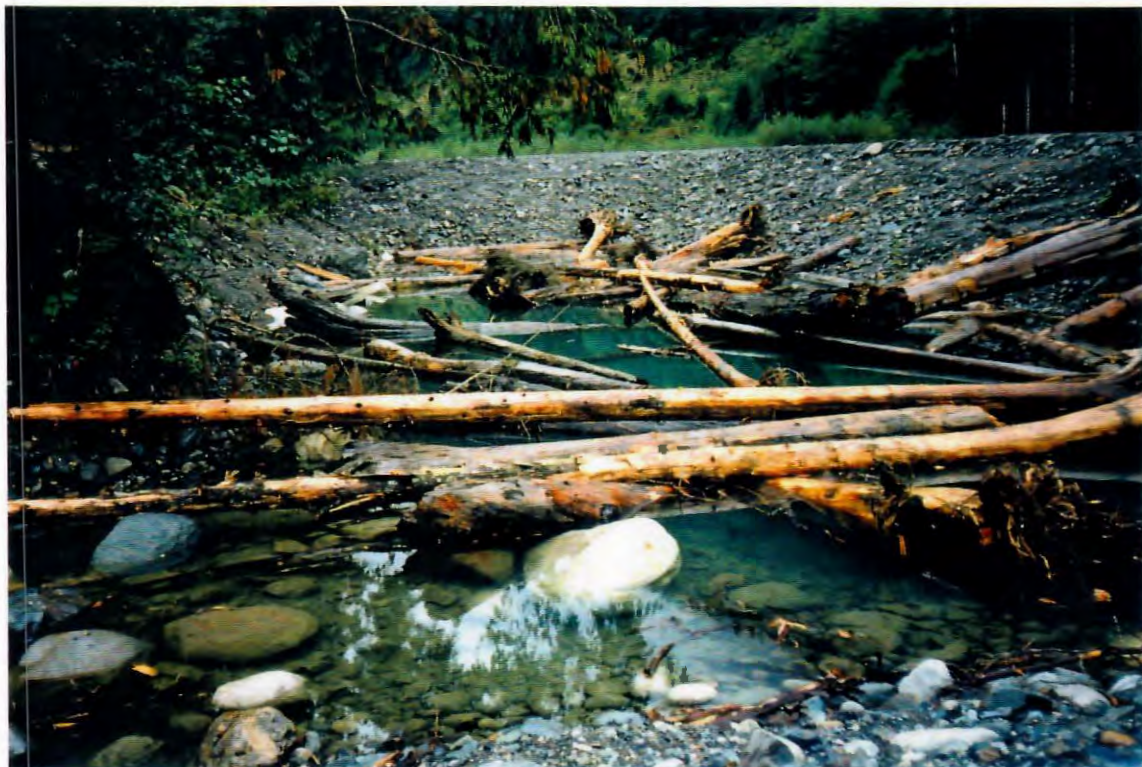
Photo 4. Constructed overwintering pond with large woody debris and rootwad placements.
