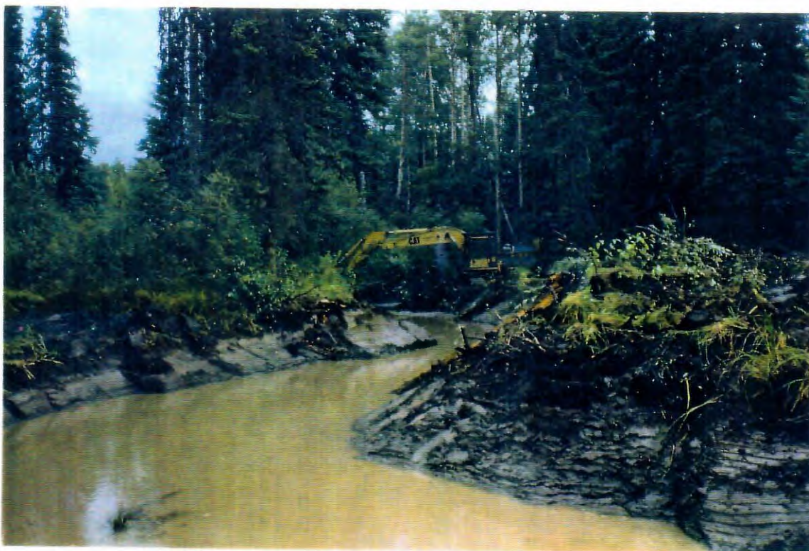
Photo 2. Excavating refuge channel between two ponds.
