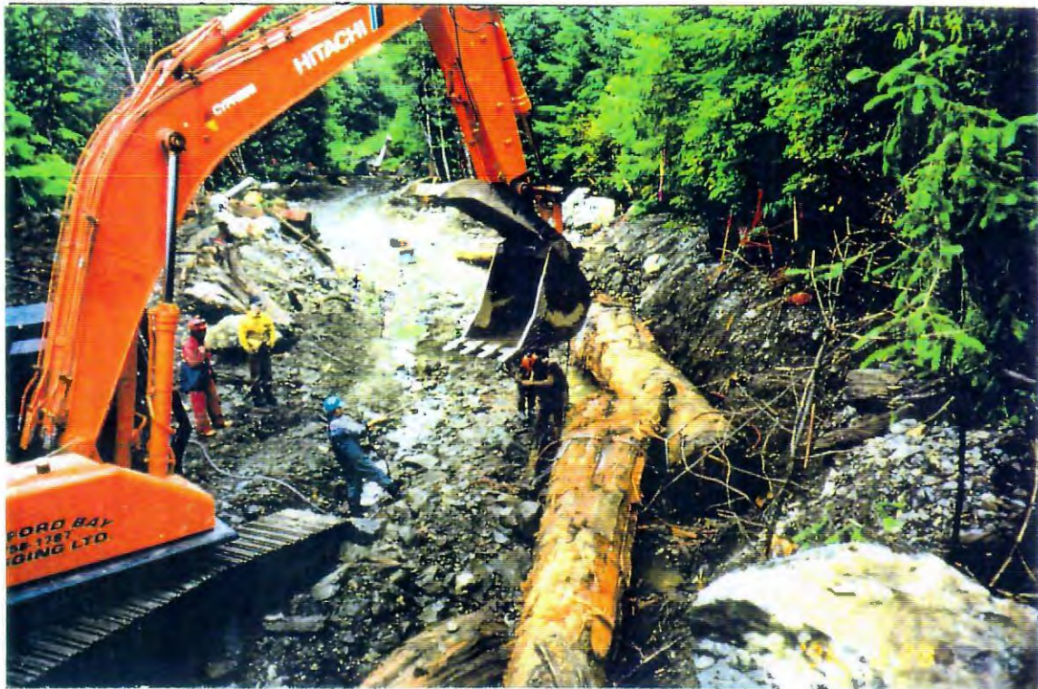
Photo 3. Construction of log bank protection at Bend 4 viewed upstream. Logs are being cabled together and have been anchored to notched stumps above the creek (note cables extending into the bush).
