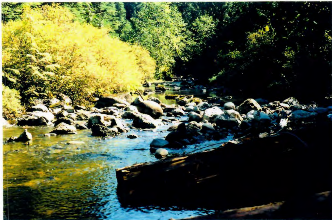
Photo 22. At this site a pool was deepened and a riffle constructed from the largest boulders available on the streambed. Future floods will help maintain this natural pool and riffle profile.
