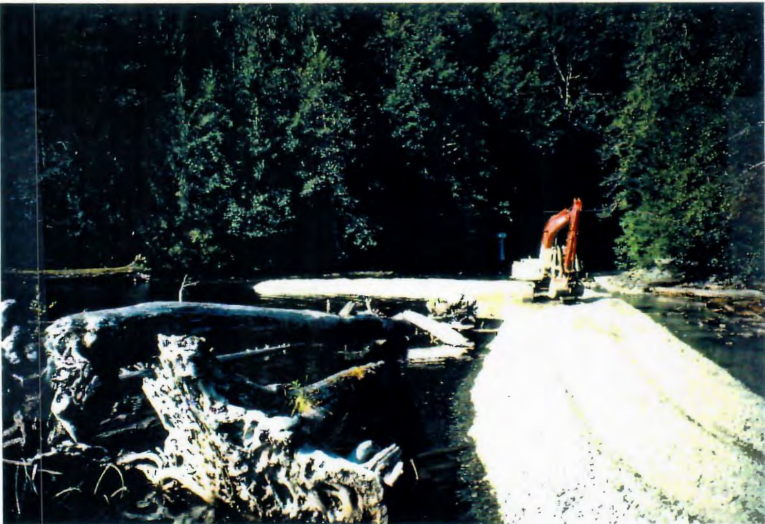
Photo 2. Gravel placed across lake outlet prior to levelling.
