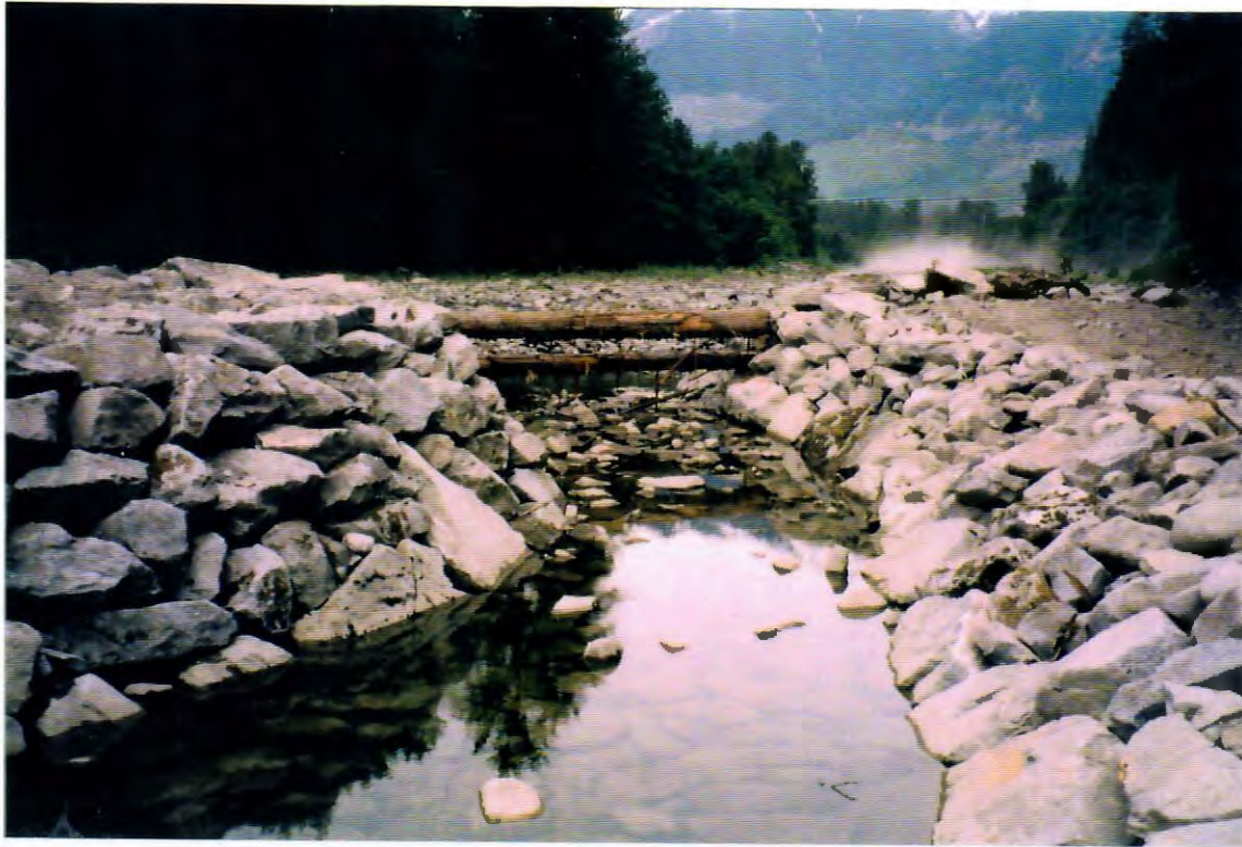
Photo 17. A controlled-flow intake and the placement of large logs across the head of Shovelnose Creek side channel to deflect floating debris.
