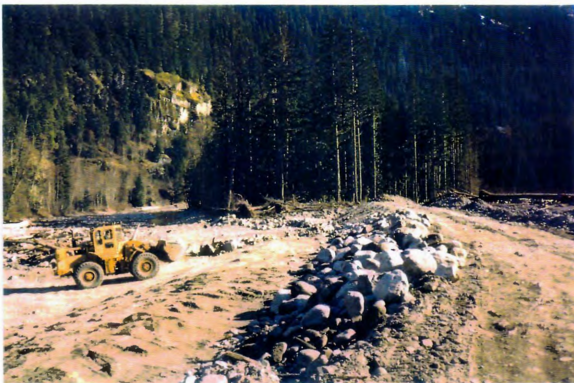
Photo 5. Rock armour placement Shovelnose Creek side.
