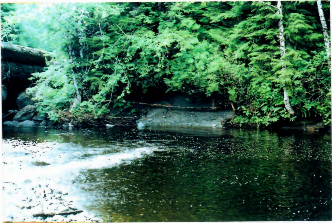
Photo 5. W80 bridge, site 18 before fish habitat rehabilitation.
