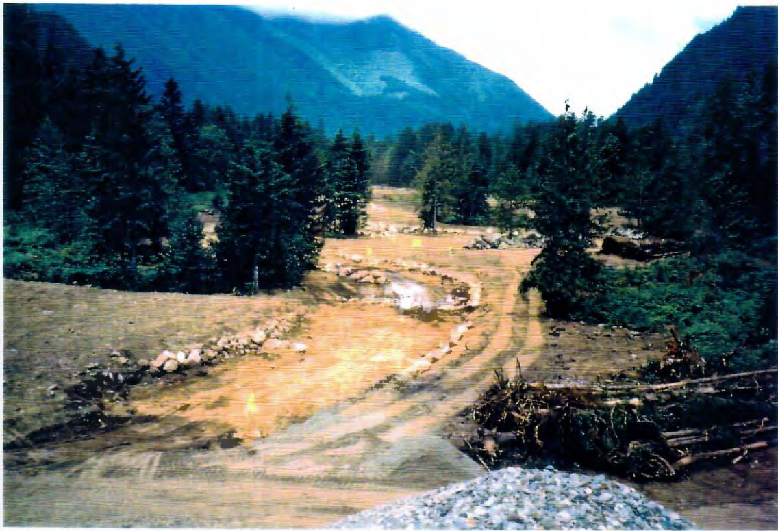
Photo 5. Armouring the channel with boulders.
