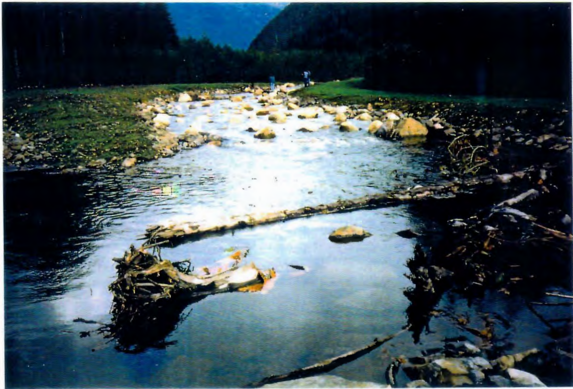
Photo 9. Centennial Trail spawning/rearing channel after construction and hand seeding (prior to hand planting of shrubs and trees by First Nations planters).
