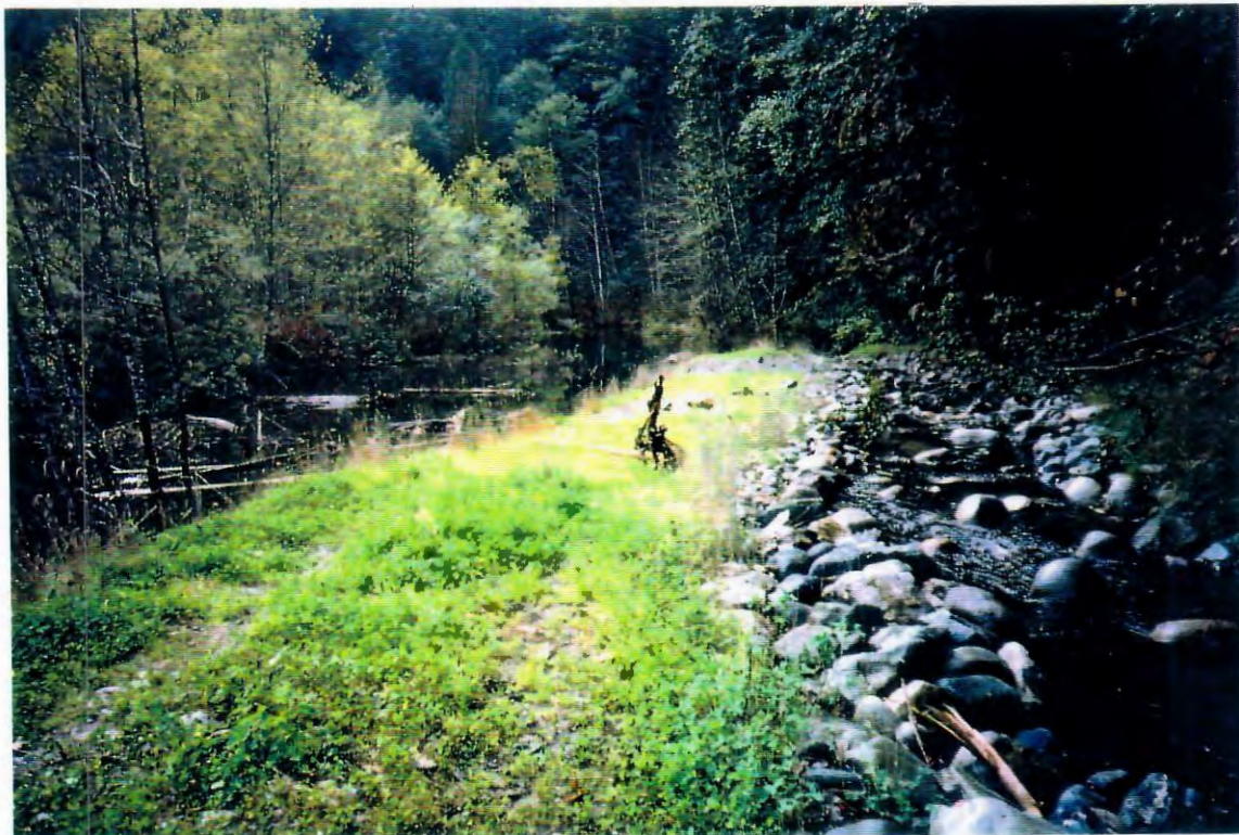
Photo 2. Completed pond and side channel with woody debris and dressed and seeded berm.
