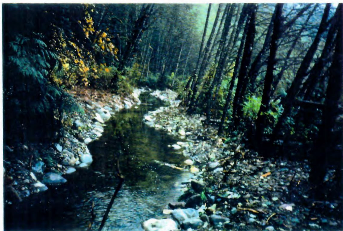
Photo 12 Completed channel taken from same angle as above photo, with outflow.
