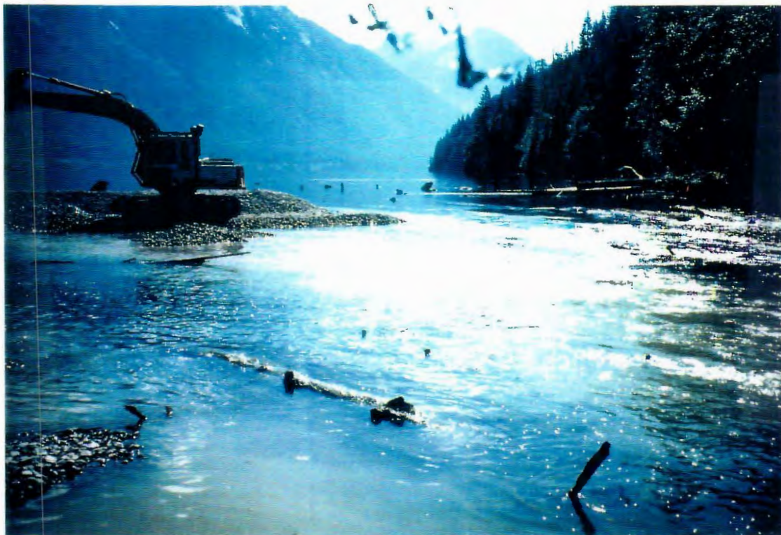
Photo 3. Excavator levelling gravel to final grade.
