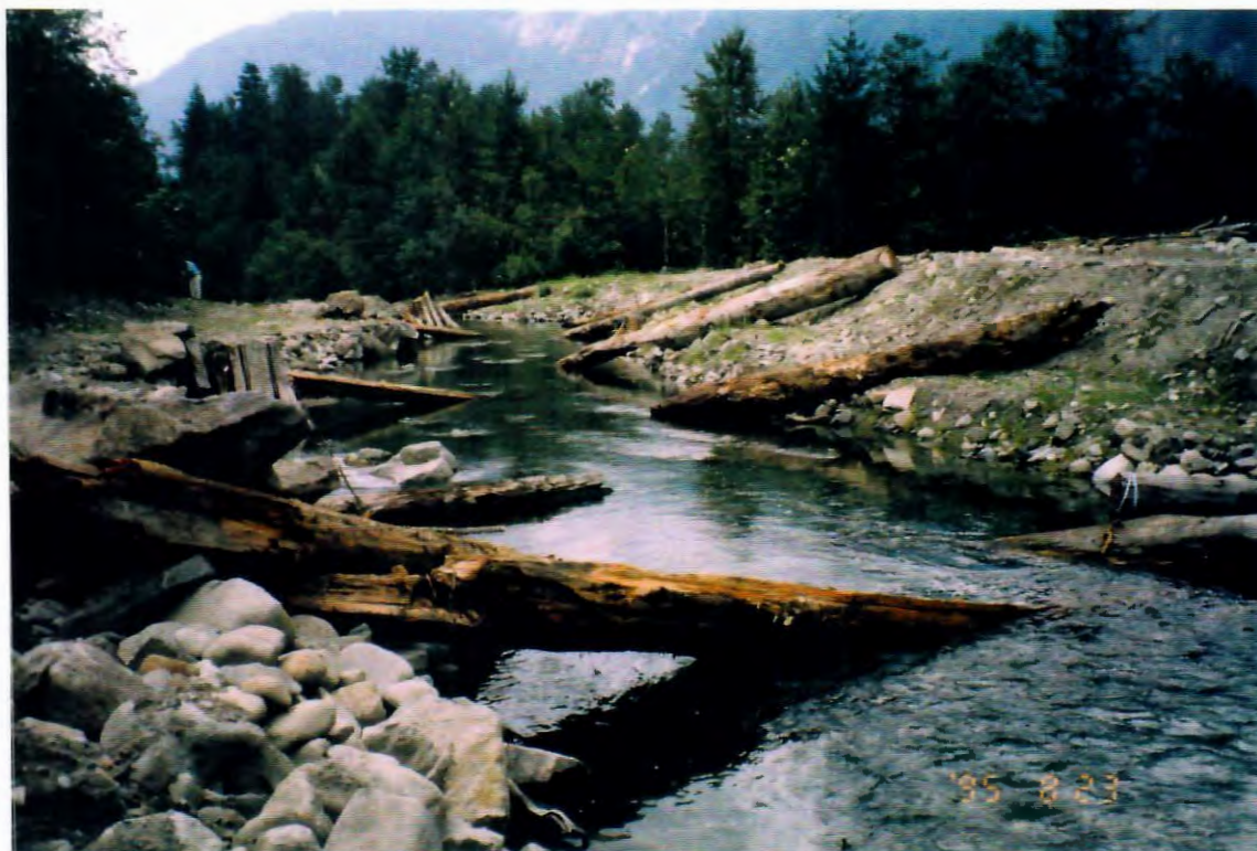
Photos 19 & 20. Selective placements of boulder clusters and holding pools in the side channel also offset habitat losses in the upper unstable reach of Shovelnose Creek.
