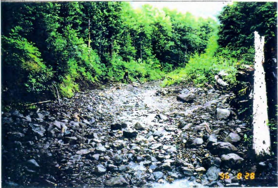
Photo 5. Completed instream work showing upstream view of Riffle 2 in the foreground.
