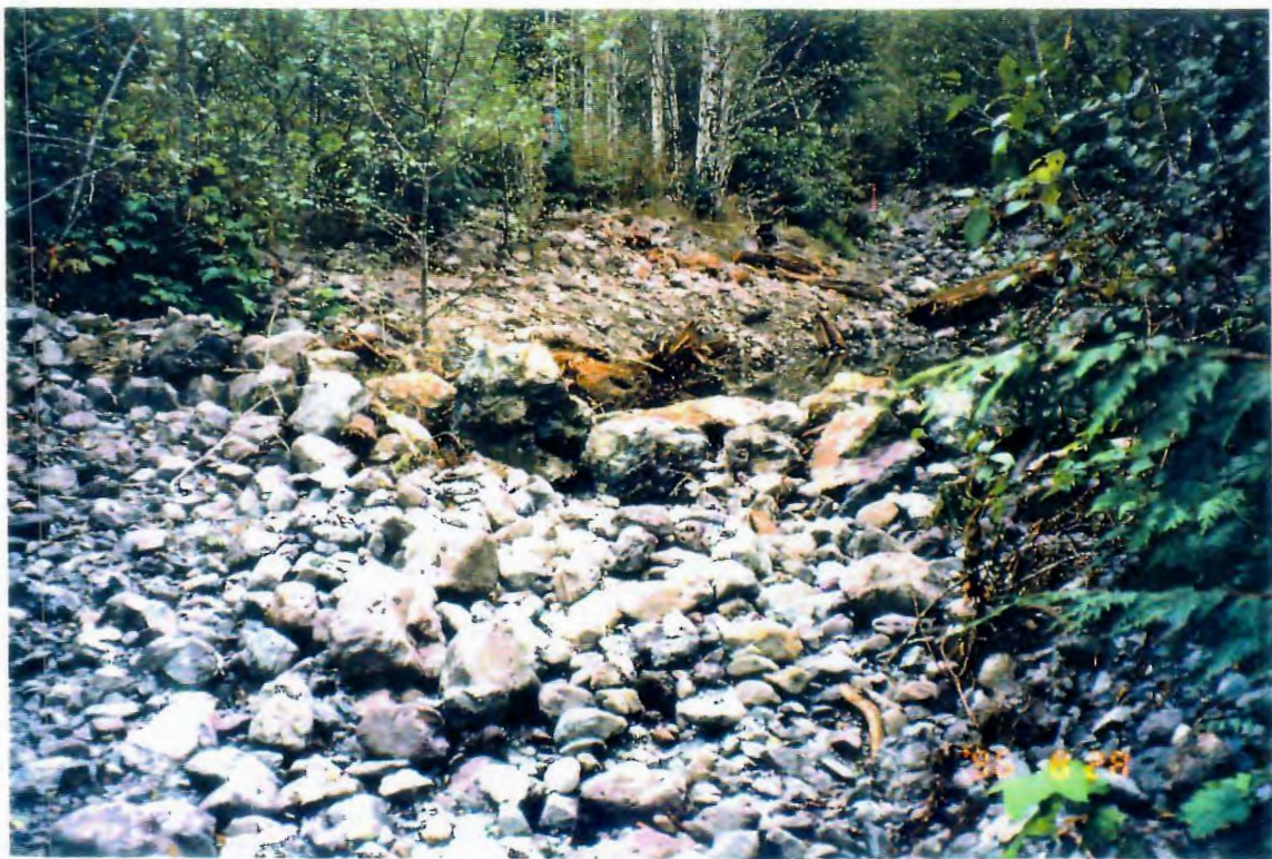
Photo 2. Historic channel (Trib. 1.37) after reconnection and reconstruction.
