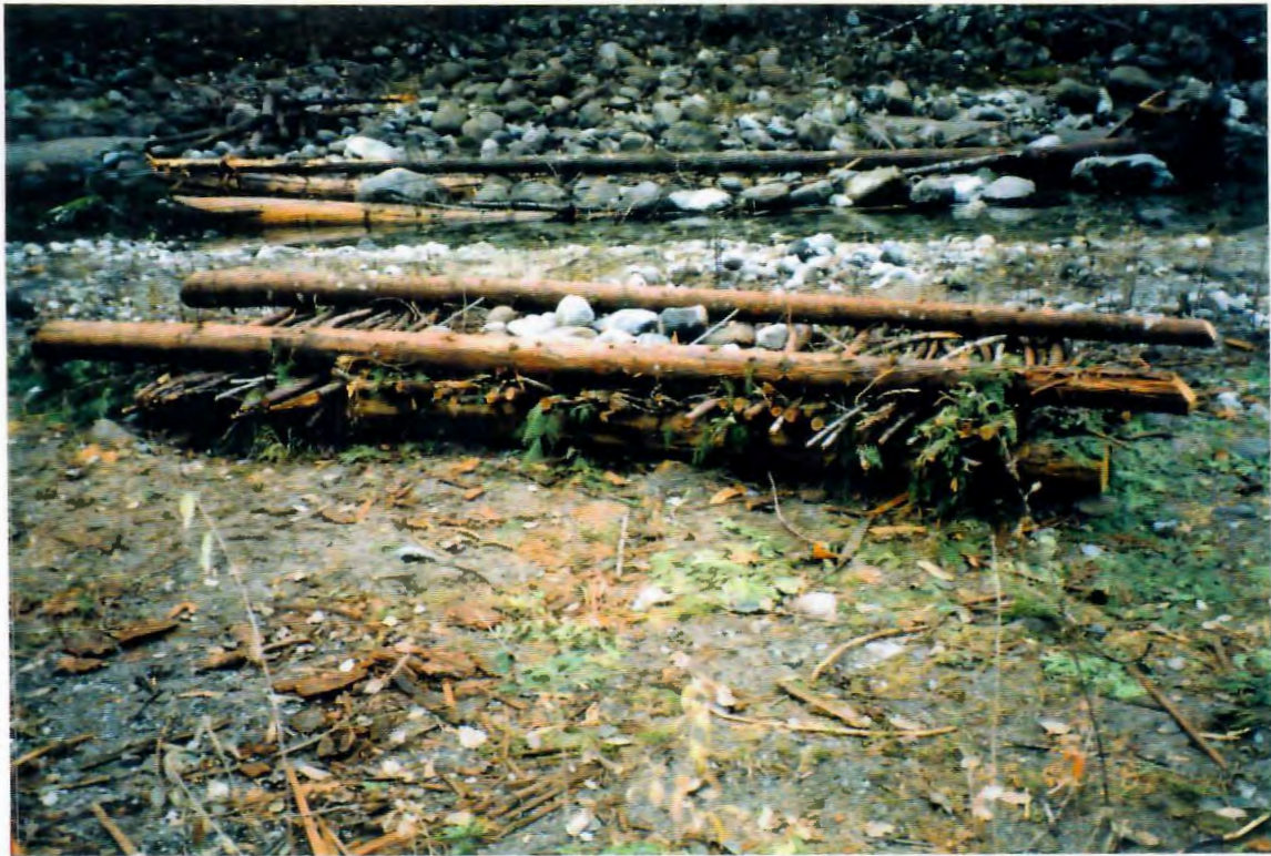
Photos 11 & 12. Artificial log reef is under construction and one is installed below. Reefs comprised of boulders and logs are well inhabited by juvenile salmon, steelhead and char and restore critical fish habitat as they are similar to (mimic) large old growth trees.
