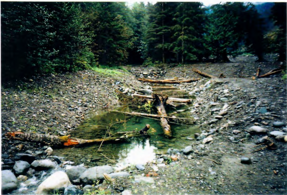
Photo 3. Constructed groundwater channel with large woody debris and boulder placements.
