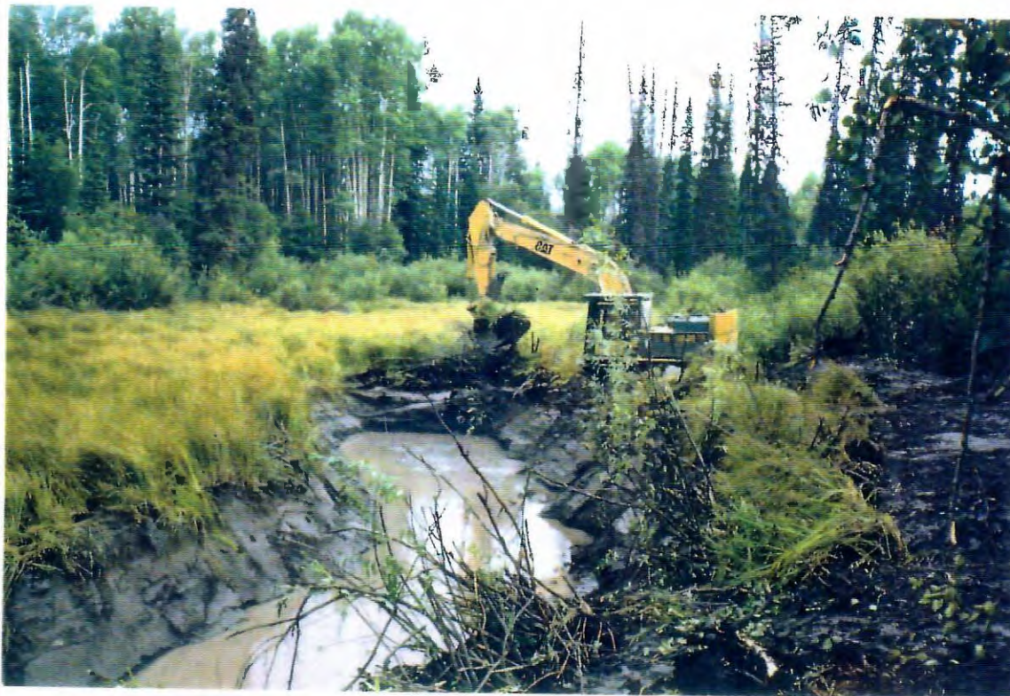
Photo 1. Excavating refuge channel within dried pond area.
