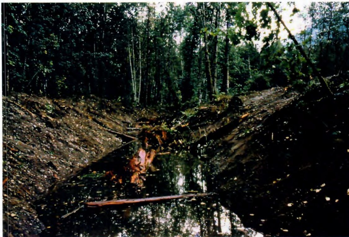
Photo 2. Completed groundwater channel on 28.5 Mile Creek, prior to revegetation.
