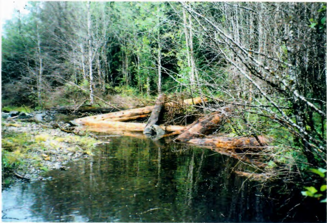
Photo 8. Streambank log jams were created at W103 to W104 sites to capture large woody debris along the stream margin during high flows: key logs were secured by attaching large boulders.
