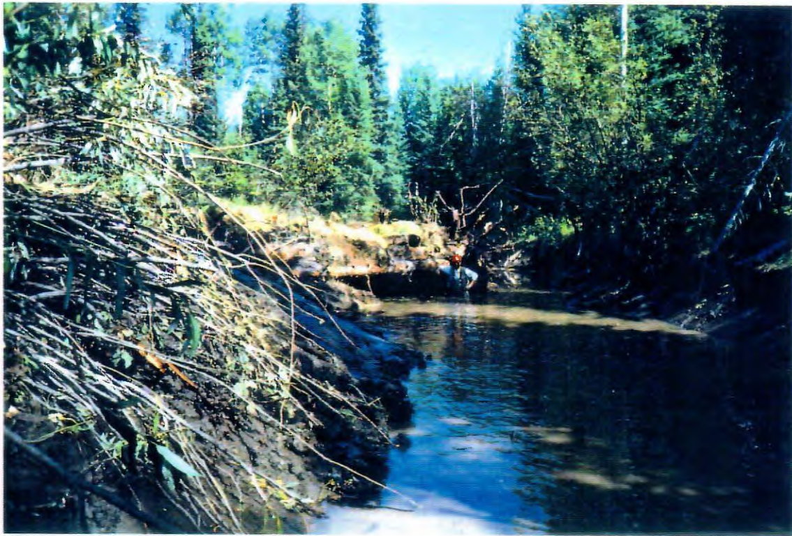
Photo 3. Artificial undercut bank (center) made by excavating notch in side slope of channel and covering with logs and then backfilling.
