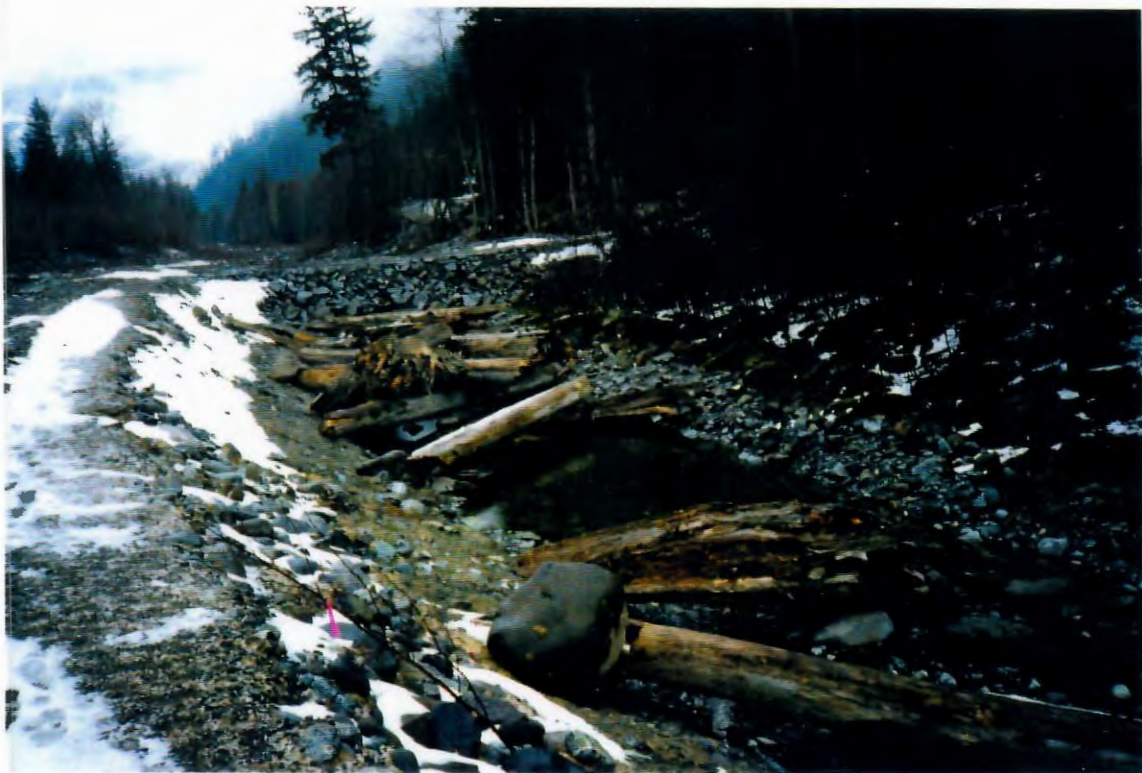
Photo 10. After construction large woody debris was added to the groundwater channel to provide cover.
