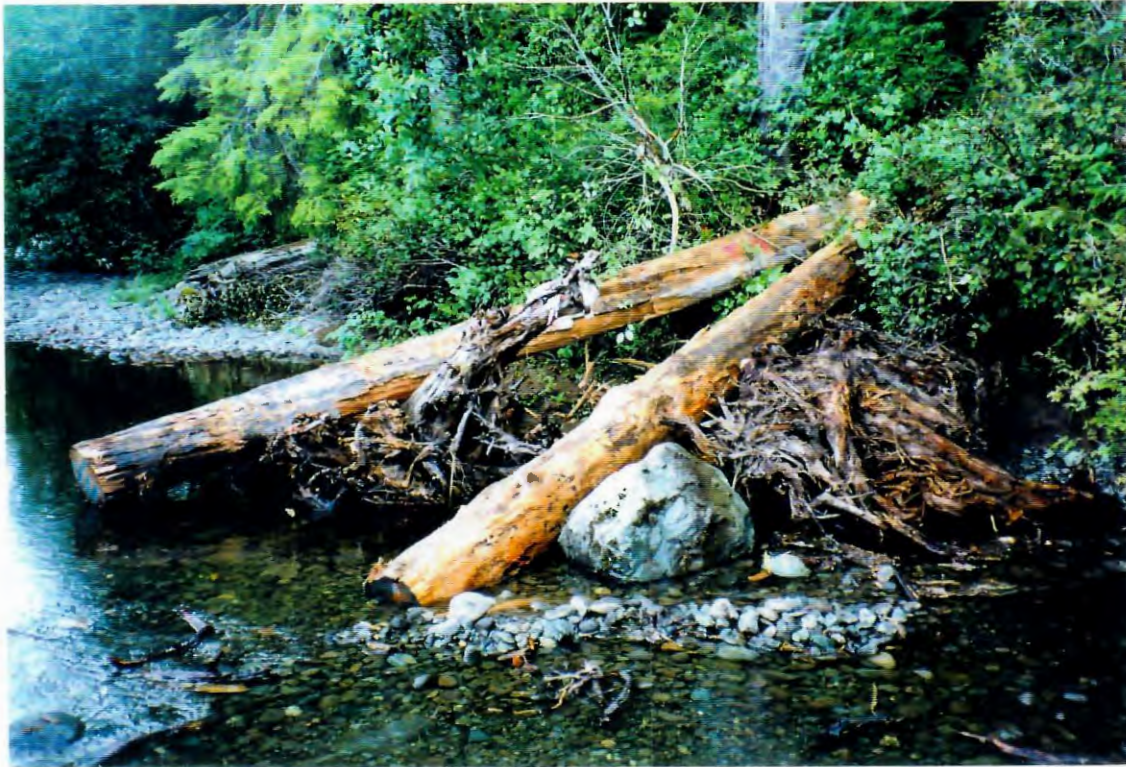
Photos 1 & 2. Streambank log jams were created at W80 sites which also capture large woody debris along the stream margin during high flows: key logs were secured by attaching large boulders. Prime juvenile salmonid rearing and overwintering habitat is provided, as well as cover for spawners.
