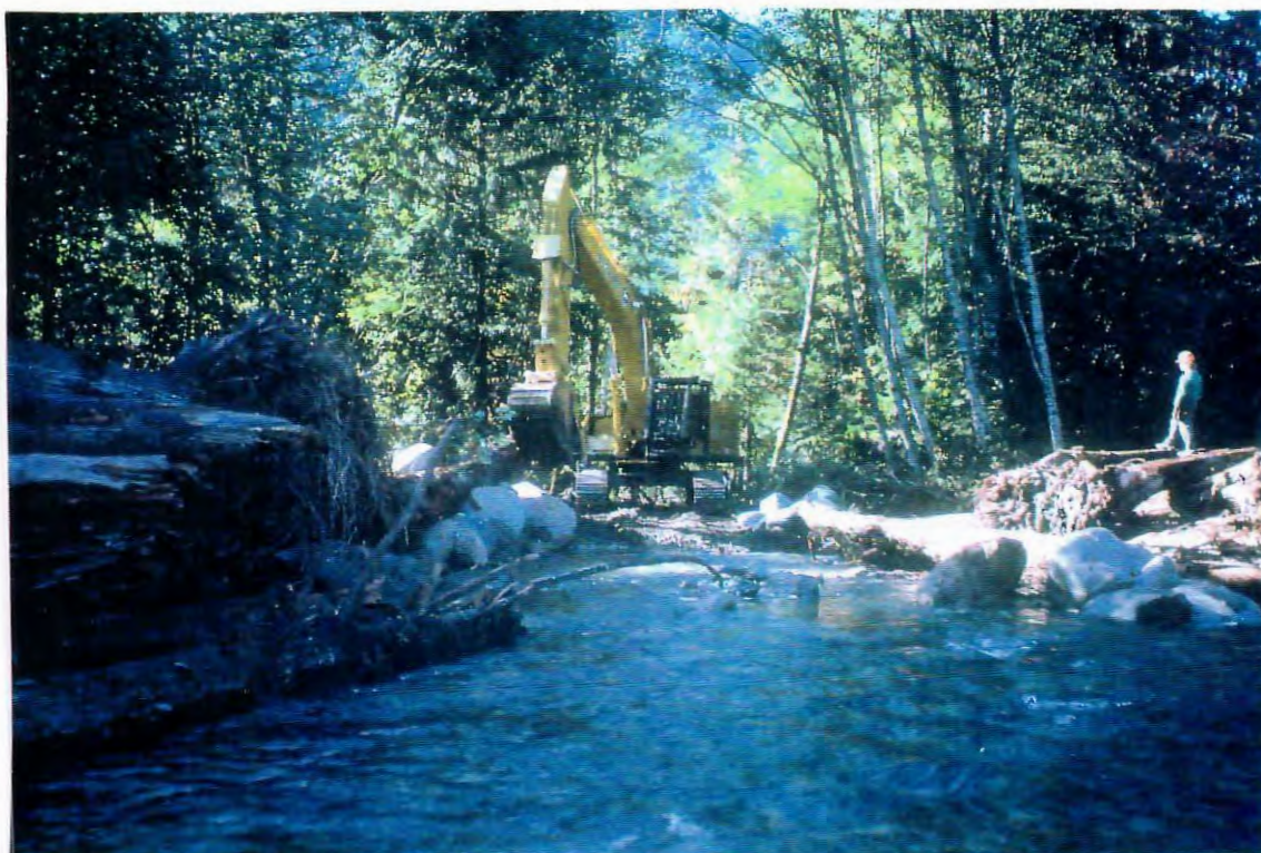
Photo 1. Coquihalla River jam construction.
