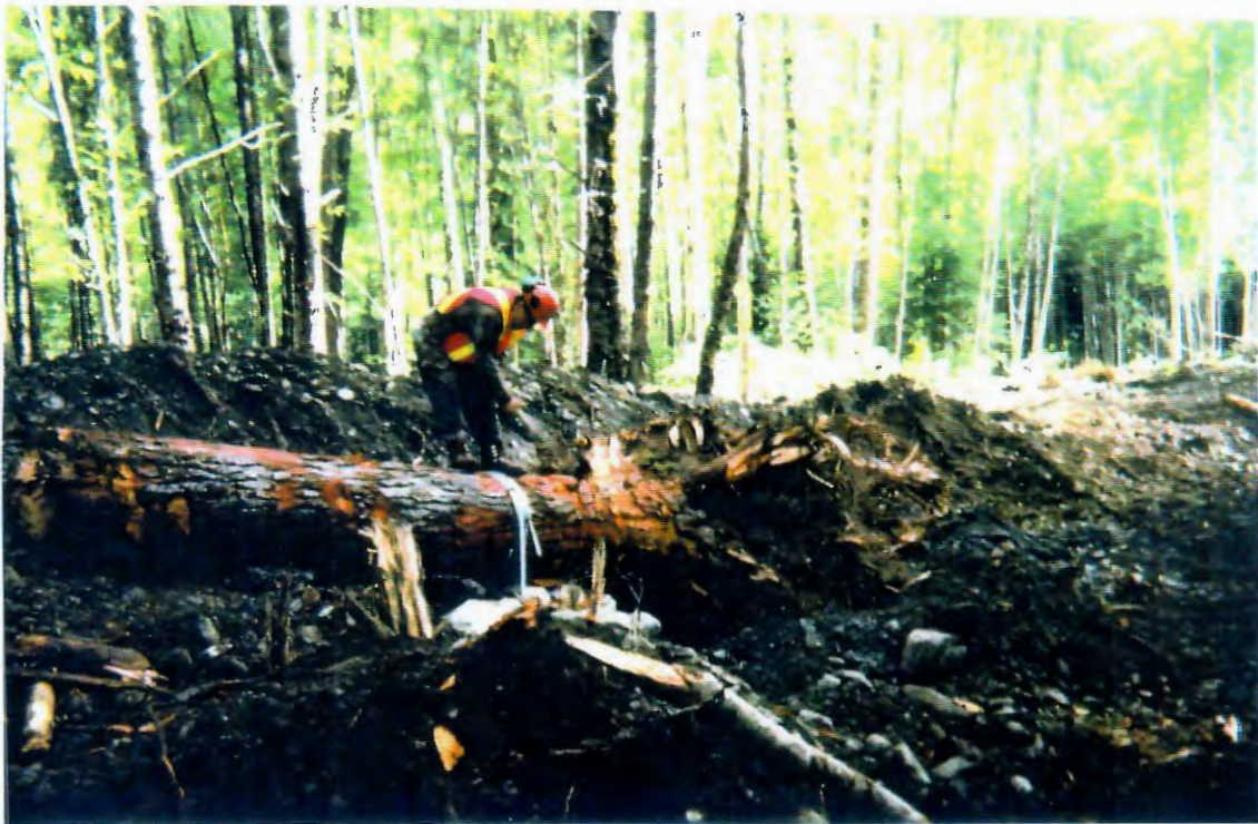
Photo 4. Cabling down large woody debris and rootwad to blocks.
