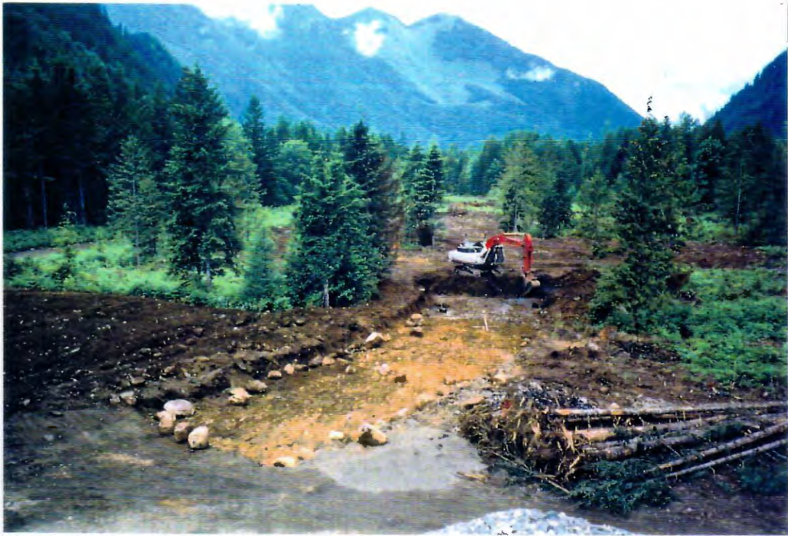
Photo 3. Excavation of channel.
