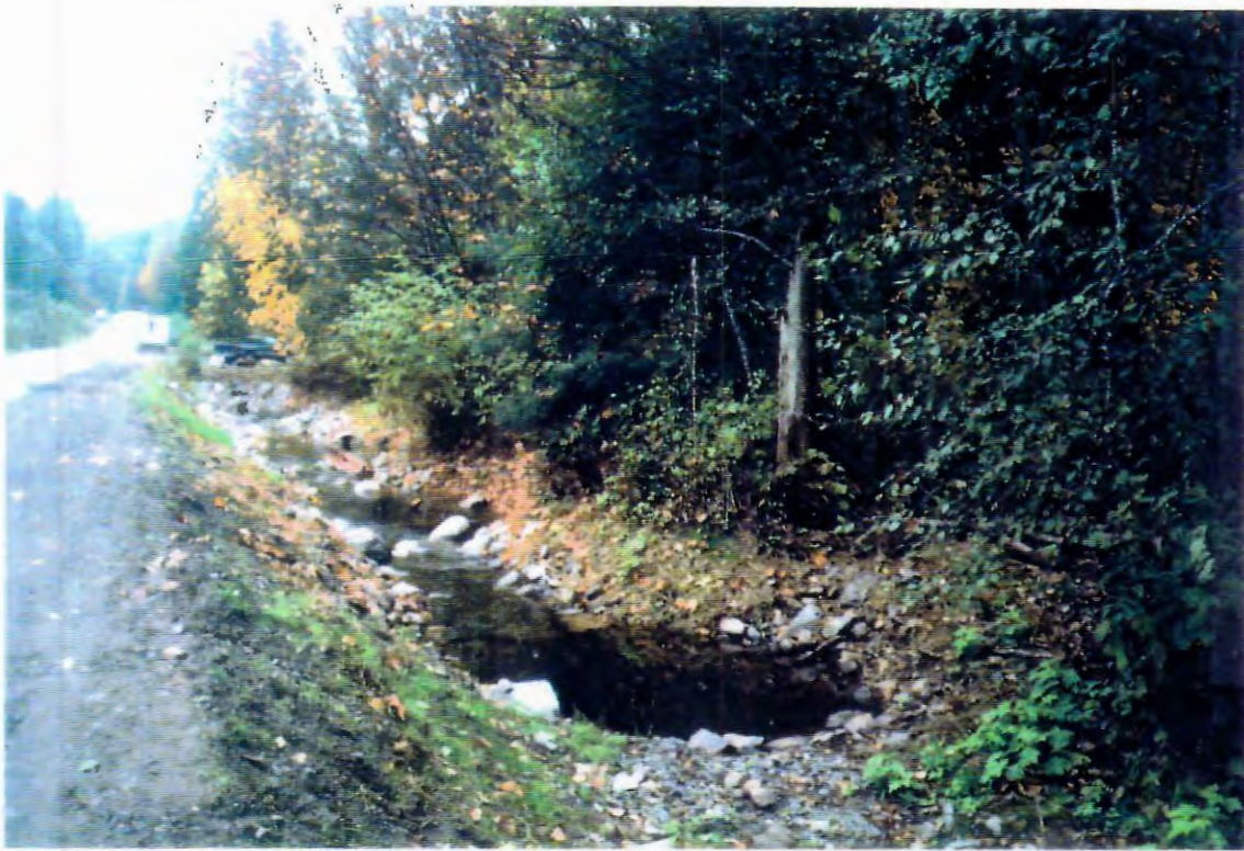
Photo 5. Downstream spawning and rearing channel below culvert.
