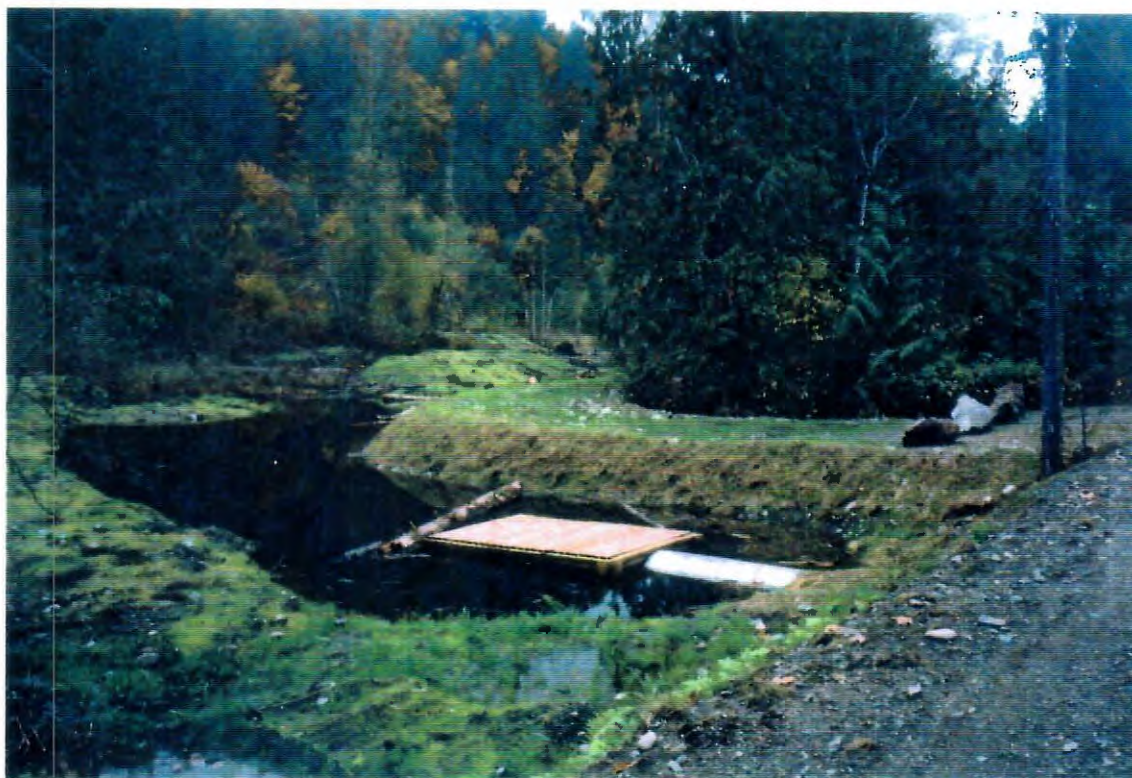
Photo 3. Flooded pond with beaver box and culvert at pond outlet.
