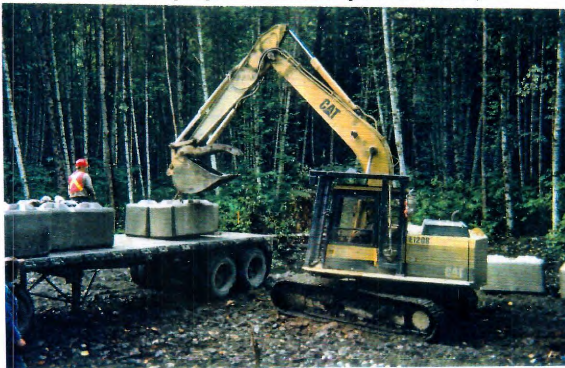
Photo 2. Anchor blocks for rootwad armouring.
