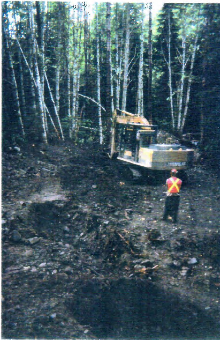
Photo 1. Preparing for bank stabilization (pits for anchor blocks).
