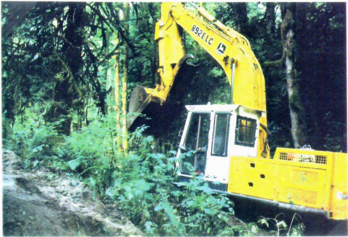
Photo 3. Excavation of overgrown channel.
