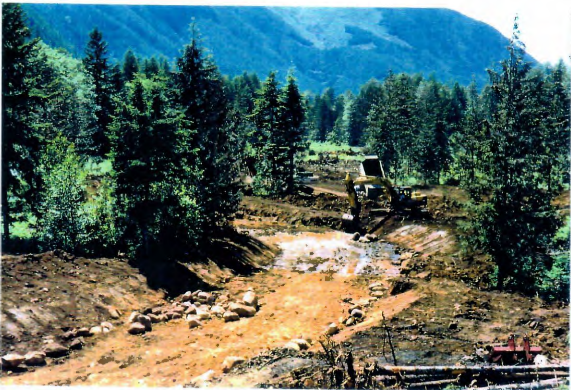
Photo 4. Sloping of channel.
