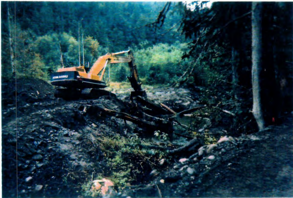
Photo 1. Excavation of deep channel along the side of the dyke in order to prevent beaver dam construction. Large woody debris was left in this channel for cover.
