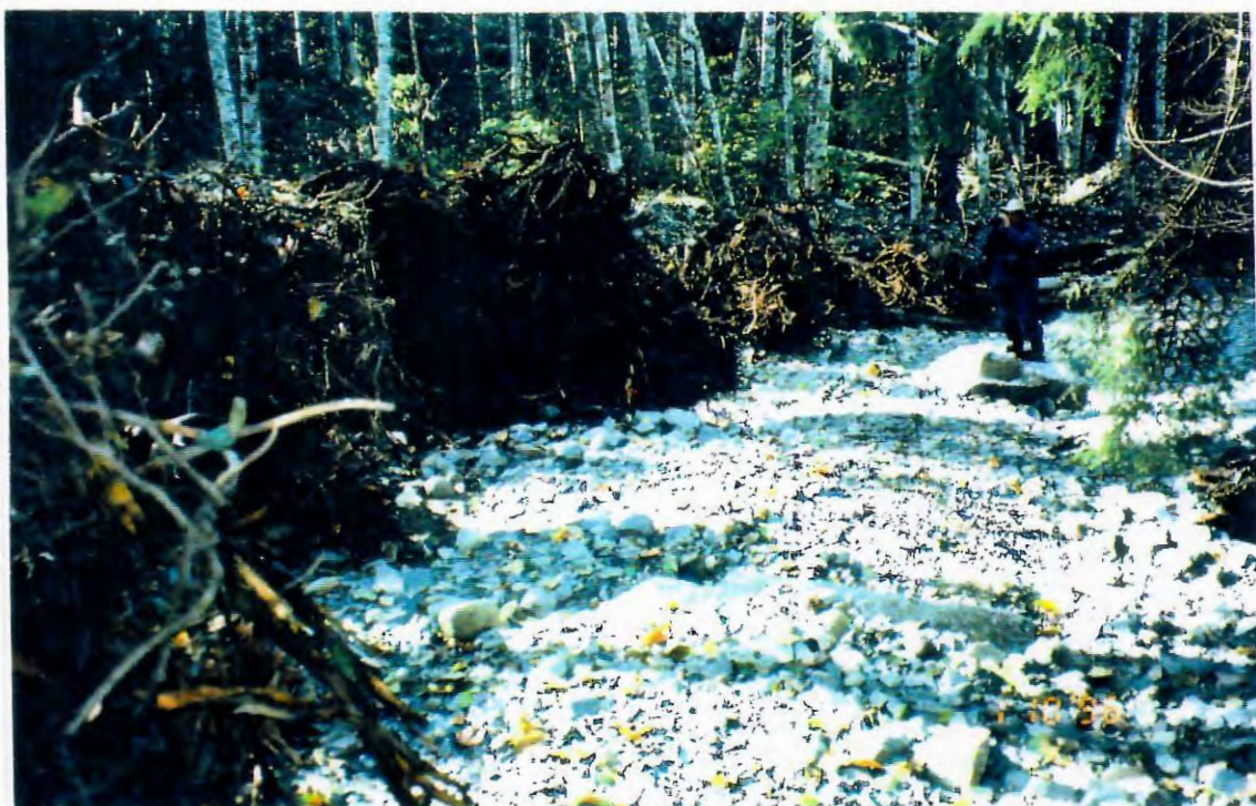
Photo 6. Final armoured bank constructed during low flows.
