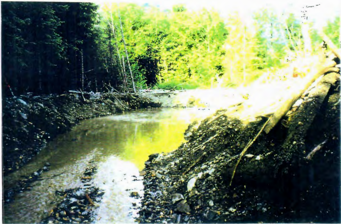
Photo 1. Instream construction of new channel between Cross-section 5 and Cross-section 7 viewed downstream from Cross-section 4. Excavation began at Cross-section 2 and worked downstream towards Cross-section 7.
