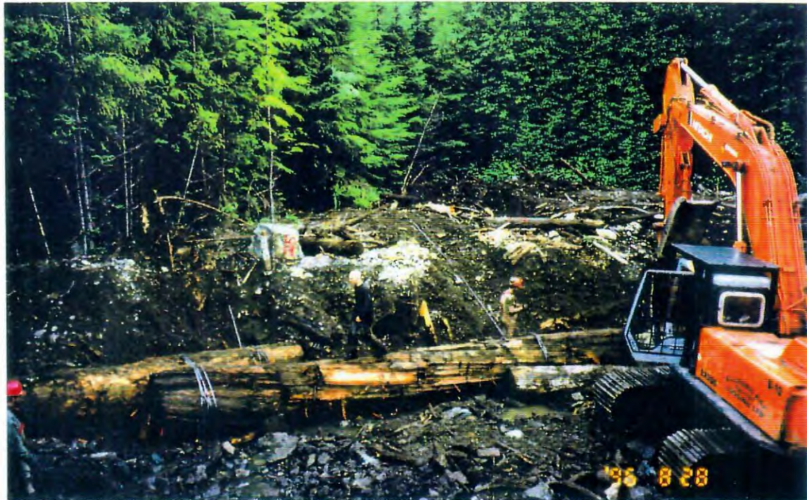
Photo 4. Construction of log bank protection at Bend 4 viewed from right bank. Logs are cabled together and have been anchored to anchor rocks buried at the base of the adjacent slope (note cables extending into the bush).
