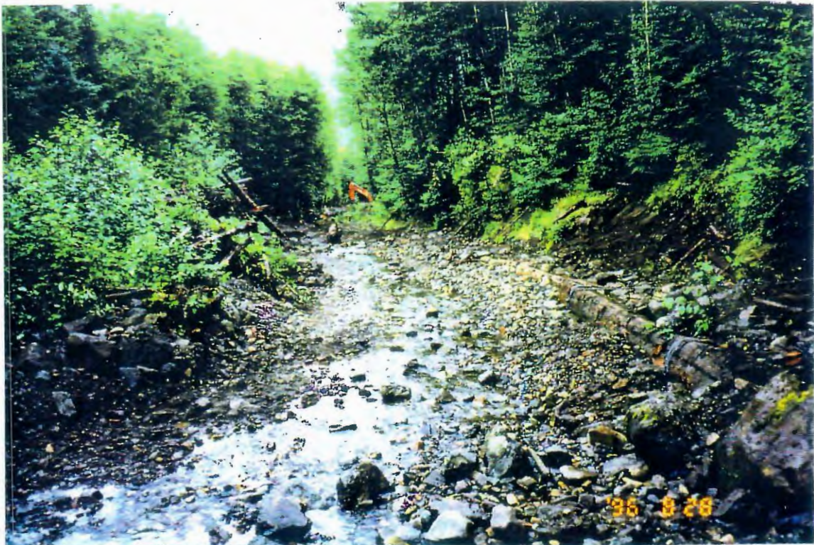
Photo 6. Completed instream work showing downstream view of log bank protection at Bend 1.
