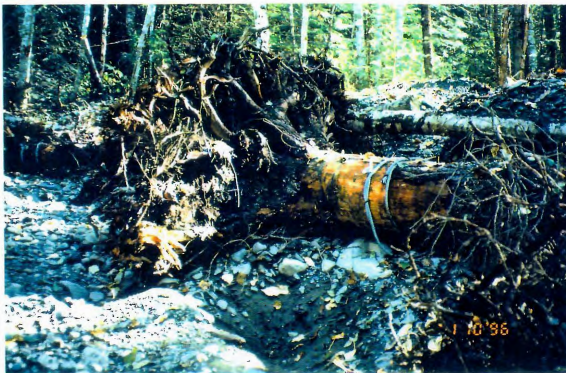
Photo 5. Backfill over tree stem and anchor block.
