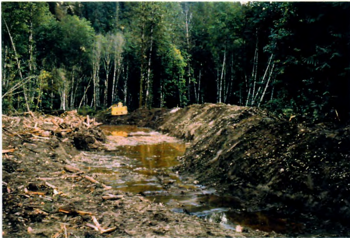
Photo 1. A dam under construction to create a large pond to provide winter refuge habitat.
