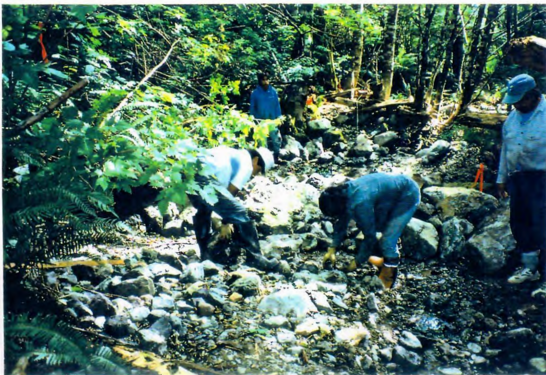
Photo 3. Channel restoration using hand labour and chainsaw winch.
