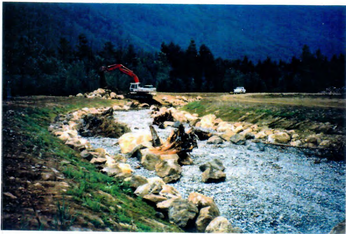
Photo 6. Gravel placement and channel complexing.
