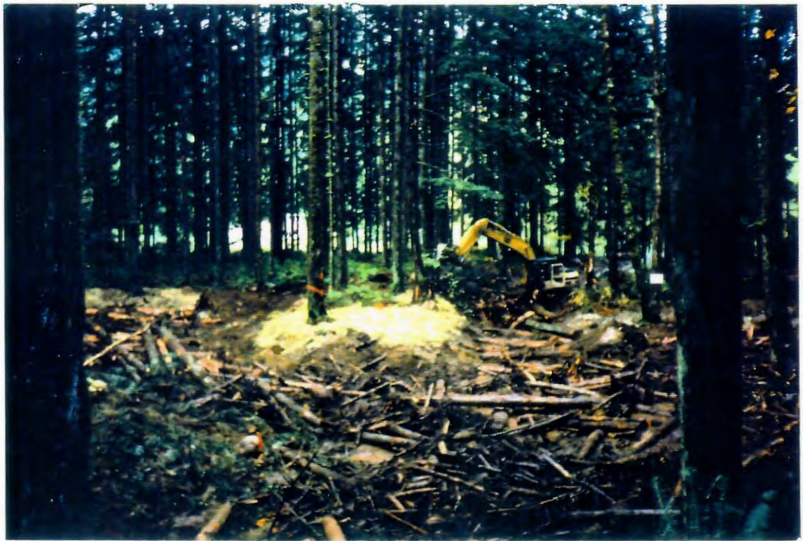
Photo 7 Excavator piling cleared debris (logs, stumps, etc.) into impoundment which will become pond.
