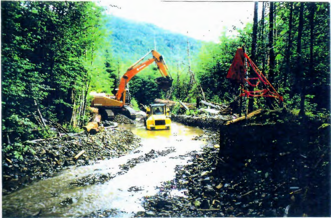
Photo 1. Instream construction of new channel between Cross-section 5 and Cross-section 7 viewed downstream from Cross-section 4. Excavation began at Cross-section 2 and worked downstream towards Cross-section 7.
