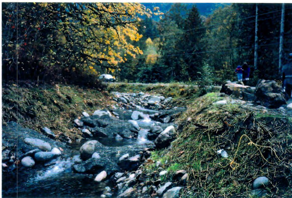
Photo 4. Fishway connecting downstream spawning channel to Chilliwack River.
