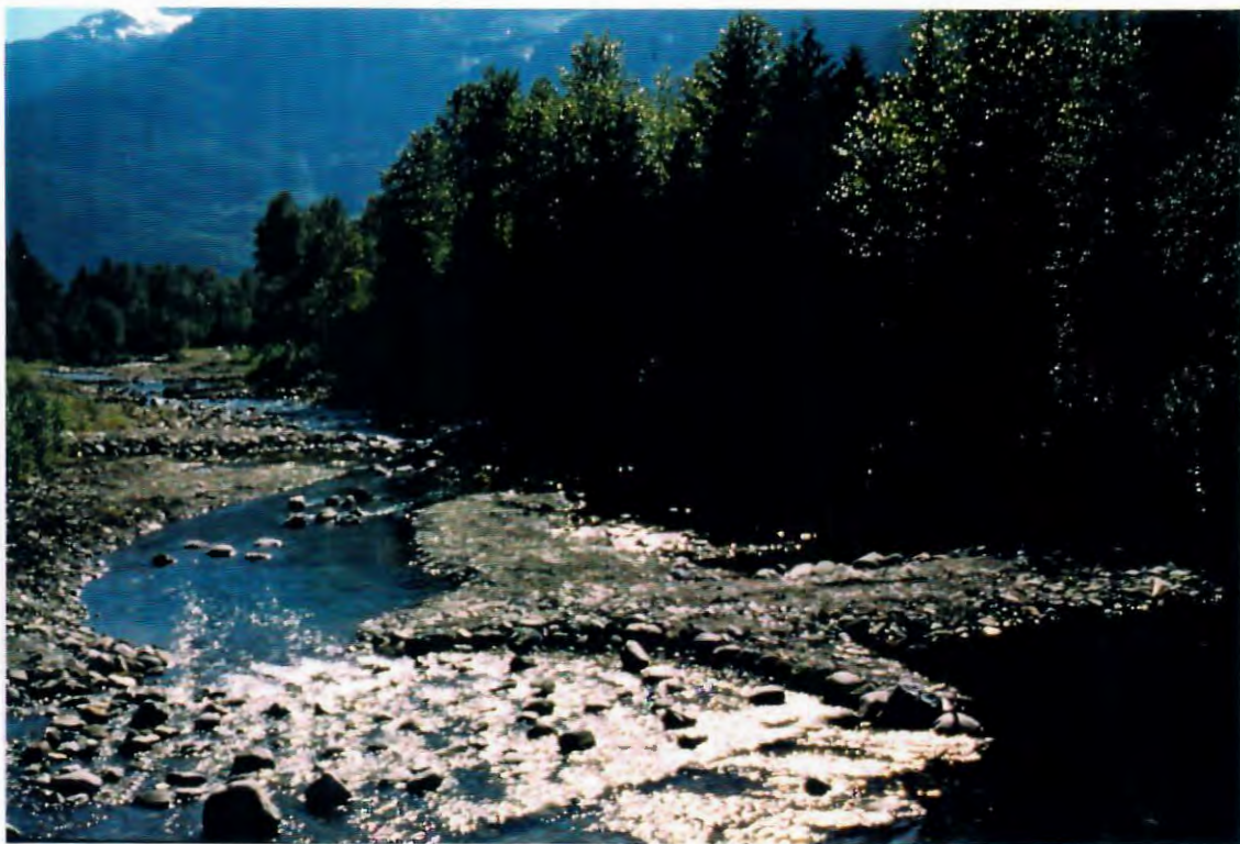
Photo 8. Six opposing wing deflectors were constructed to create deep pools and a meander pattern within the channel. During summer/fall 1996 chinook and chum salmon were seen spawning throughout this section of creek.
