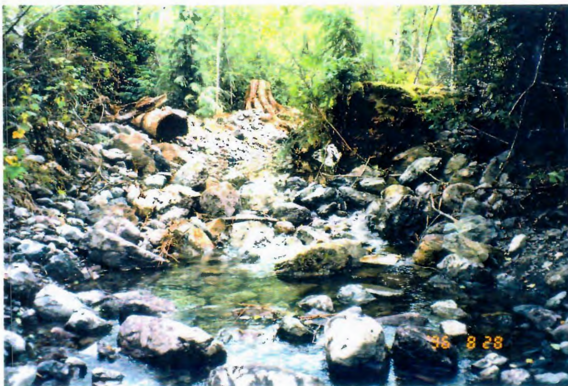
Photo 4. Trib. 1.37 after reconstruction.
