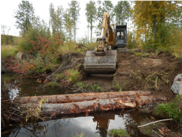
Photo 1. Bulkley River at Craker Rd (Lower) – Excavating the 3-log trench of the LWD structure at 0+000 m (26 September 2017).
