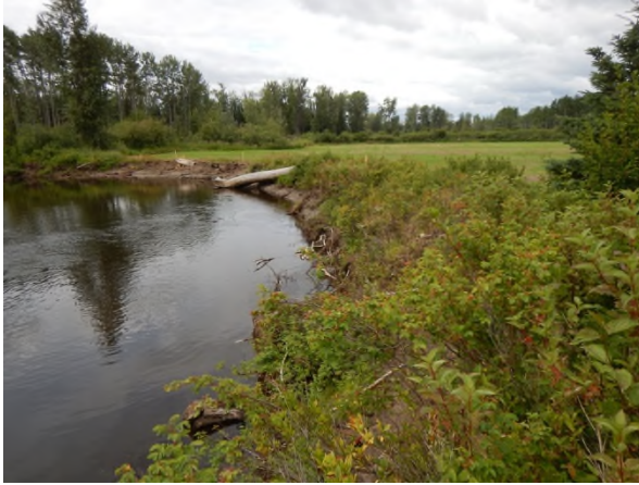
Photo 7. Bulkeley River at Craker Rd (Lower) – Looking downstream from 0+090 m prior to construction (23 July 2017).
