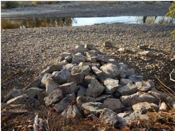
Photo 3. Bulkley River at Craker Rd (Lower) – View from the right bank of the rock groin at 0+105 m (3 October 2017).
