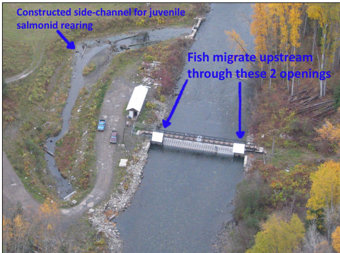
Photo 1: Aerial view of the KSEF, with the river flowing from the bottom to the top of the photo.
