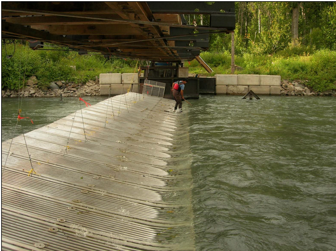
Photo 2: Looking at panels underneath the fence walkway. Cables on the left side of the photo are attached to the walkway by winches, which lower or raise the panels when needed.
