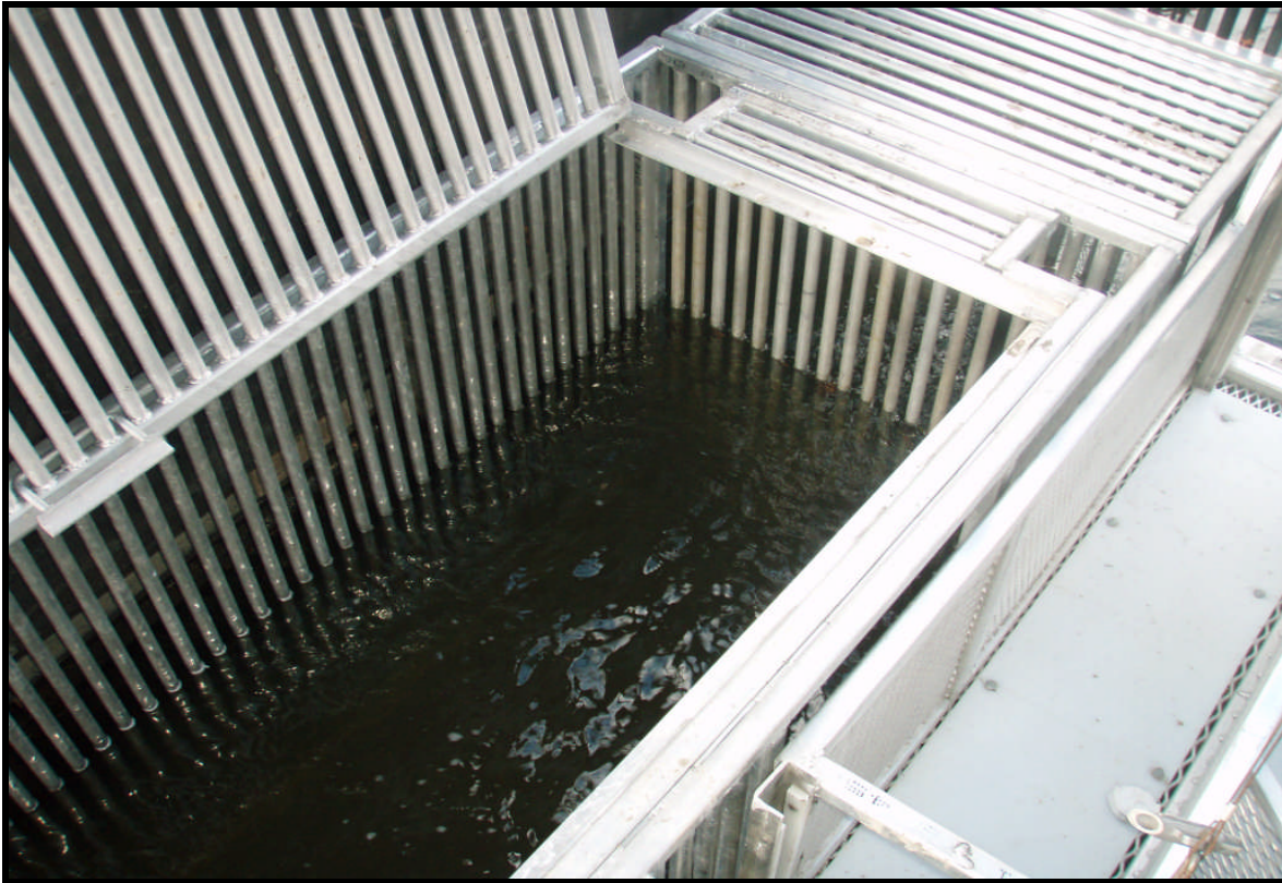
Photograph 5. Left bank holding bin.
