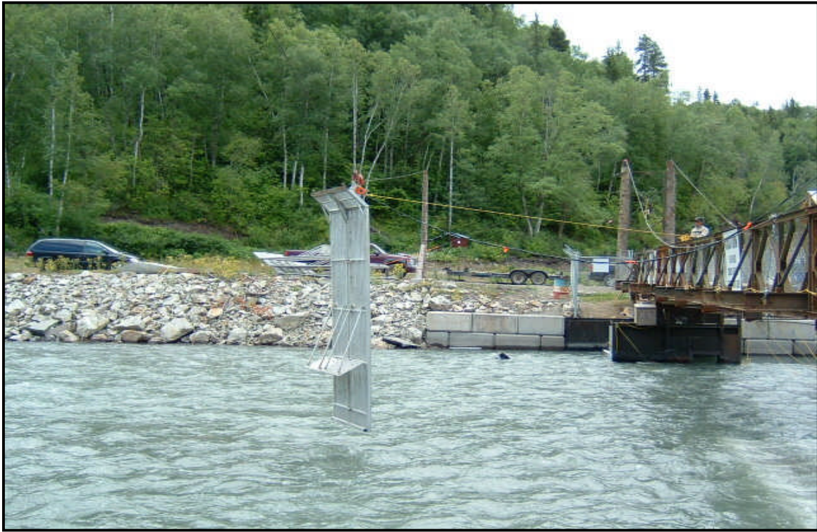
Photograph 3. Overhead winch used to raise and lower aluminium panels.
