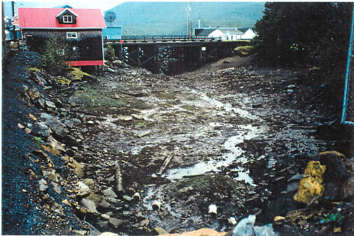
Cow Bay Slough at low tide. Note the log cribbing (upper photo) and gravel/vegetative bank (lower photo) which forms the northeast shoreline of the slough.
