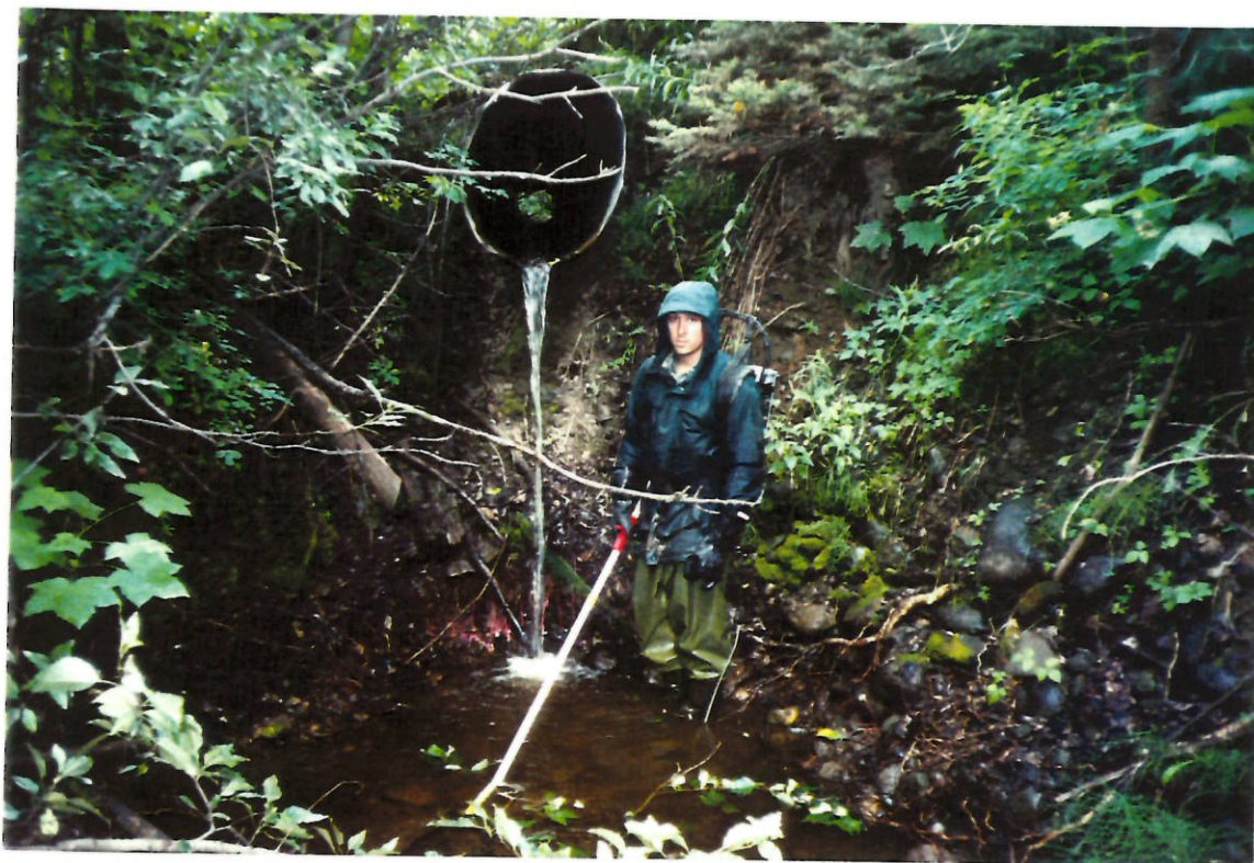
Photo #: 15 - 14 Site 163, upstream view of perched culvert 50 m upstream of Morice River.
