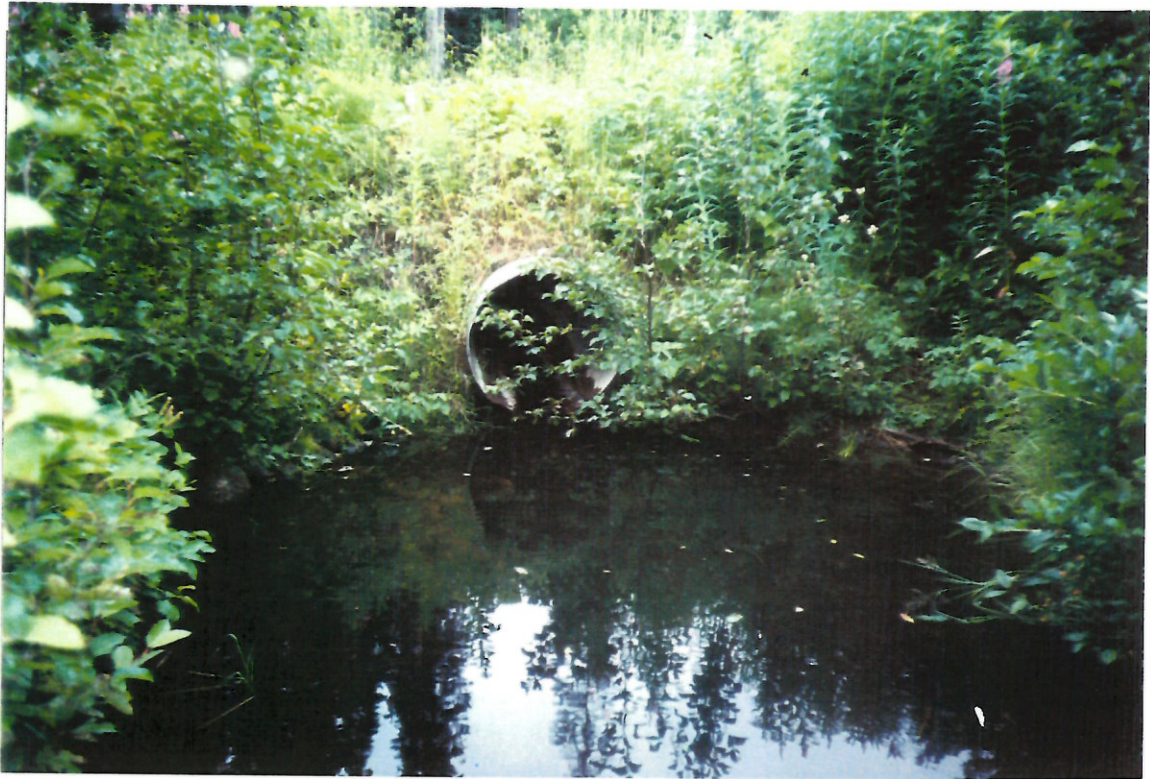
Photo #: 4 - 6 Site 340, looking upstream at culvert - well placed.
