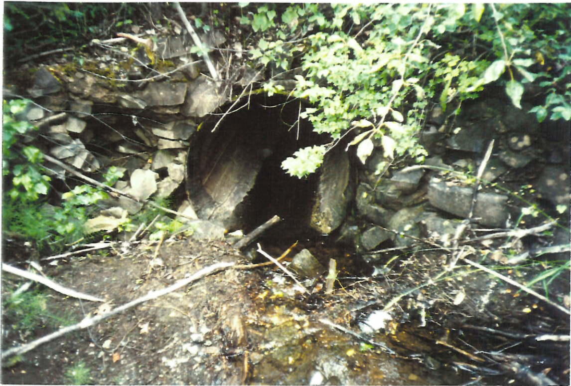
Photo #: 3 - 22 Site 332, looking downstream at wooden culvert.
