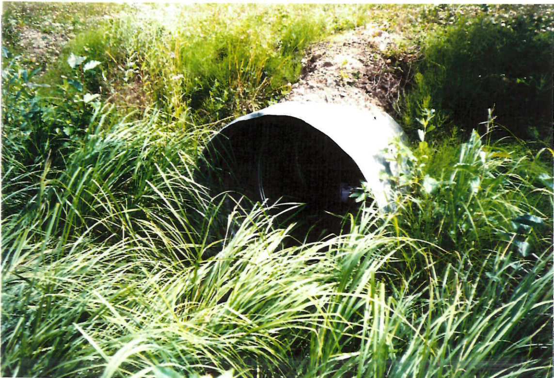
Photo #: 4 - 33 Site 349, looking downstream at lower culvert 1m inlet.
