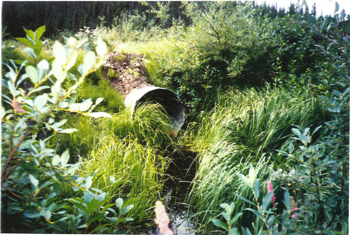
Photo #: 4 - 30 Site 349, looking upstream at culvert 1m upper road crossing.
