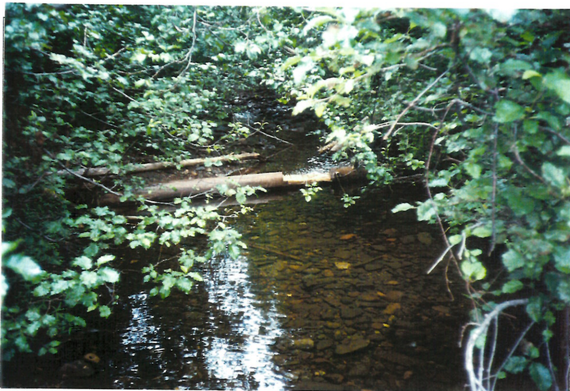
Photo #: 4 - 10 Site 341, looking upstream at WRP notched weir.
