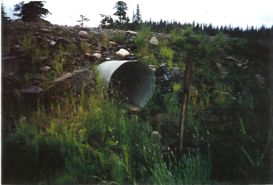
Photo #: 2 - 7 Site 312, looking upstream at a culvert crossing.
