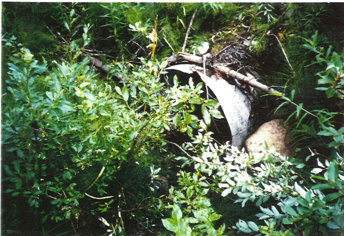
Photo #: 2 - 21 Site 317, looking downstream at culvert inlet (800 mm).
