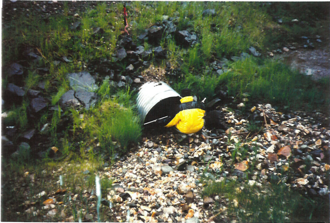
Photo #: 1 - 24 Site 309, culvert (1000m) well placed.
