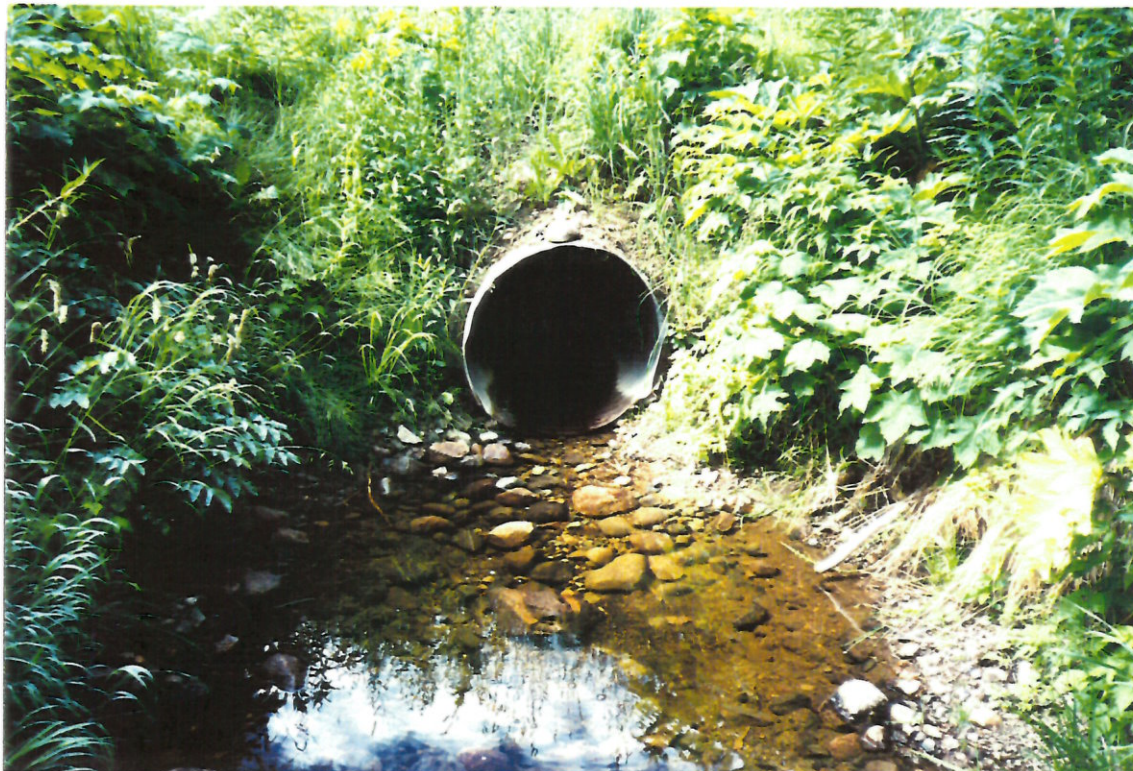
Photo #: 2 - 31 Site 320, looking upstream at well placed culvert (1000m).
