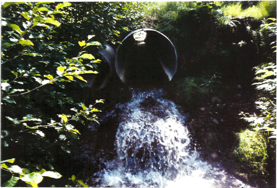
Photo #: 2 - 30 Site 319, looking upstream at barrier to u/s fish migration (1m CV).
