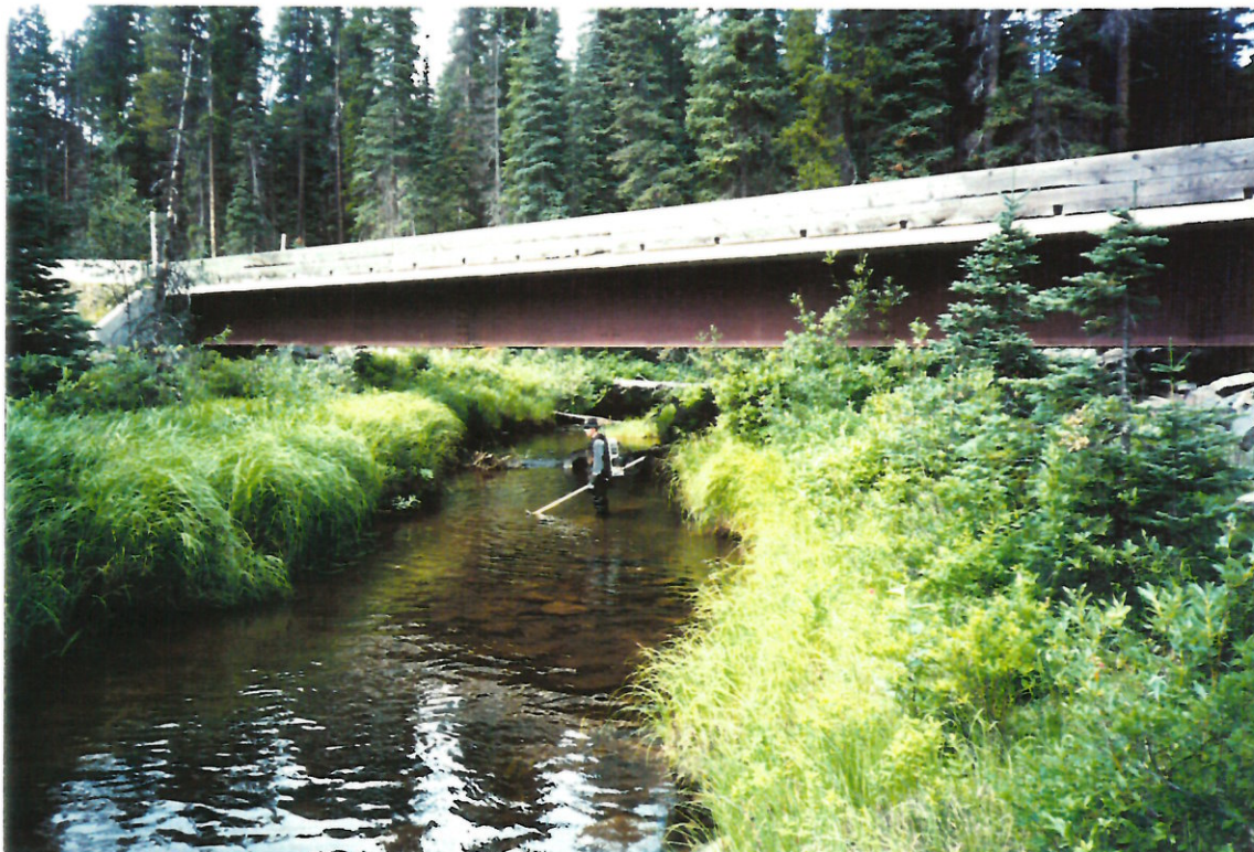
Photo #: 1 - 14 Site 305, looking upstream at bridge.
