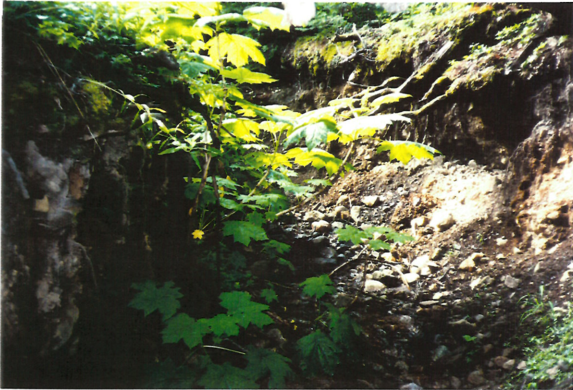
Photo #: 2 - 27 Site 319, looking upstream at entrenched, eroding banks.
