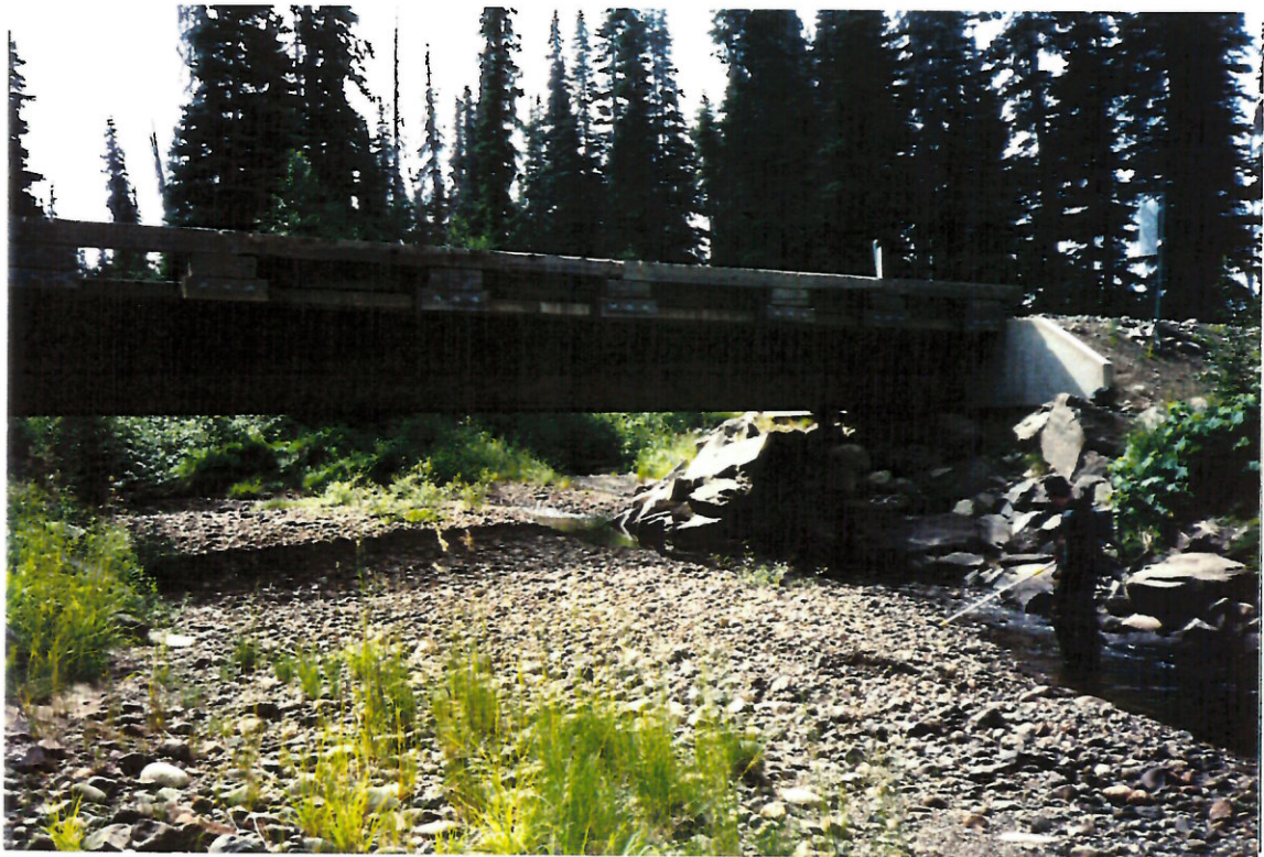
Photo #: 1 - 10 Site 304, looking upstream at full span bridge.
