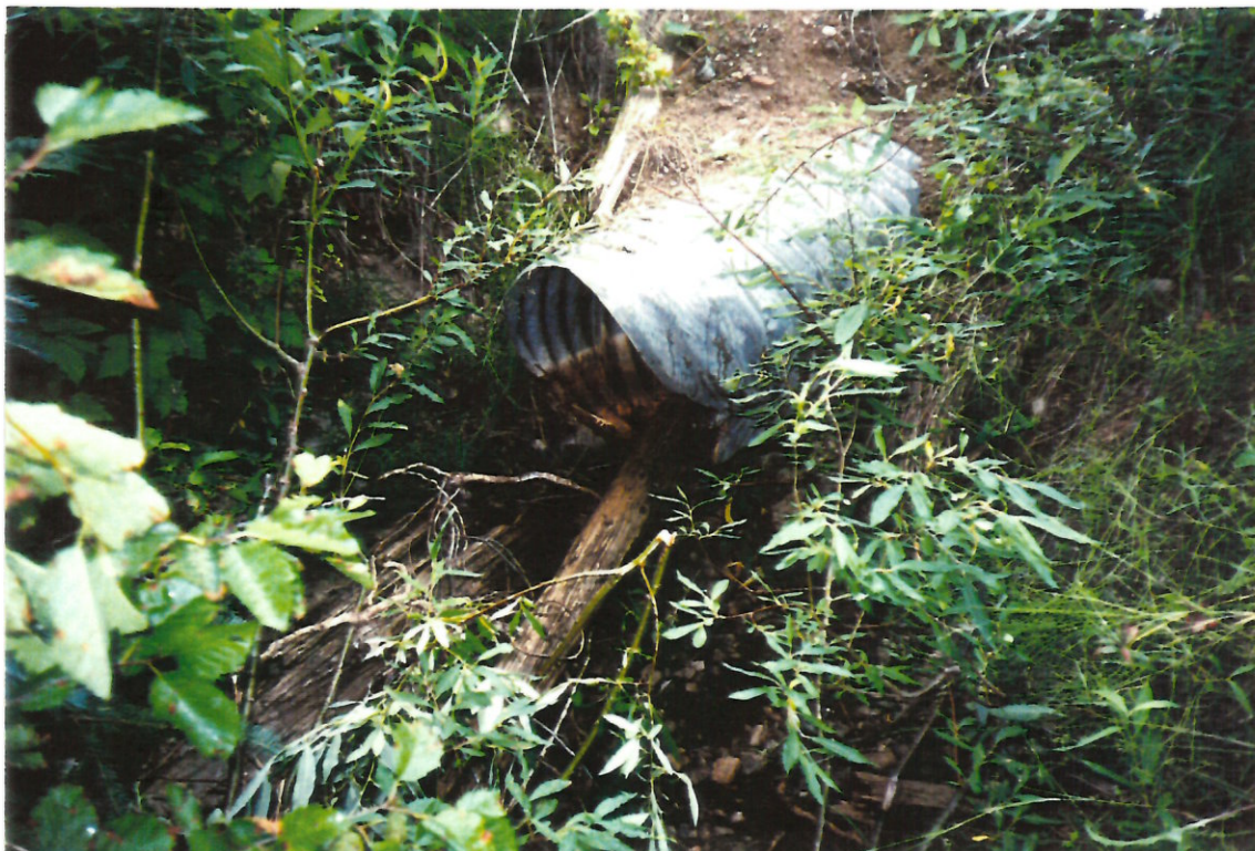
Photo #: 3 - 4 Site 325, looking upstream at a 600 mm culvert.
