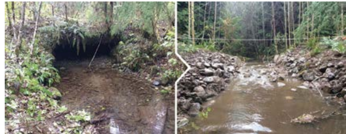
Before: Looking upstream toward the collapsed wood box culvert outlet
