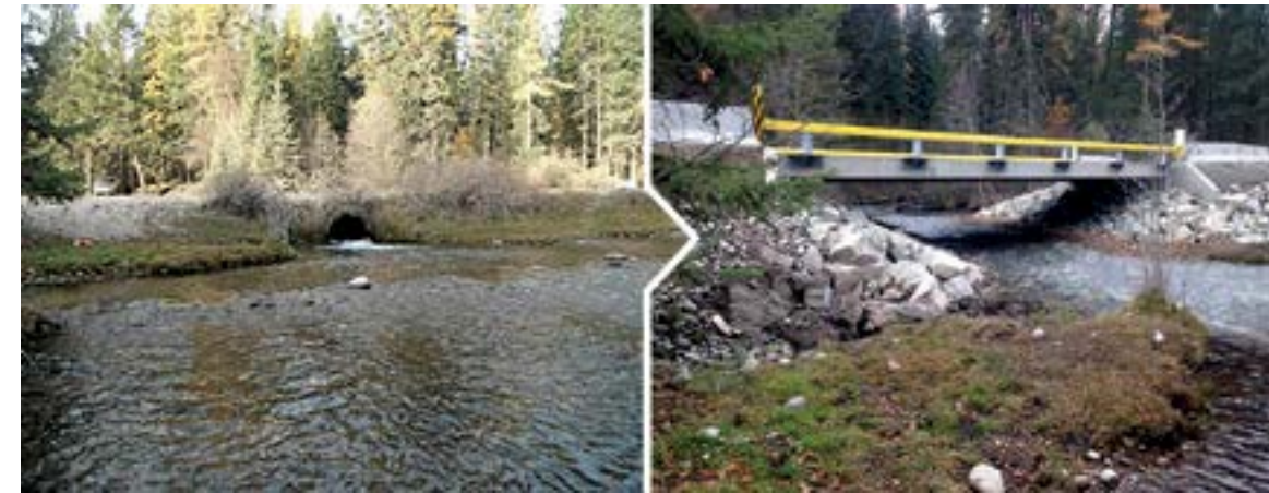
Plumbob Creek Crossing - before and after
