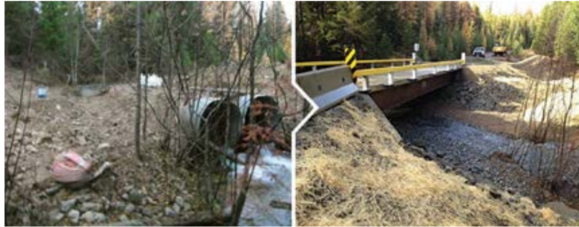
Purcell Creek Crossing – before and after
