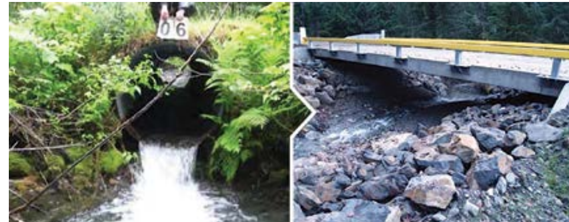
Before: Tributary to Cherry Creek crossing
