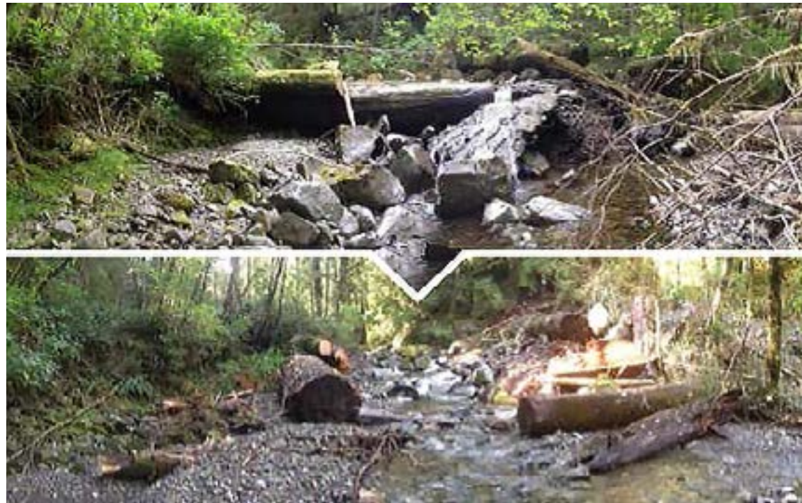
Upper photo: Clint Creek dam before the project
