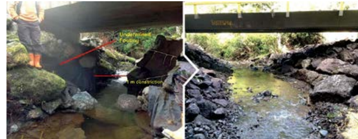
Before: Significant constriction of channel with large rip rap
