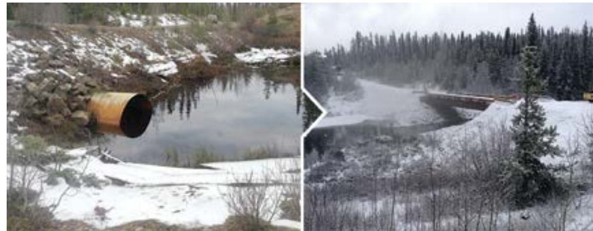
Before: Closed bottom structure that impeded fish passage that was removed
