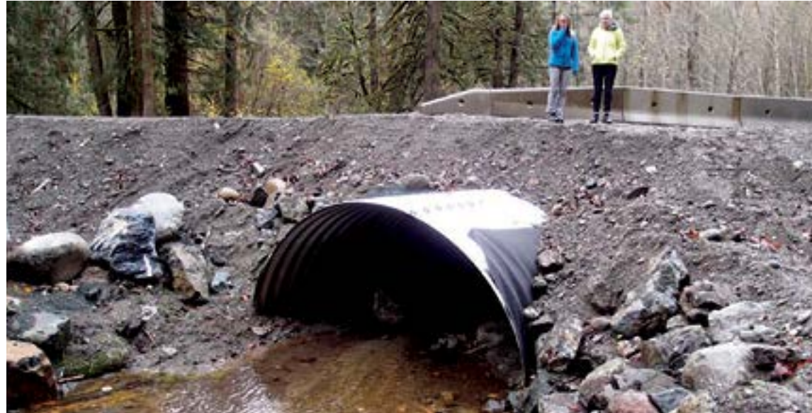
Newly installed open bottom arch culvert that provides for safe fish passage
