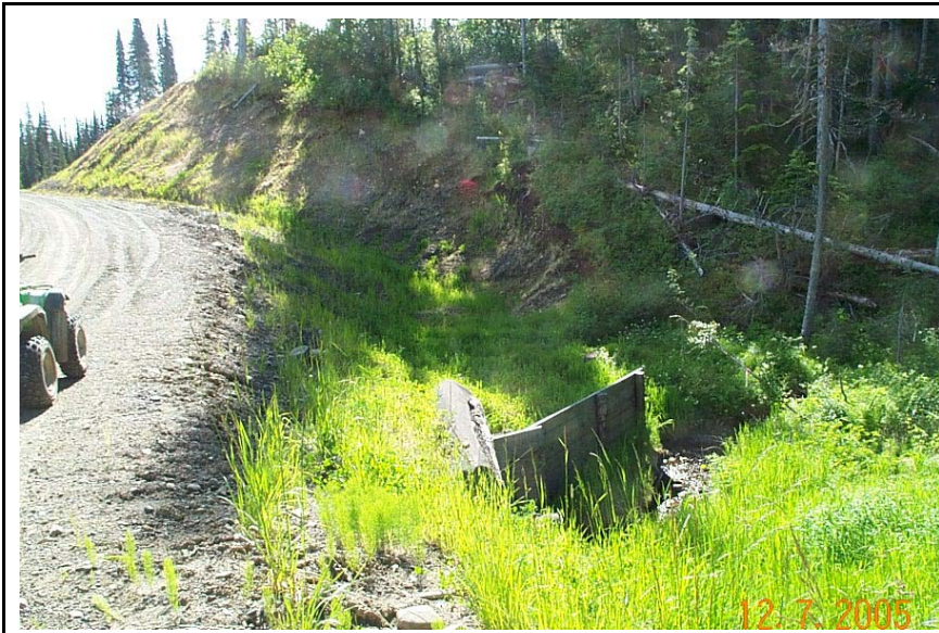
Figure 5. Crossing RC-15, cut-slope sediment source
