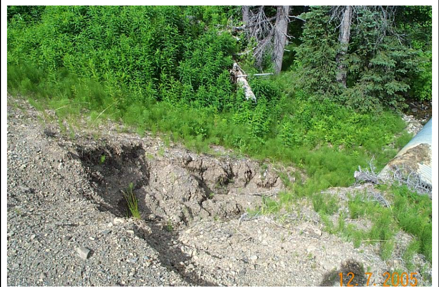
Figure 8. Crossing RC-21, small road failure directly into stream
