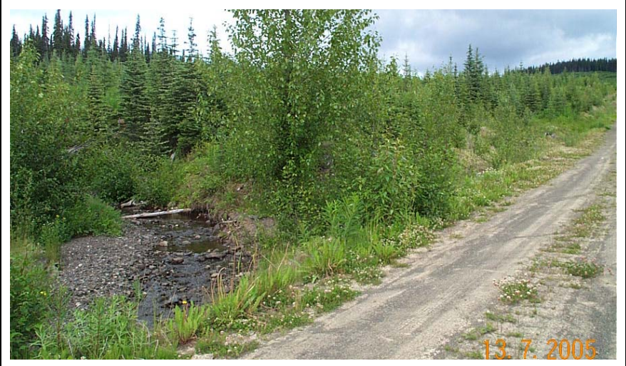
Figure 12. Crossing RC-40, sediment delivered from road and ditches surface
