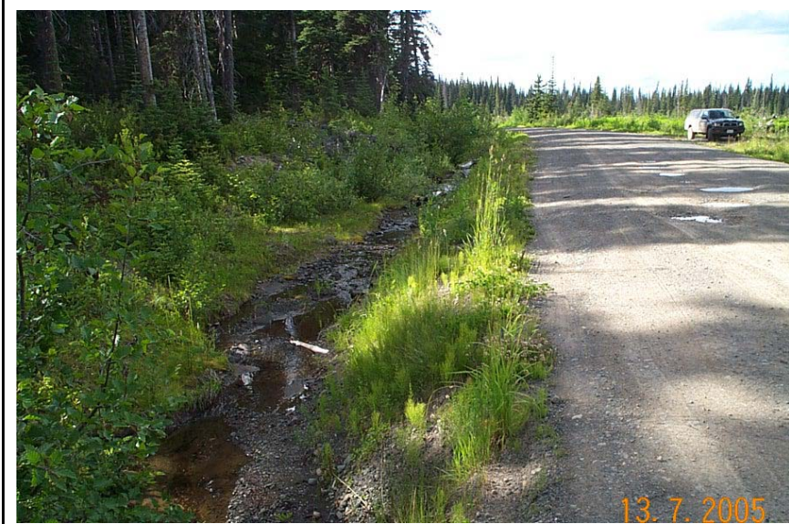
Figure 7. Crossing RC-42, Stream diverted down ditch
