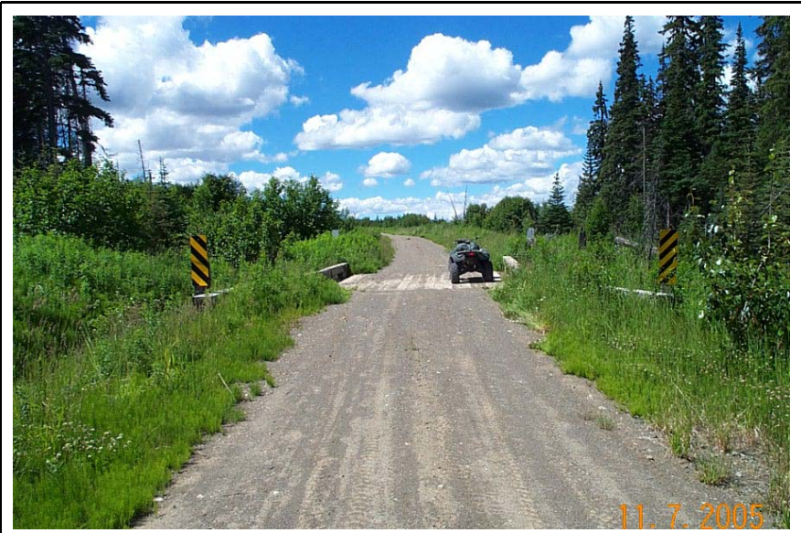
Figure 18. Crossing RC05, elevated bridge – no sediment delivery
