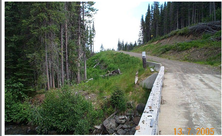
Figure 15. Crossing RE14, Some minor sediment is delivered to the stream from the road surface and onto the bridge deck and then into stream.
