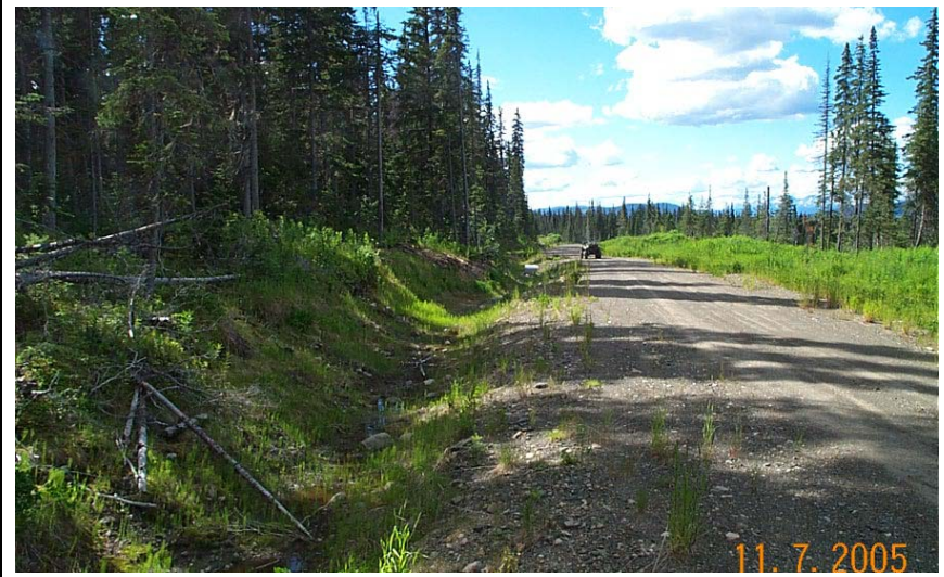
Figure 16. Crossing RC14, Some minor sediment is delivered from the road and down the ditch.
