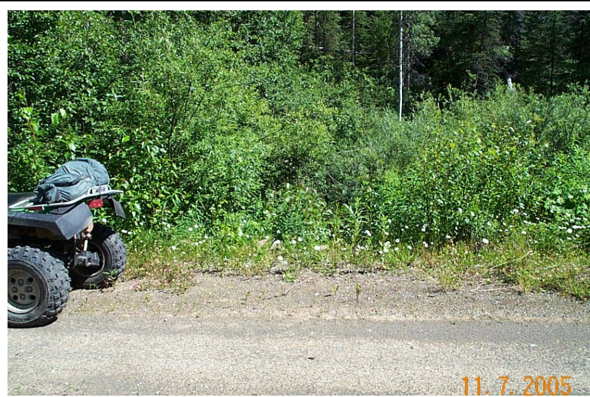
Figure 9. Crossing RC-02, some sediment is making it from the road surface to the stream
