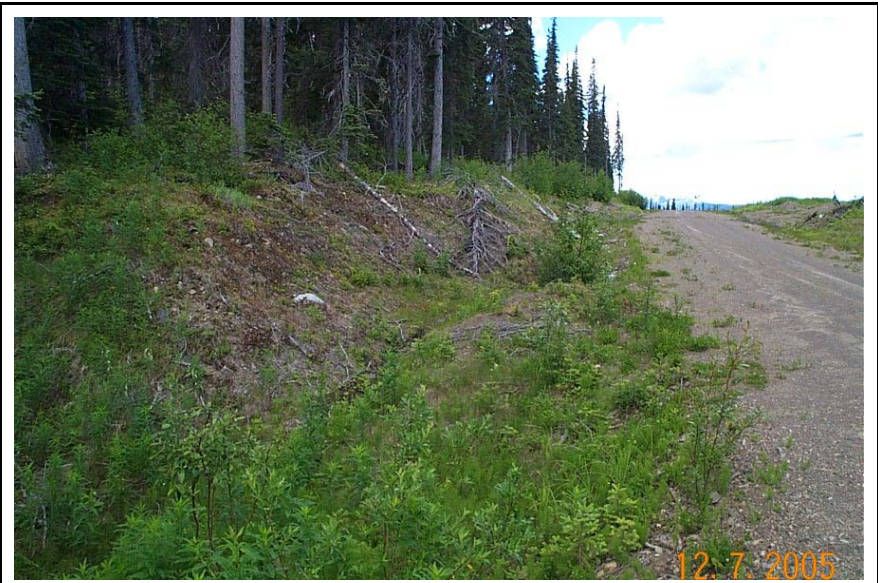
Figure 6. Crossing RC-16, slope/ditch sediment source
