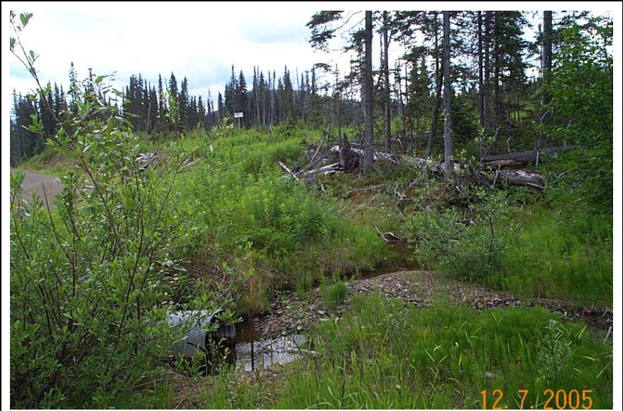
Figure 10. Crossing RC-17, Some sediment is still be eroded from the ditchline and transported to the stream.
