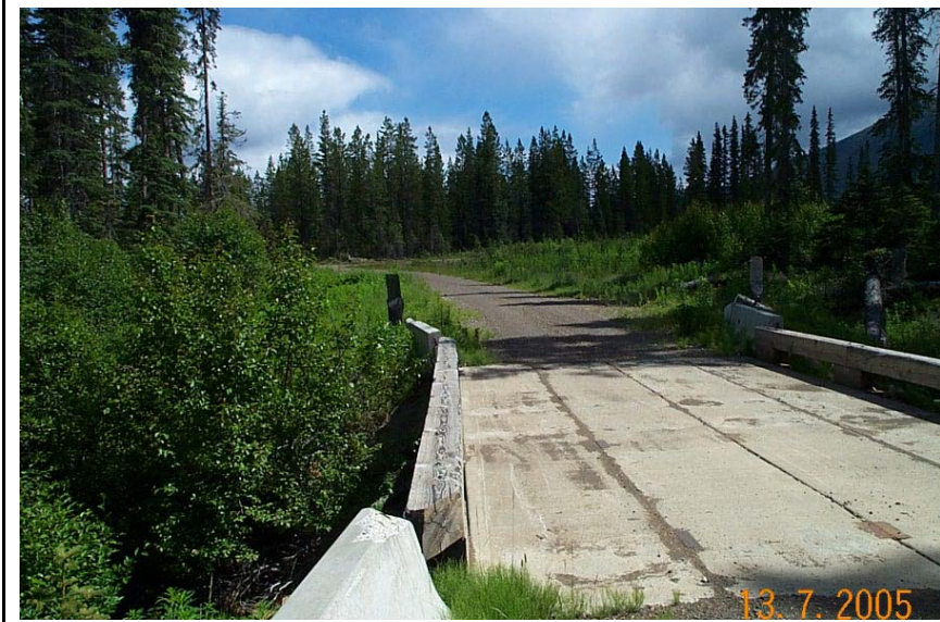
Figure 19. Crossing RC11, no sediment delivery issues identified
