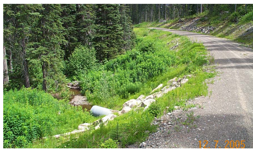
Figure 11. Crossing RC-19, sediment is being delivered from the road surface
