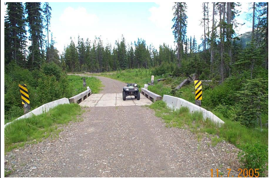
Figure 20. Crossing RC12, no sediment delivery issues identified
