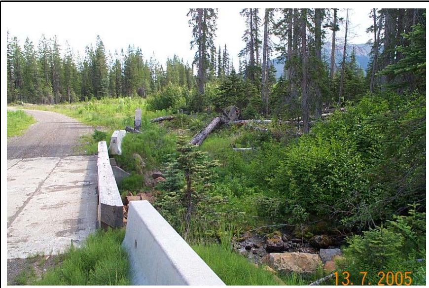
Figure 14. Crossing RE6, some minor sediment is delivered down the ditch
