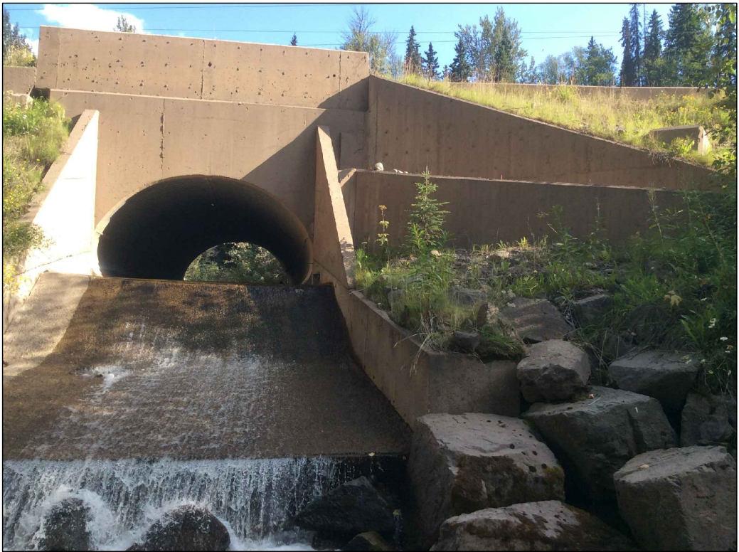
PHOTO #4 - VIEW OF CULVERT OUTLET
