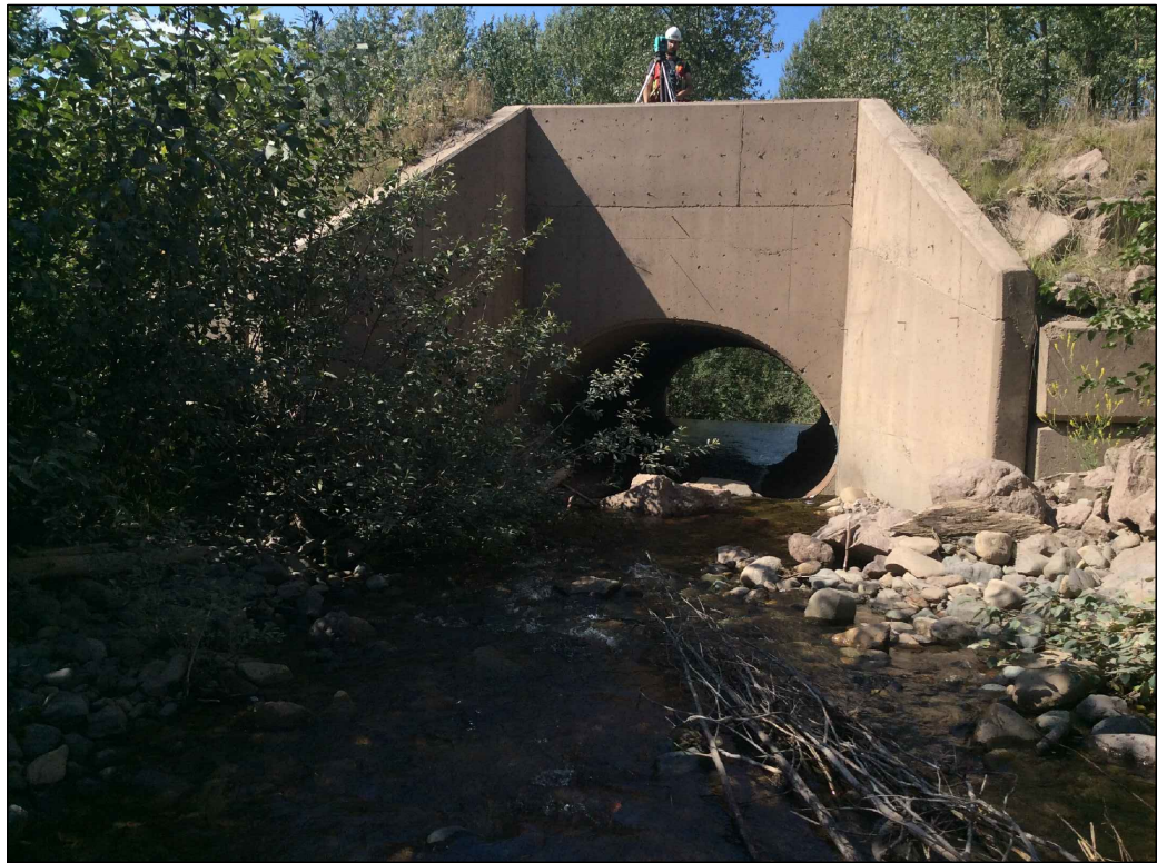
PHOTO #3 - VIEW OF CULVERT INLET
