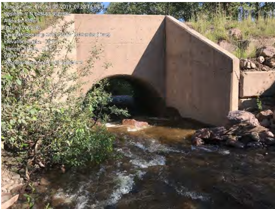
Photo 2. Culvert inlet and concrete headwall at Peacock Creek.
