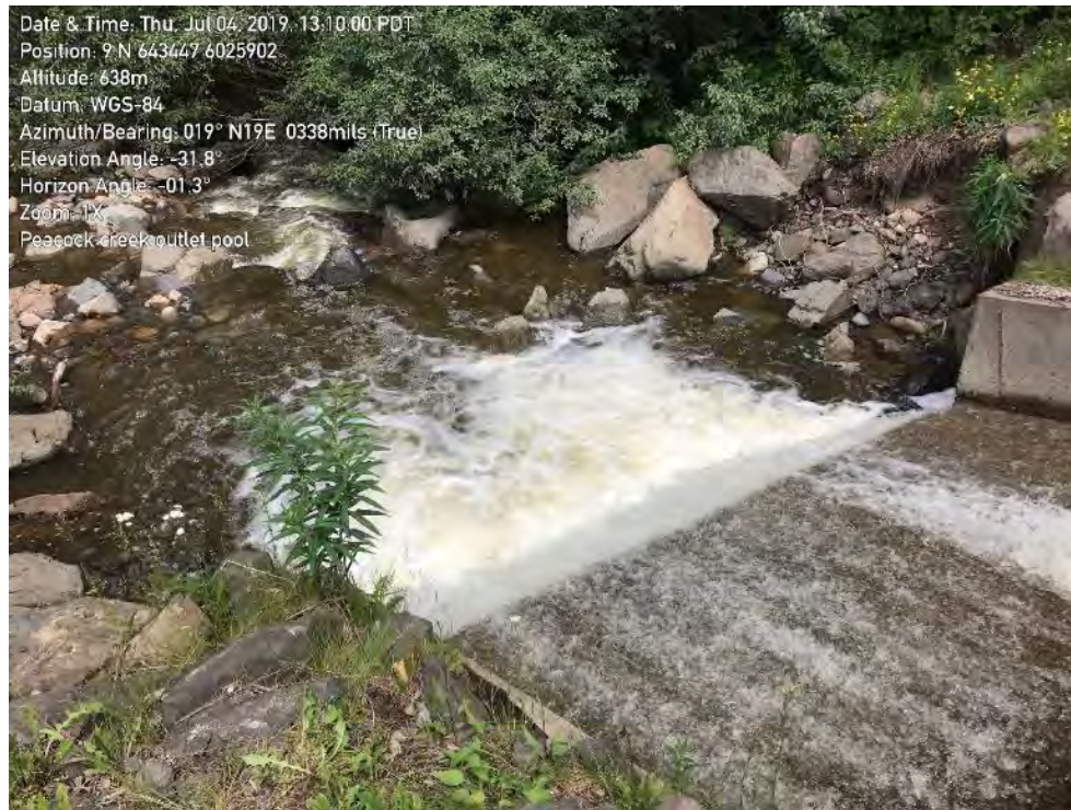
Photo 5. Looking downstream from the spillway towards the plunge pool.
