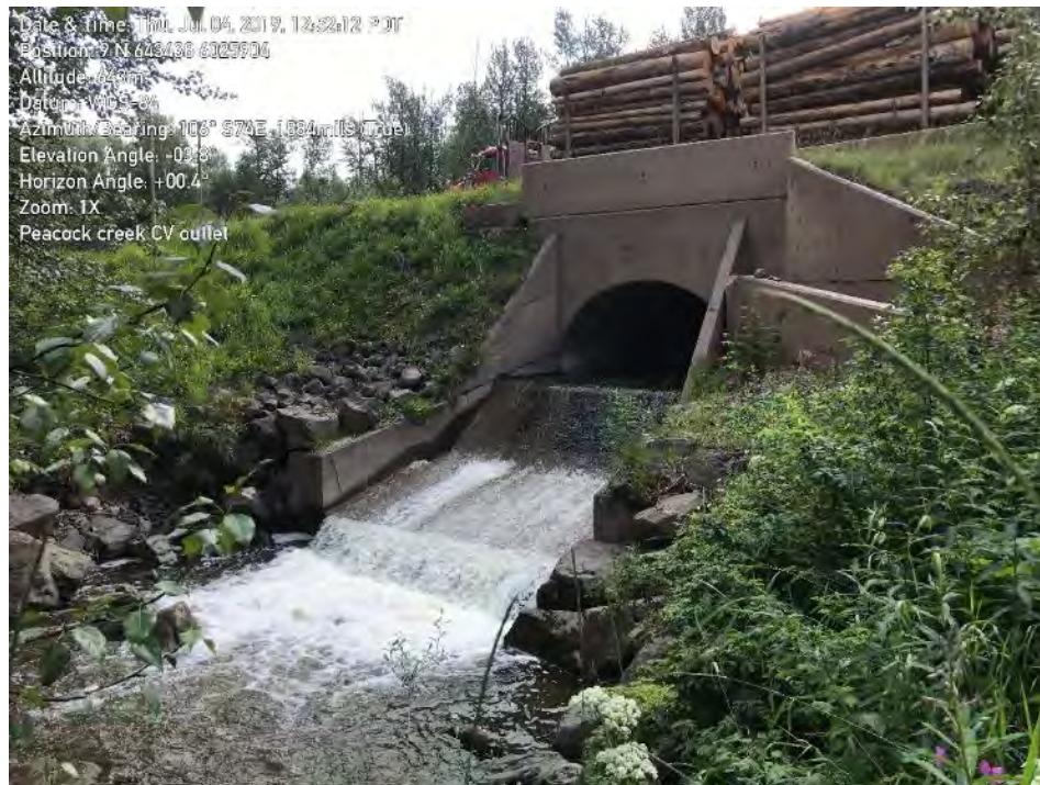
Photo 1. Peacock Creek CSP outlet and spillway.
