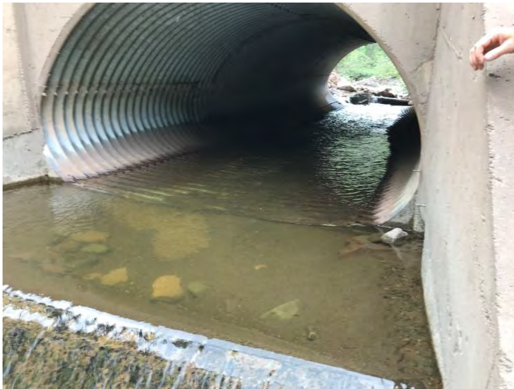
Photo 6. View through the culvert, looking from the outlet towards the inlet.
