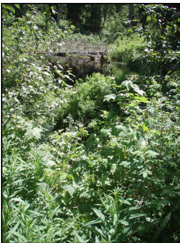
Figure 42. Site 240 culvert inlet. View upstream from inlet.
