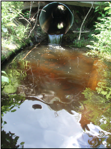
Figure 49. Site 239 culvert outlet. View upstream to outlet.
