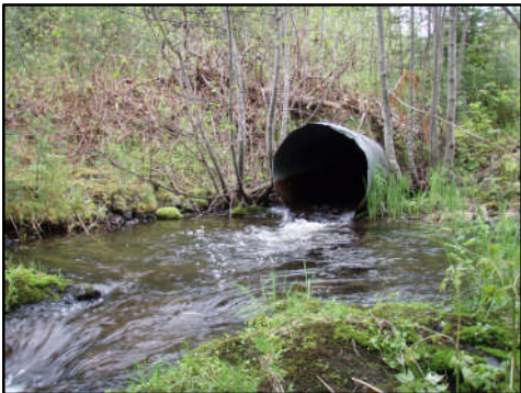
Figure 28. Hodder Creek culvert outlet. View upstream to outlet.
