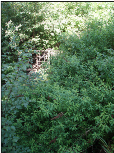
Figure 41. Site 240 culvert inlet. View downstream to inlet
