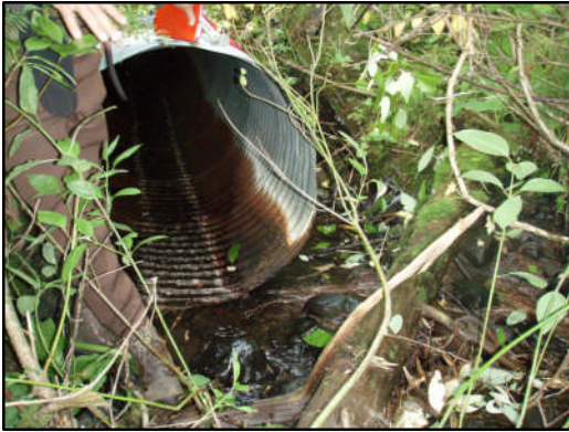
Figure 51. Site 390 culvert inlet. View downstream to inlet.
