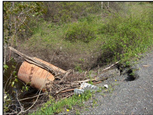
Figure 35. Kline Creek culvert inlet. View shows failure in road shoulder
