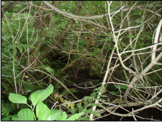
Figure 53. Site 390 culvert outlet. View downstream from outlet.
