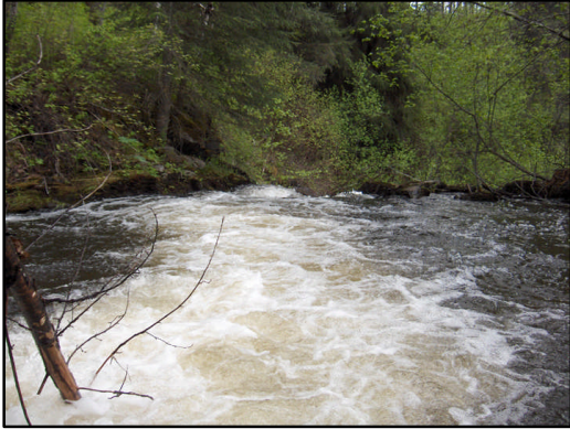
Figure 18. Skunsnat Creek culvert outlet. View downstream from outlet.
