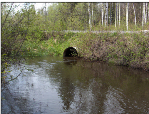
Figure 31. Kline Creek culvert outlet. View upstream to outlet.
