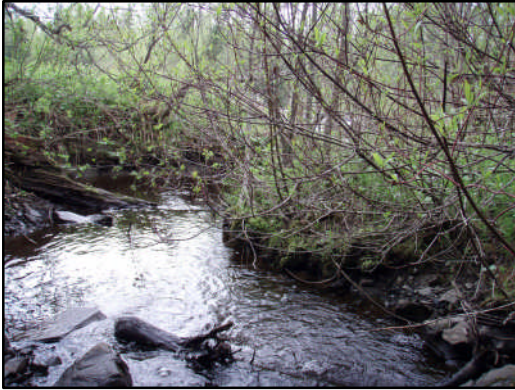
Figure 37. Site 74 culvert outlet. View downstream from culvert.
