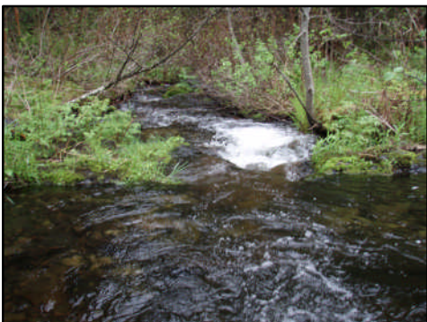
Figure 29. Hodder Creek culvert outlet. View downstream from outlet.
