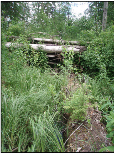
Figure 46. Site 239 culvert inlet. View downstream to inlet.
