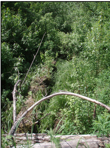
Figure 47. Site 239 culvert inlet. View upstream from inlet.
