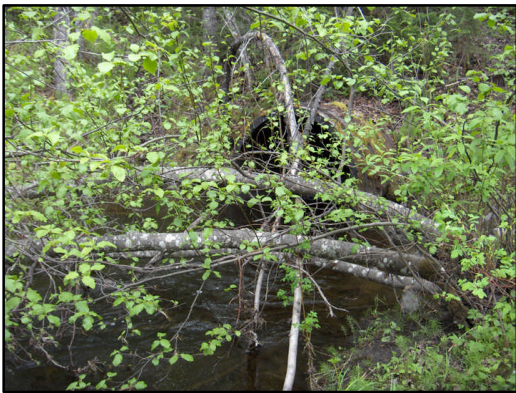
Figure 20. Skunsnat Creek inlet. View downstream to inlet.
