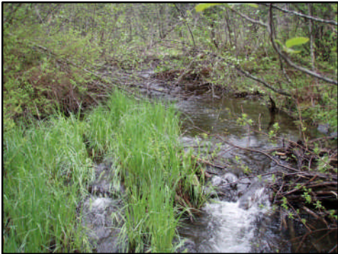
Figure 27. Hodder Creek culvert inlet. View upstream from inlet.
