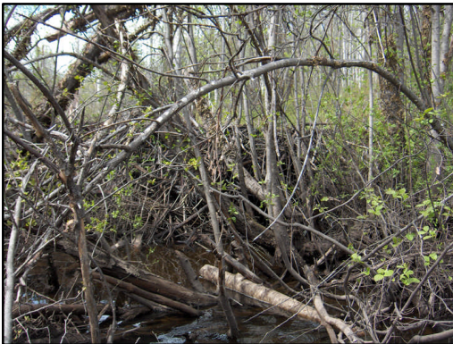
Figure 34. Kline Creek culvert inlet. View to beaver dam 29 m upstream.
