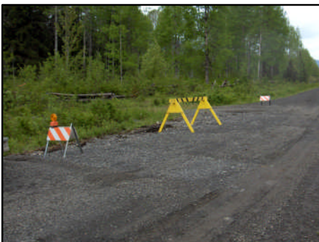
Figure 36. Kline Creek View shows erosion where Kline flowed over Kispiox Trail
