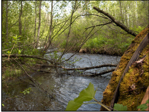
12. Clifford Creek culvert inlet View upstream from inlet.
