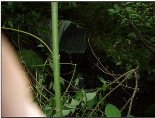
Figure 54. Site 390 culvert outlet. View upstream to outlet.
