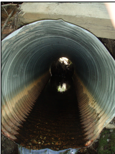
Figure 50. Site 239 culvert. View upstream through culvert.
