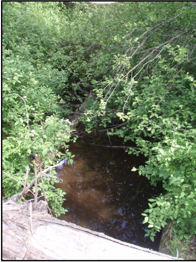
Figure 48. Site 239 culvert outlet. View downstream from outlet.
