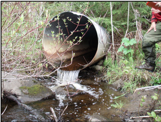
Figure 38 Site 74 culvert outlet. View upstream of outlet.
