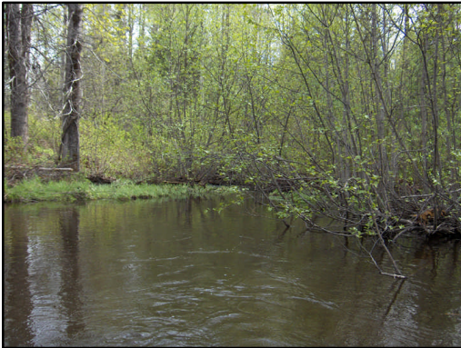
Figure 30. Kline Creek culvert outlet. View downstream from outlet.
