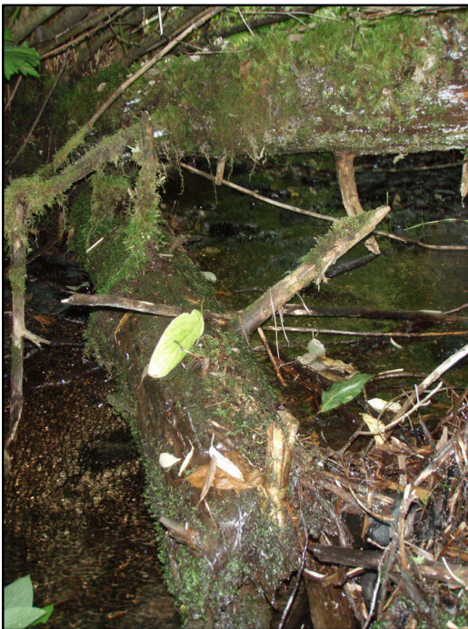
Figure 52. Site 390 culvert inlet. View upstream from inlet.
