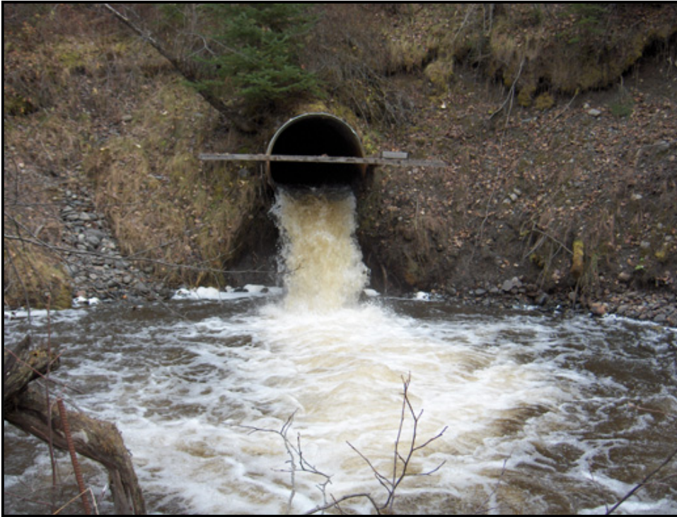
Station Creek: outlet upstream
