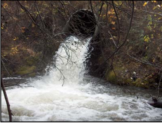
Andimaul Creek: Outlet upstream
