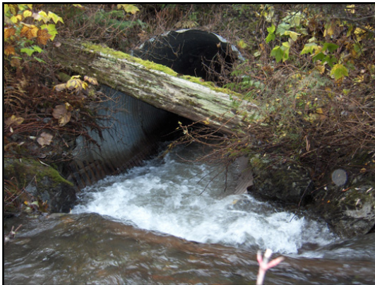
Singlehurst Creek: Inlet downstream
