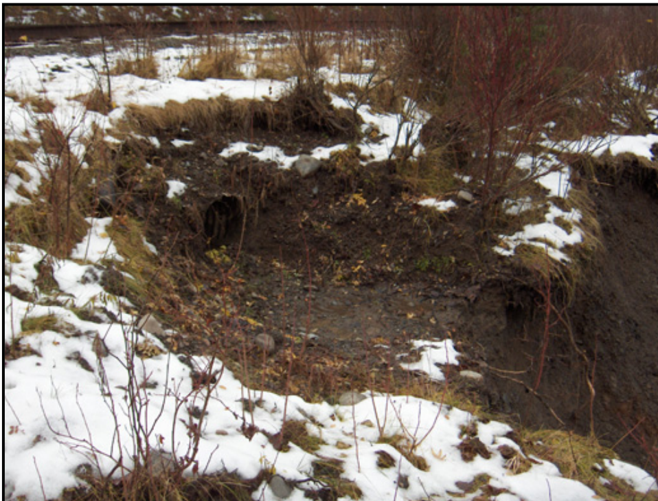
Station Creek slide initiated by ditchline drainage from Highway #16.
