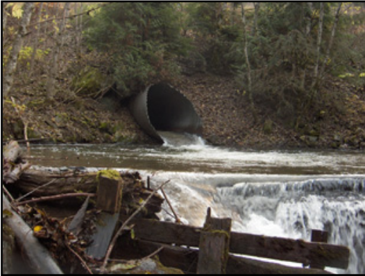
Singlehurst Creek: Outlet upstream
