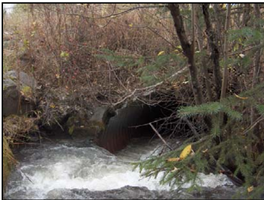
Andimaul Creek: Inlet downstream
