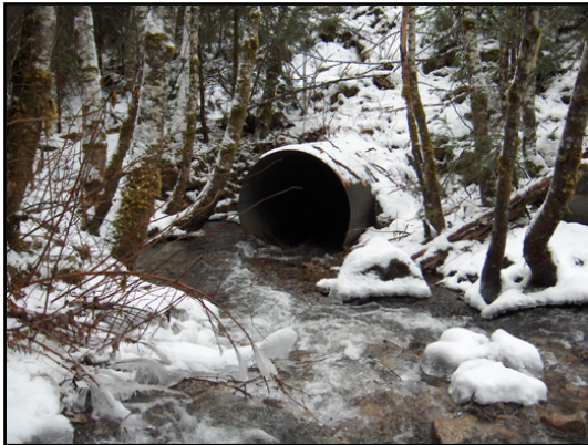
Unnamed Stream # 76: Inlet downstream
