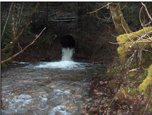
Noble Five Creek: Outlet upstream
