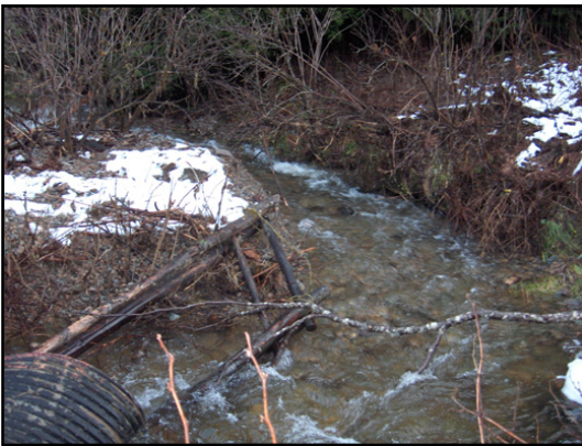
Noble Five Creek: Inlet upstream
