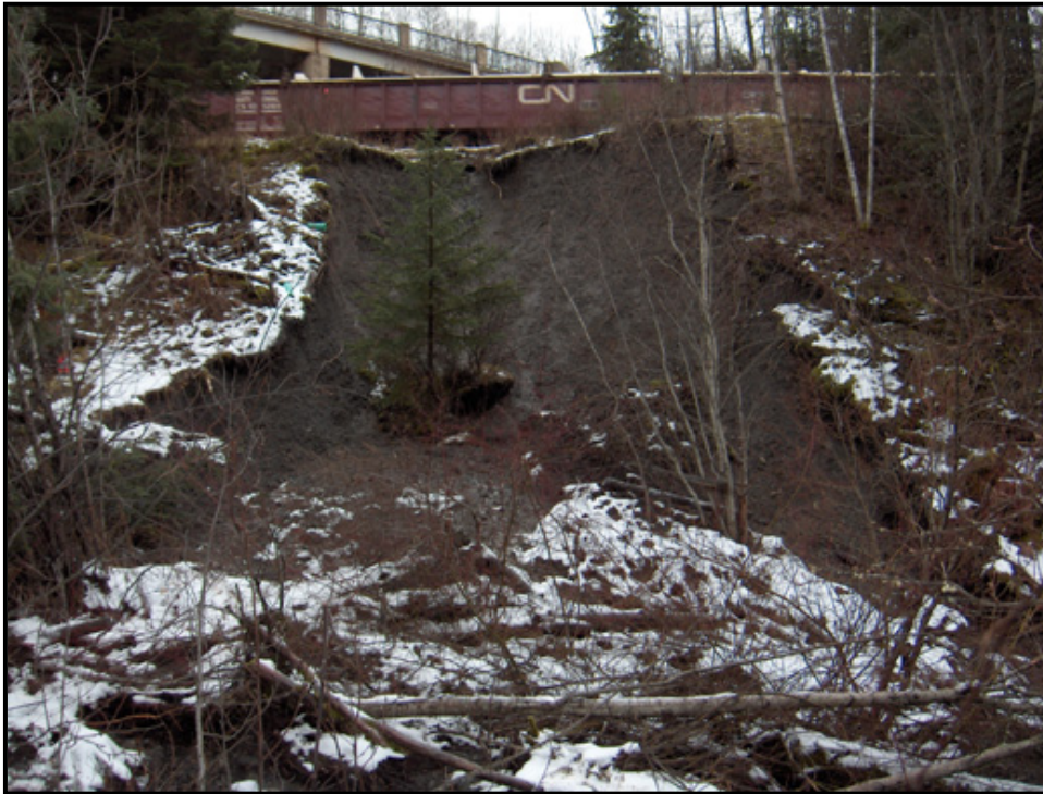
Station Creek: November 22, 2004, view across creek 7 m downstream of outlet.
