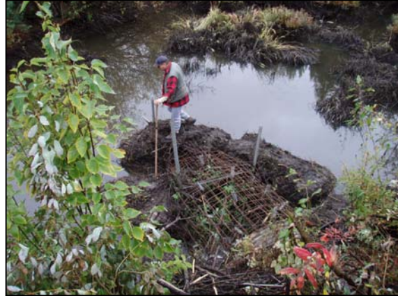
Figure 73. Strawberry Creek culvert inlet.
