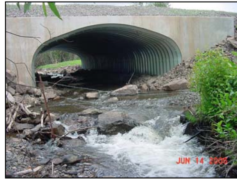
Figures 3 & 4. Thompson Creek – Highway #16 crossing. View on the left shows the Thompson Creek culvert outlets, which were replaced in 2004 with the steel plate arch on the right.
