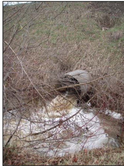
Figure 52. McDowell Creek culvert outlet in high flows. Note hillslope slump above culvert.
