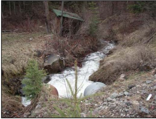
Figure 59. Tyhee Creek culvert outlets. View downstream to outlets in high water, spring, 2007.
