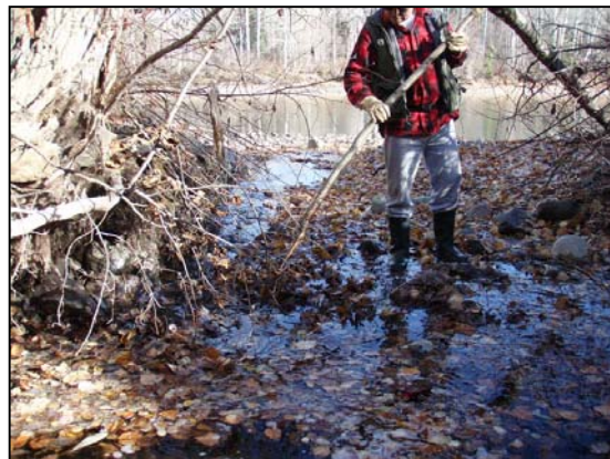
Figure 38. Moan Creek culvert outlet. View downstream from culvert outlet with Bulkley River in the background.
