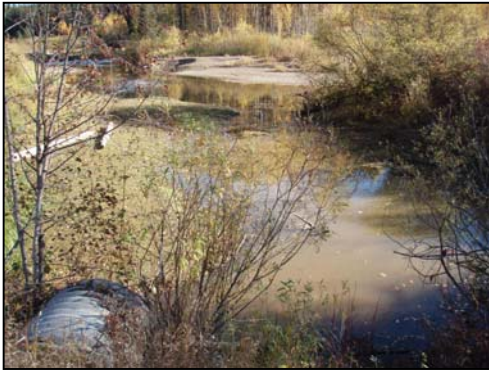
Figure 34. Bulkley Oxbow 1 culvert inlet. View upstream.
