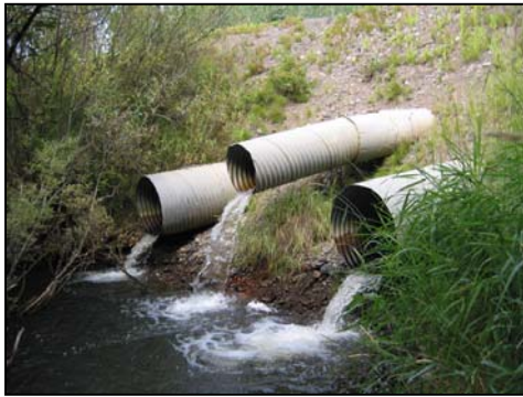
Figures 3 & 4. Thompson Creek – Highway #16 crossing. View on the left shows the Thompson Creek culvert outlets, which were replaced in 2004 with the steel plate arch on the right.
