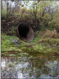
Figure 9: Map Culvert No. 36 Looking downstream from Exchamsiks Backchannel to highways culvert inlet
