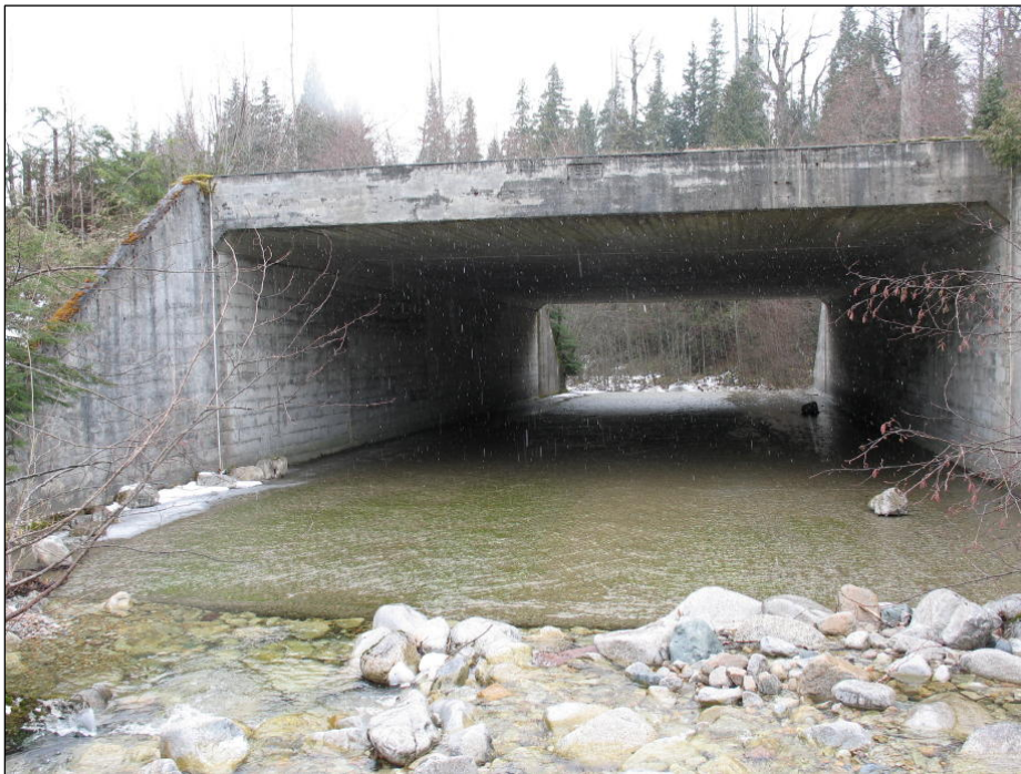
Figure 48: Furlong Creek box culvert, view shows inlet downstream.
