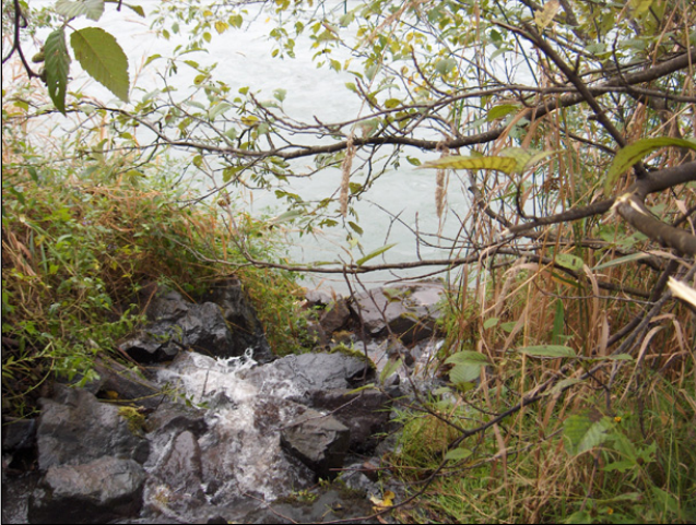
Figure 42: Map Culvert No. 83 View of outlet downstream to Skeena River
