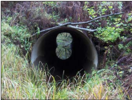
Figure 14: Map Culvert No. 36 CN Rail culvert inlet, view downstream
