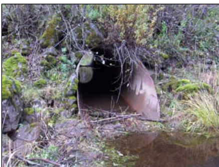
Figure 12: Map Culvert No. 36 View upstream of highways culvert outlet
