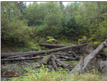
Figure 8: Map Culvert No. 35 Looking downstream from outlet into drainage area between the highway and rail line.
