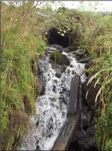
Figure 43: Map Culvert No. 83 View of outlet upstream
