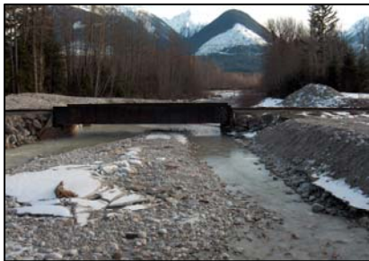
Figure 5: Shames River aggradation sediment accumulated under and upstream of the CN Rail Bridge.
