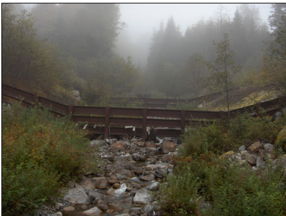
Figure 31: Map Culvert No.61 View upstream from CN bridge shows lower two sediment traps
