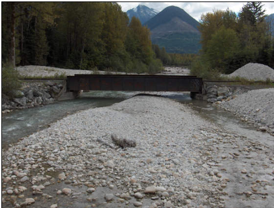
Figure 28: Map Culvert No. 51 Elevated mid channel bar constricting flow under CN Rail Bridge. Sediment spoil dredged from the channel is visible on both banks. View from Highway #16 Bridge
