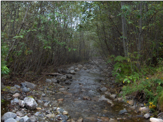
Figure 33: Map Culvert No.61 View downstream of Amsbury Creek from CN Rail's Bridge
