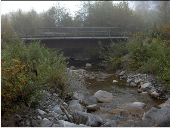
Figure 32: Map Culvert No.61 View downstream to CN Rail's Amsbury Creek Bridge
