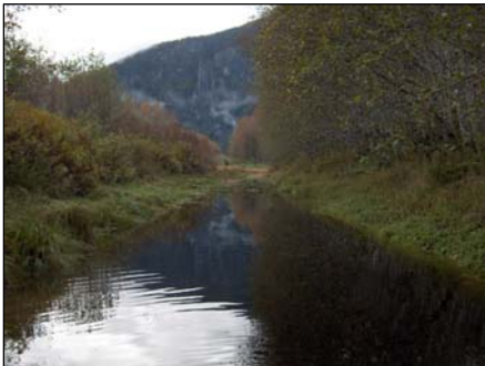
Figure 11: Map Culvert No. 36 View west downstream on Exchamsiks Backchannel
