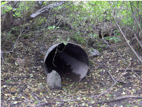
Figure 39: Map Culvert No. 53 View of highway outlet upstream
