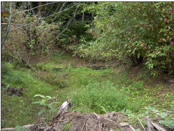
Figure 36: Map Culvert No. 53 Unnamed stream upstream from highway culvert inlet
