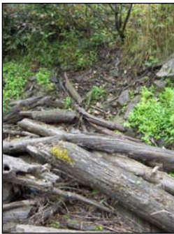
Figure 18: Map Culvert No. 37 View downstream at buried inlet from Backchannel #1
