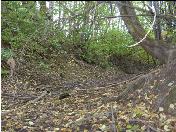
Figure 38: Map Culvert No. 53 View of highway outlet downstream
