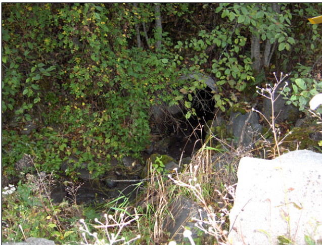
Figure 41: Map Culvert No. 83 View of inlet downstream
