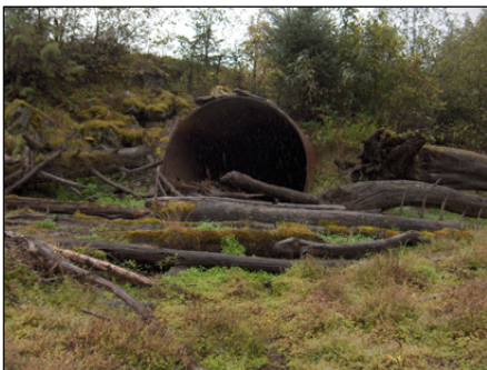
Figure 7: Map Culvert No. 35 Looking downstream from Exchamsiks Backchannel to inlet
