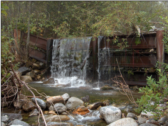
Figure 30: Map Culvert No.61 View shows upper sediment trap
