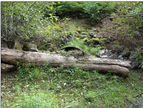
Figure 37: Map Culvert No. 53 View of highway inlet downstream that is largely blocked by LWD and sediment
