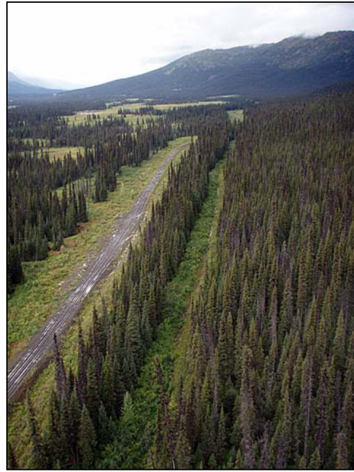
Figure 38. Drainage ditch intercepts soil water movement and converts it to surface flow.
