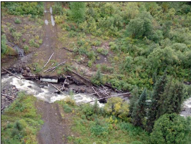
Figure 62. Site 59, view east across Langlois Creek and washed out culvert.
