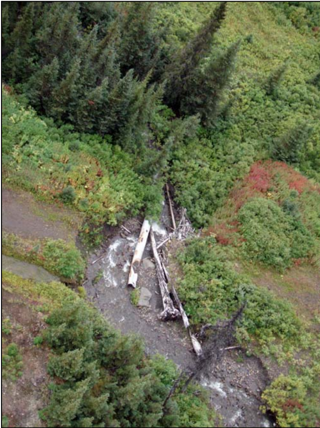
Figure 71. Site 120, washed out culvert on Unnamed Creek.
