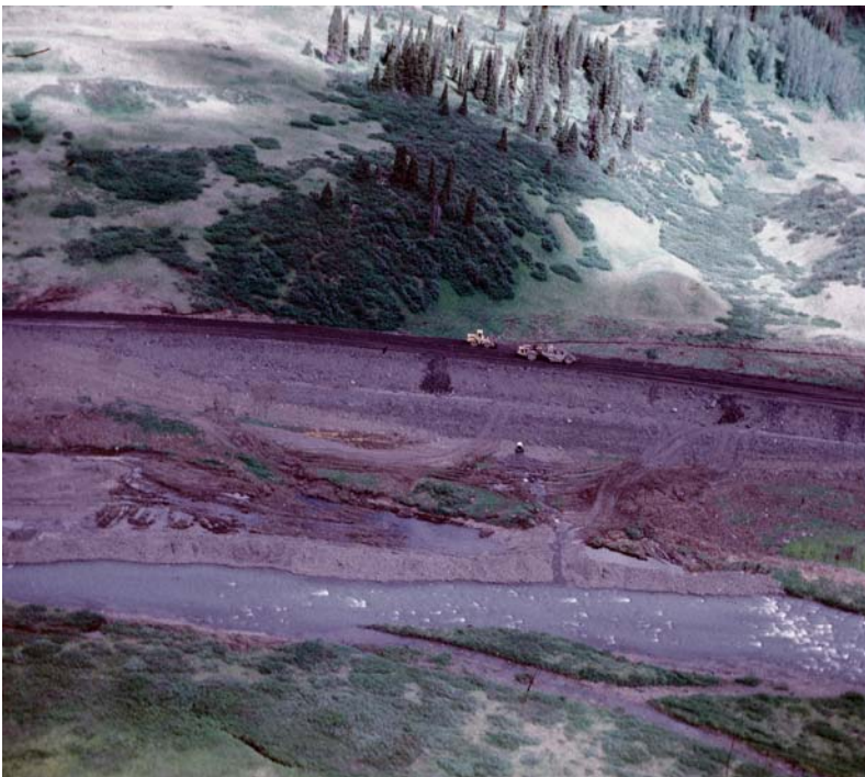
Figure 28. Photo shows Bear River with fill and waste soil encroaching on the channel, 1974.
