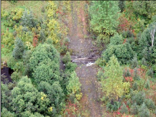
Figure 61. Site 56, Telfer Creek and washed out culvert.
