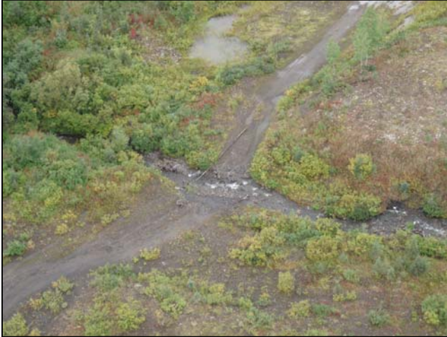
Figure 67. Site 69, view shows washed out culvert.
