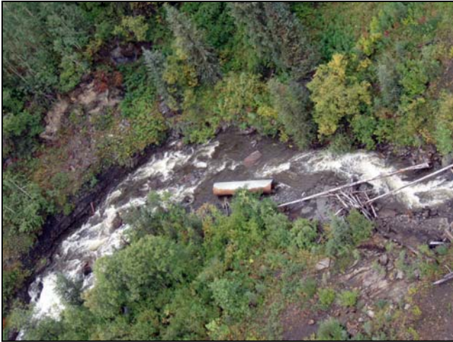
Figure 64. Site 59, view downstream of crossing on Langlois Creek showing section of washed out culvert.
