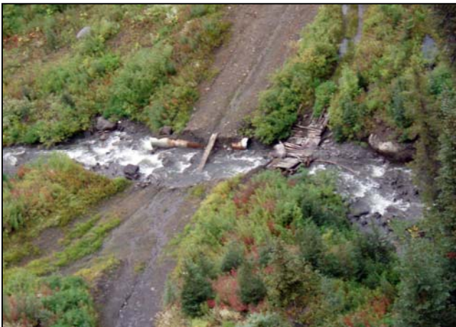
Figure 68. Site 76, view west on Unnamed Creek and washed out culvert.
