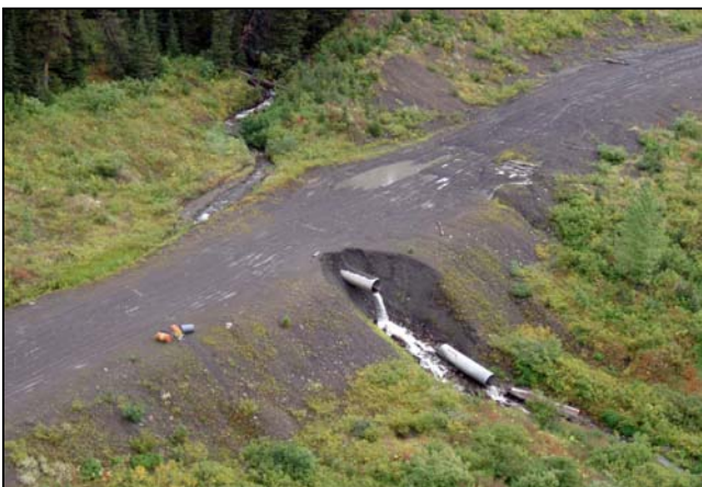
Figure 69. Site 86, Unnamed Creek. View shows washed out culvert outlet.
