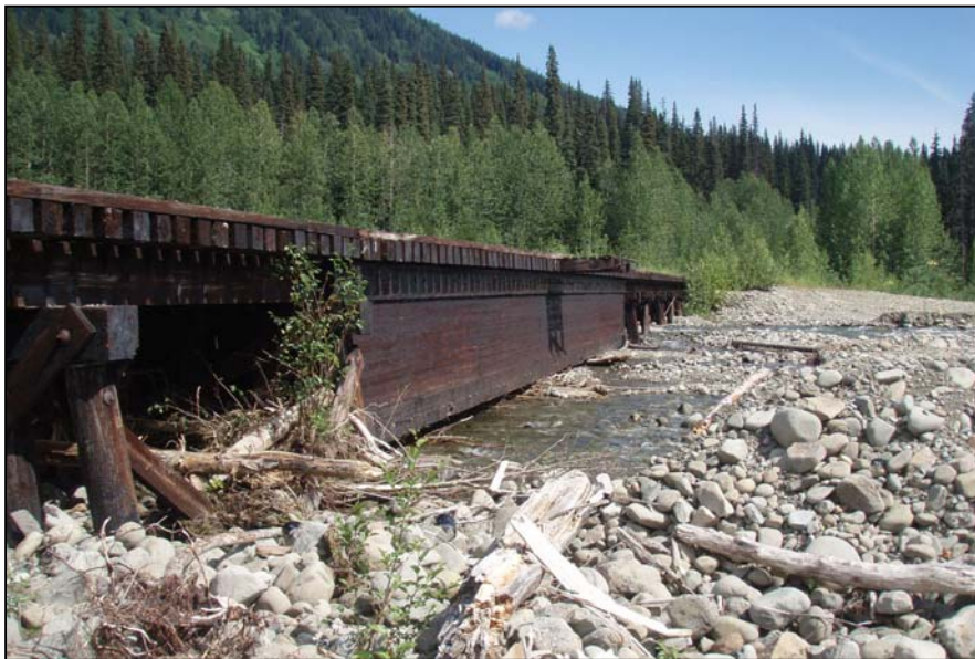
Figure 41. View across downstream side of Azuklotz Creek Bridge showing 10 cm clearance between the bridge span and the stream surface, July 2007.
