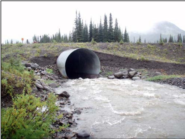
Figure 58. View downstream of the Garner Creek culvert inlet. Note the erosion of the grade fill.
