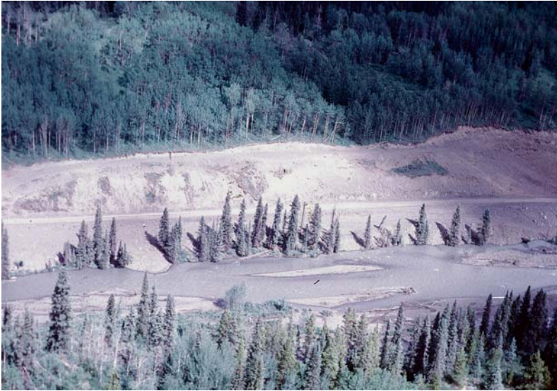
Figure 27. Sediment and waste earth into Bear River, August 1974.
