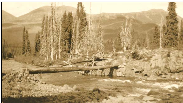
Figure 22. Photo shows log bridge in front of older aboriginal cantilever bridge across Kluatantan River. (Campbell-Johnston 1912)
