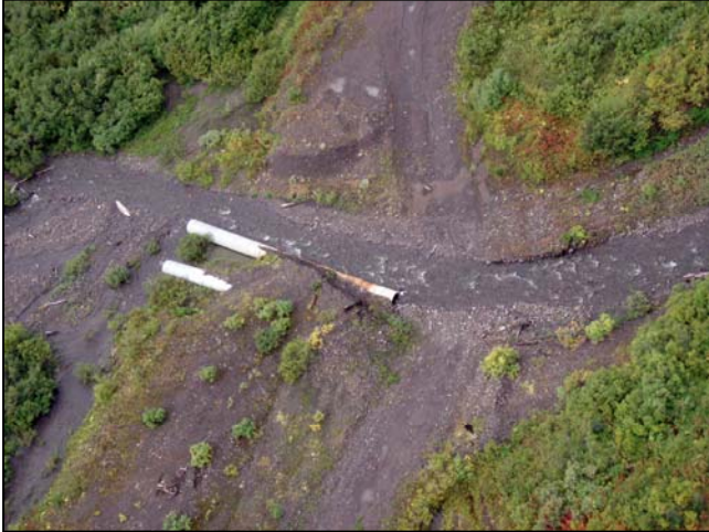
Figure 70. Site 91, view shows washed out culverts.
