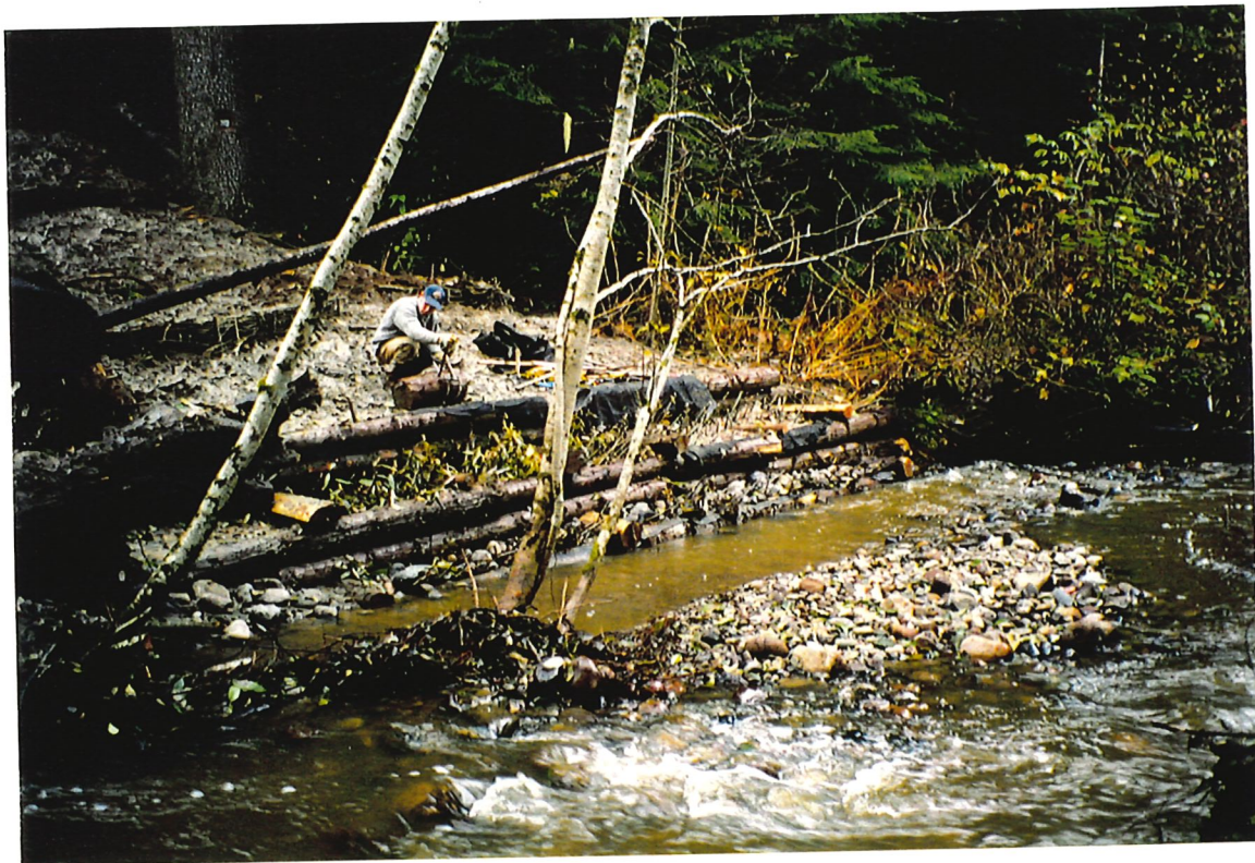
Photo 8: Crib wall structure constructed to stabilize toe of slope.
