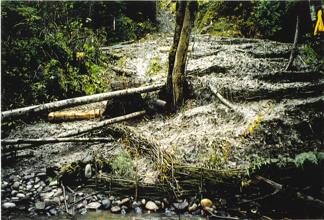
Photo 13: View of slide from right bank showing wattle fencing and bioengineering.
