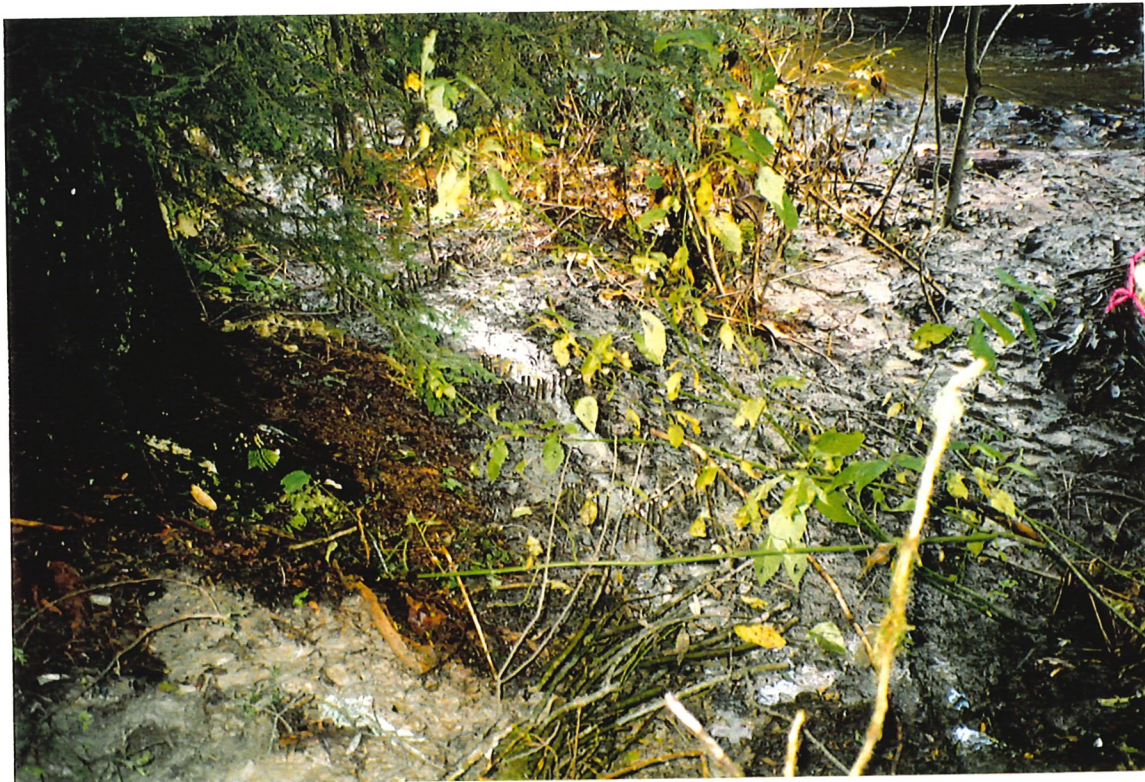
Photo 12: Live pole drain exit with live silt fencing downstream.
