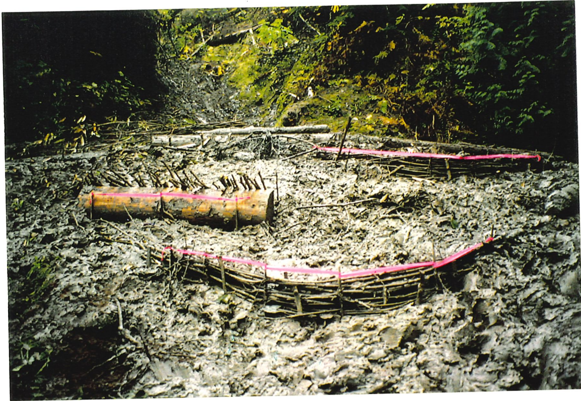
Photo 9: Bioengineering structures: live smiles (bottom and right) and modified brush layer(left).
