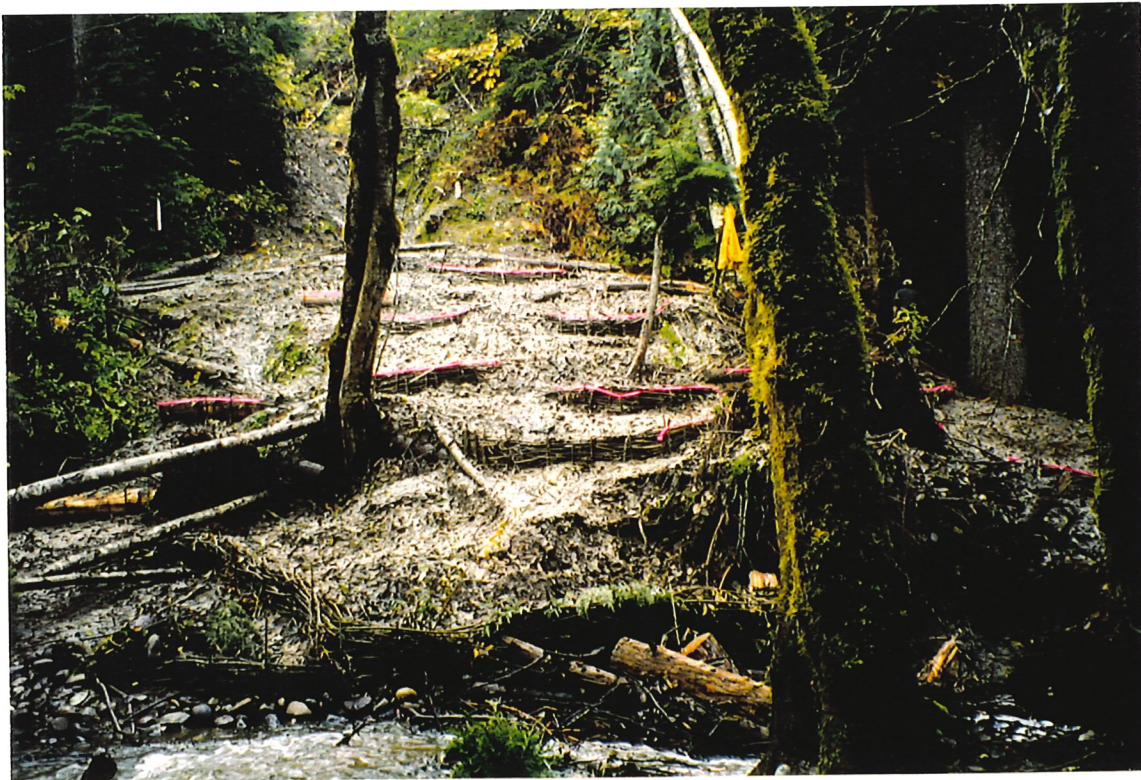
Photo 10: View of depositional zone, showing bioengineering structures.
