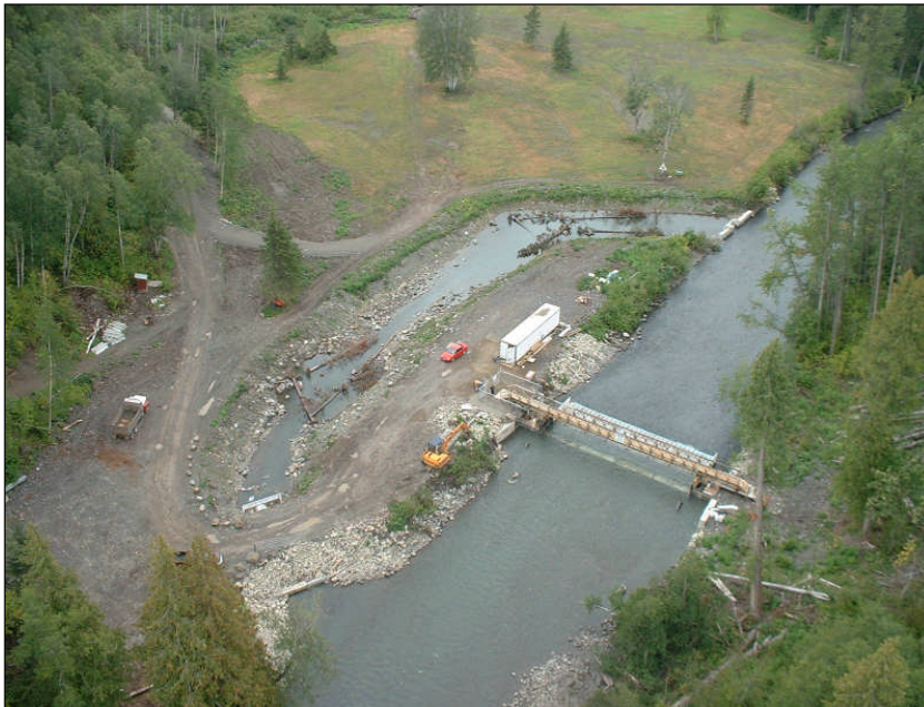
Kitwanga River Salmonid Enumeration Facility, 2003.
