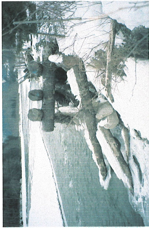
Photo 13. Looking upstream at the backside of Debris Catcher 2. The structure has remained stable with minor shifting.
