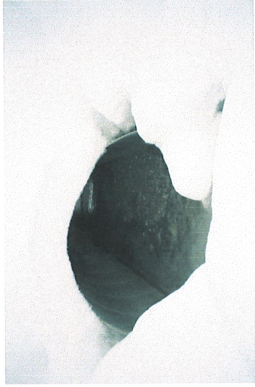
Photo 3. Looking at the culvert inlet at Site 77. Gravels have infilled the bottom of the culvert for 6m.
