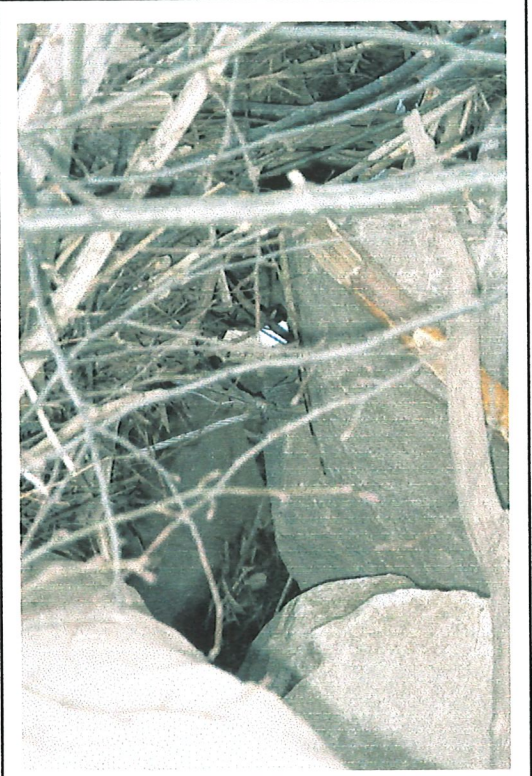
Photo 11. Looking underneath Debris Catcher 1 at a frayed cable attached to a boulder that required re-attachment.
