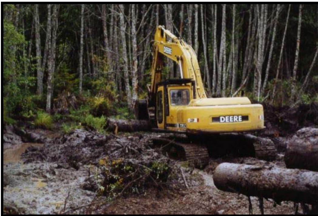
Figure 4. Excavation of the lower pond.
