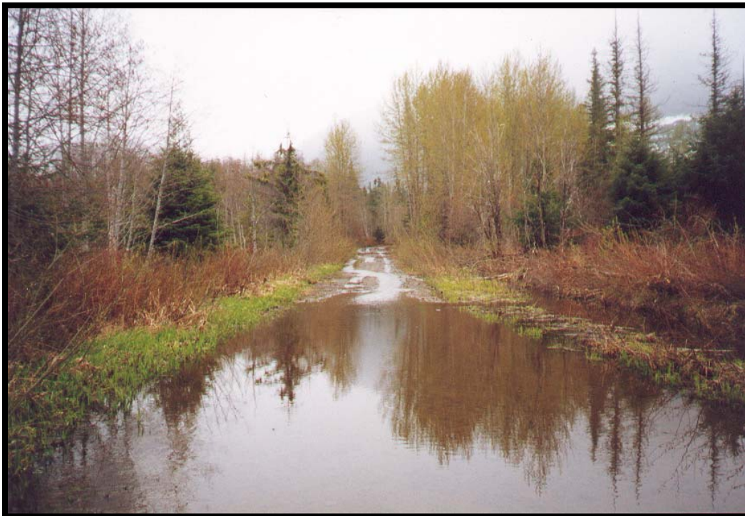
Figure 1. Killutsal Creek flows flooding White Creek Road.
