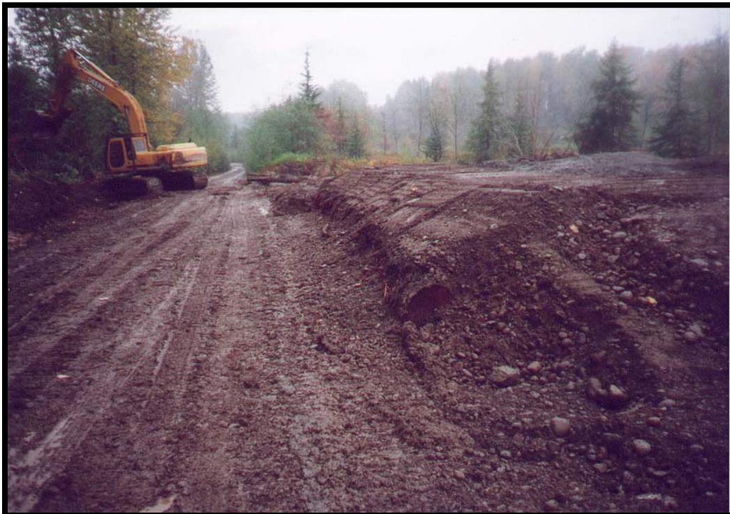
Figure 6. Berm construction parallel to White Creek Road.
