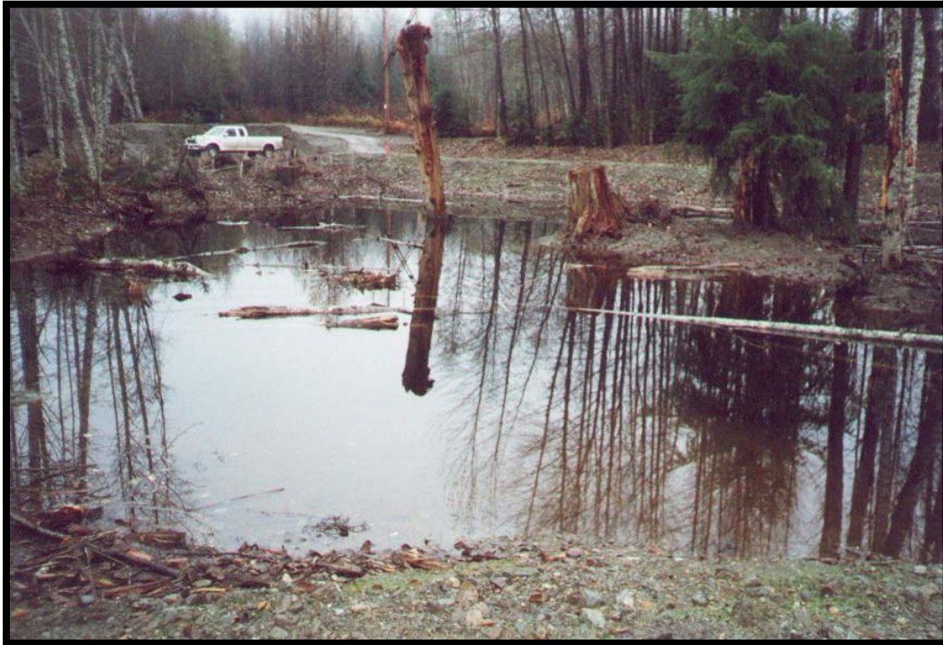
Figure 5. Lower rearing pond after construction. Note LWD.
