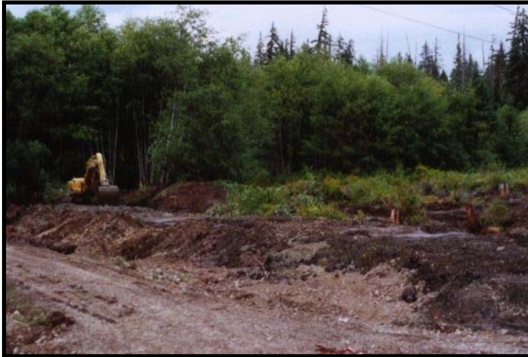
Figure 7. Upper pond construction adjacent to the road.
