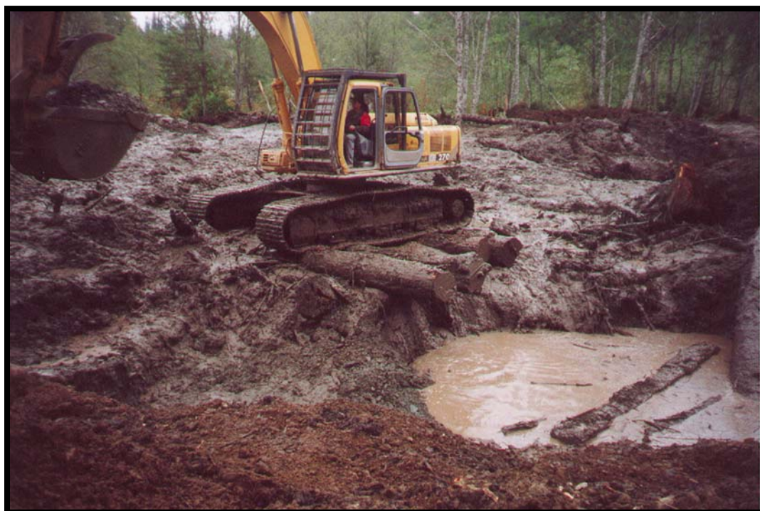
Figure 3. Corduroy road used during the pond construction.
