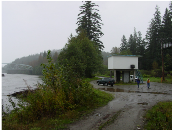
Photo 7: Kitimat River with pump house #7
