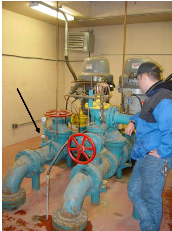
Photo 9: Sampling tap inside pump house #7
