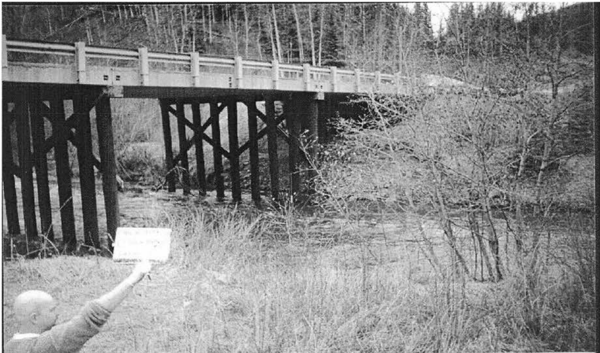
Plate 2: Trap site at Buck Flats bridge #1 looking approximately upstream.
