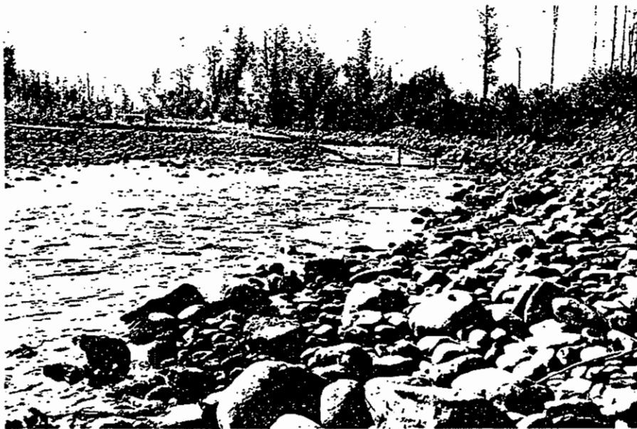
Figure 3.11 SC2 is a large active side channel of the Telkwa River. This substrate, with large interstitial spaces provides excellent cover for juvenile fish.
