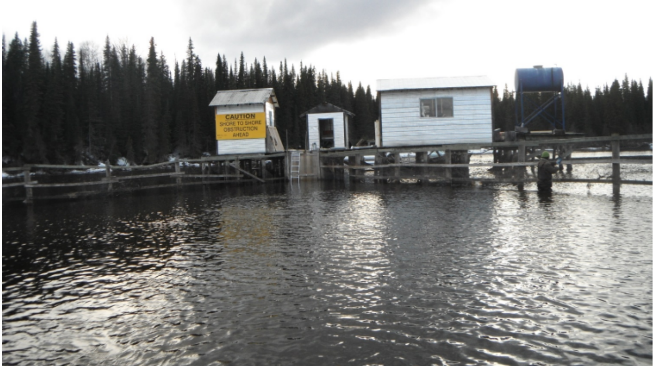
Figure 5. Front view of the Babine smolt enumeration facility, with the wire mesh leads, and the entrance to the smolt trap in the middle of the two leads.
